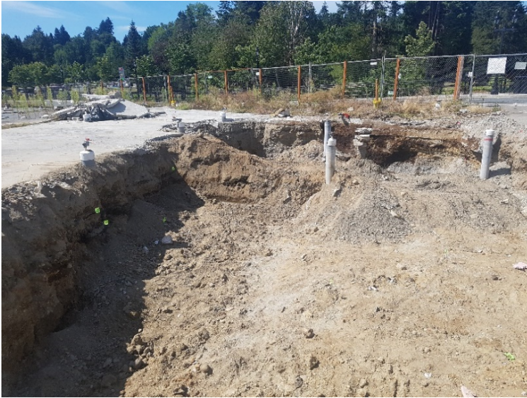
Excavation; monitoring wells intact
