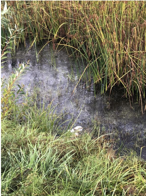
Location 1. Standing Water in West Bioswale
