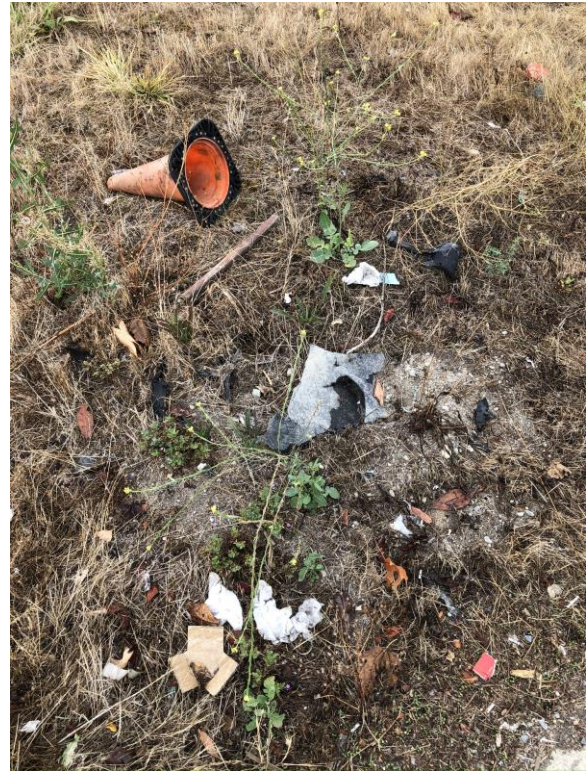
Location 9. Exposed Geomembrane
