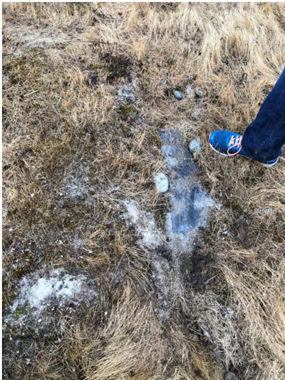
Location 4. Exposed Geomembrane
