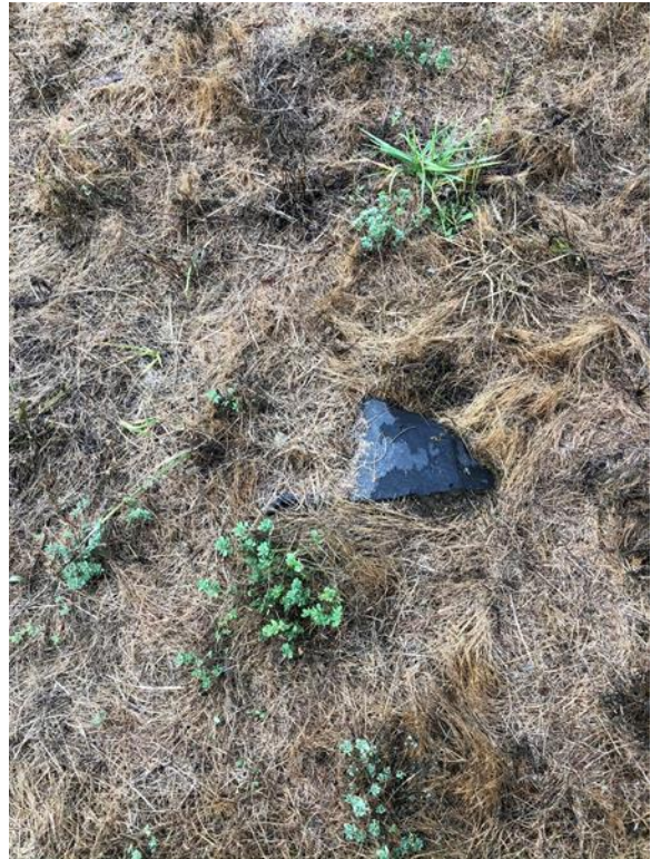
Location 5. Exposed Geomembrane
