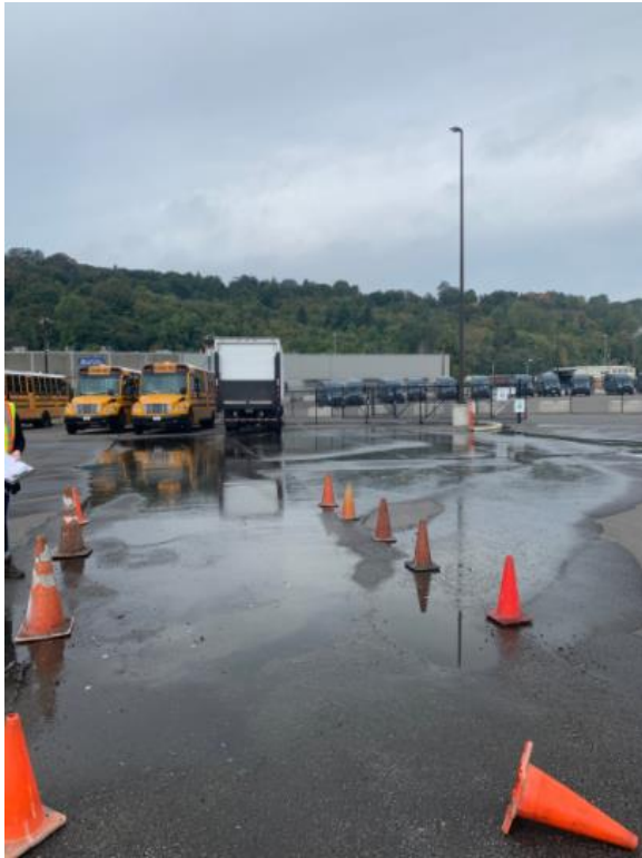
Location 20. Water Flowing from Asphalt
