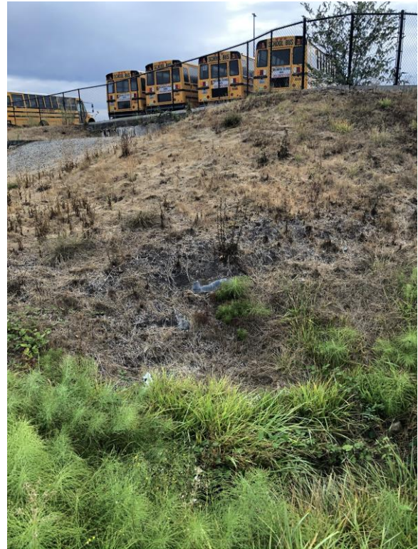
Location 7. Exposed Geomembrane
