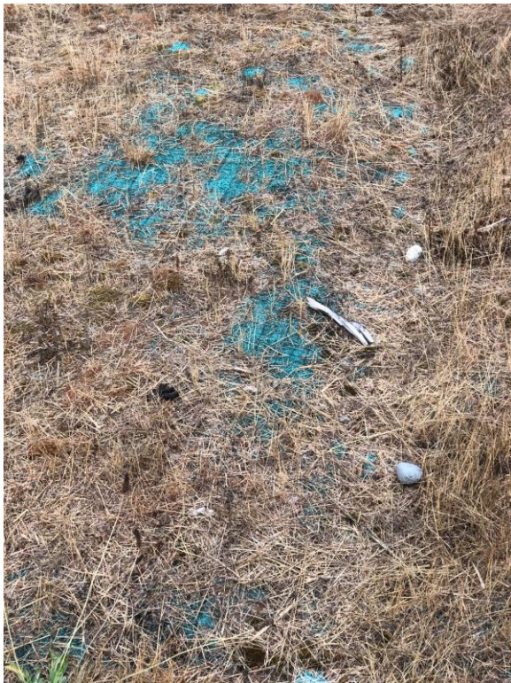
Location 2. Exposed Geotextile
