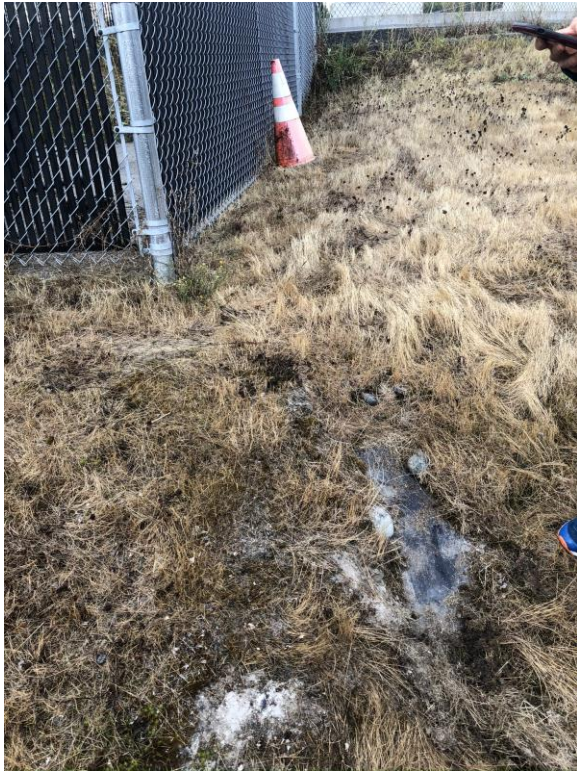
Location 4. Exposed Geomembrane
