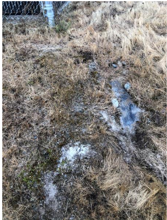
Location 4. Exposed Geomembrane
