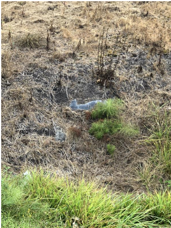
Location 7. Exposed Geomembrane
