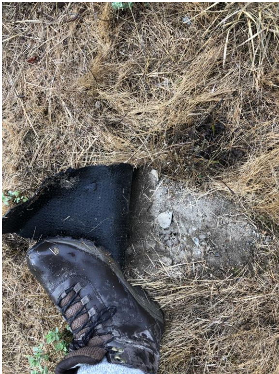
Location 5. Exposed Geomembrane
