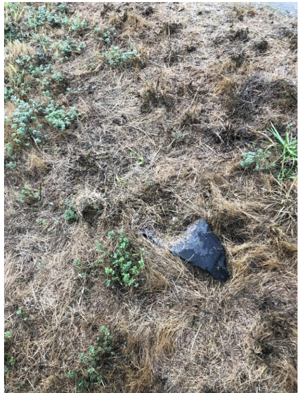
Location 5. Exposed Geomembrane
