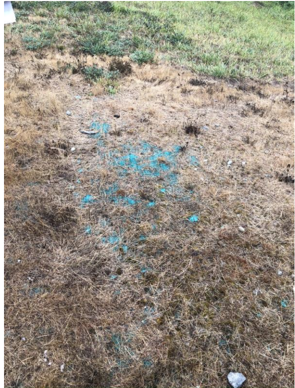
Location 3. Exposed Geotextile
