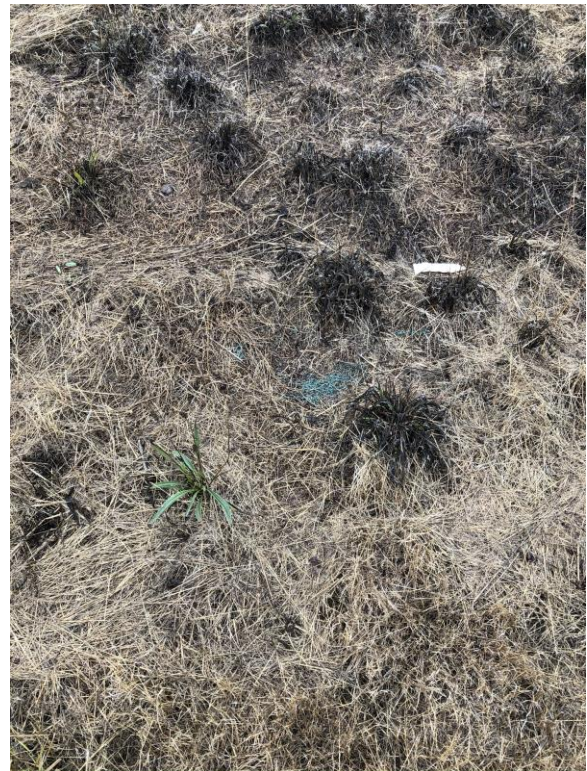
Location 11. Exposed Geotextile
