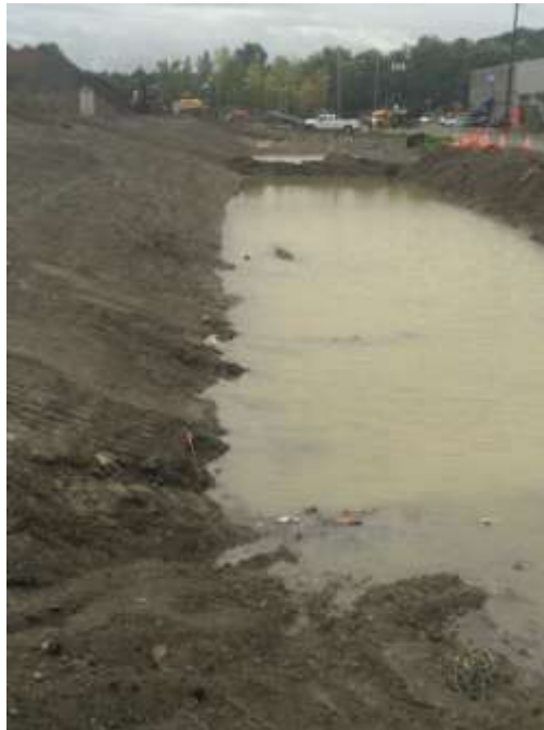
Photo 8: Water in newly formed West Ditch above solidification soil
