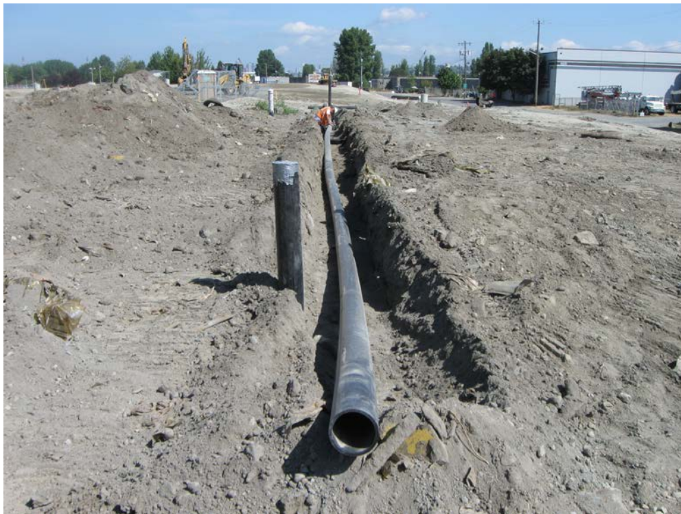
Photograph 26: Installation of gas connector pipe, looking north.
