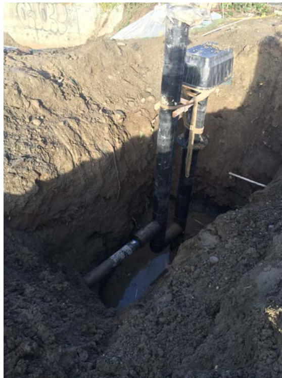
Photograph 24: North sump following installation.
