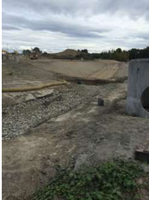
Photo 7: New West Ditch formed atop solidified soil
