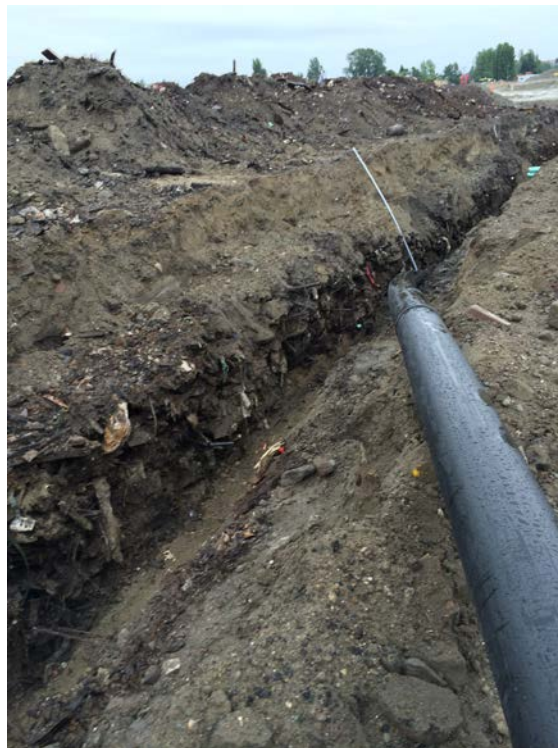
Photograph 22: Placement of landfill gas main, looking northwest.
