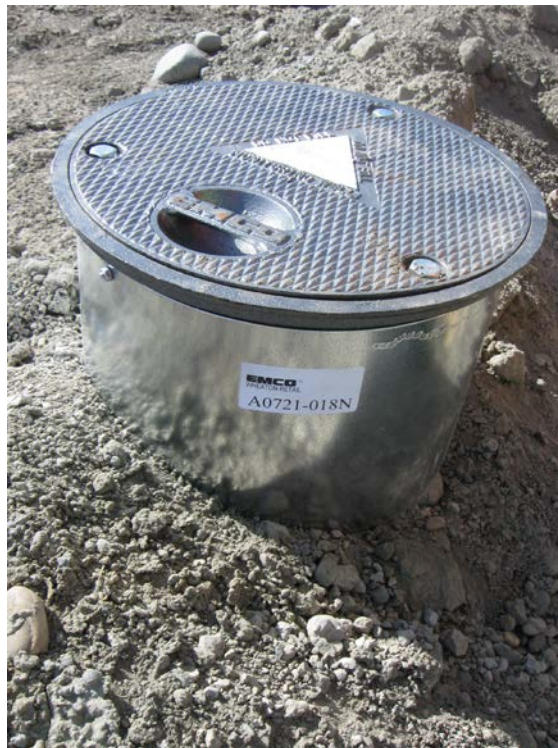
Photograph 34: Eighteen-inch monument and well head cover following installation.
