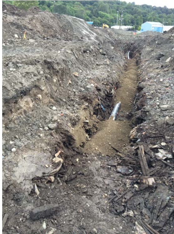
Photograph 23: Placement and backfill of gas main piping, looking northwest.
