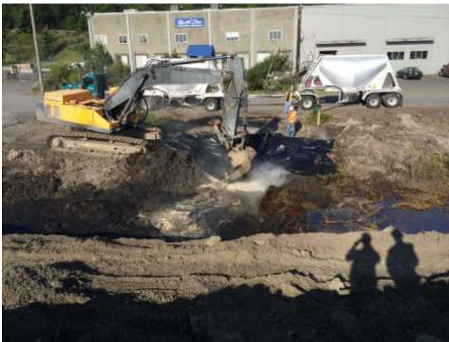
Photo 6: Dust control during West Ditch soil solidification
