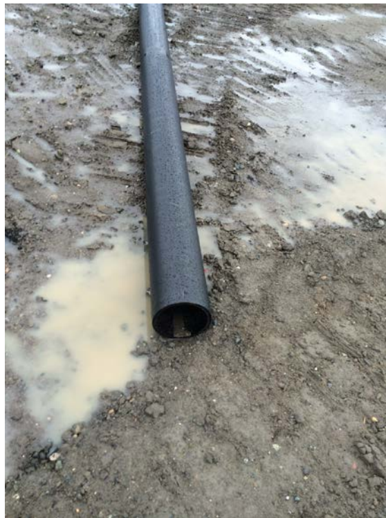
Photograph 16: Eight-inch landfill gas main piping prior to installation.
