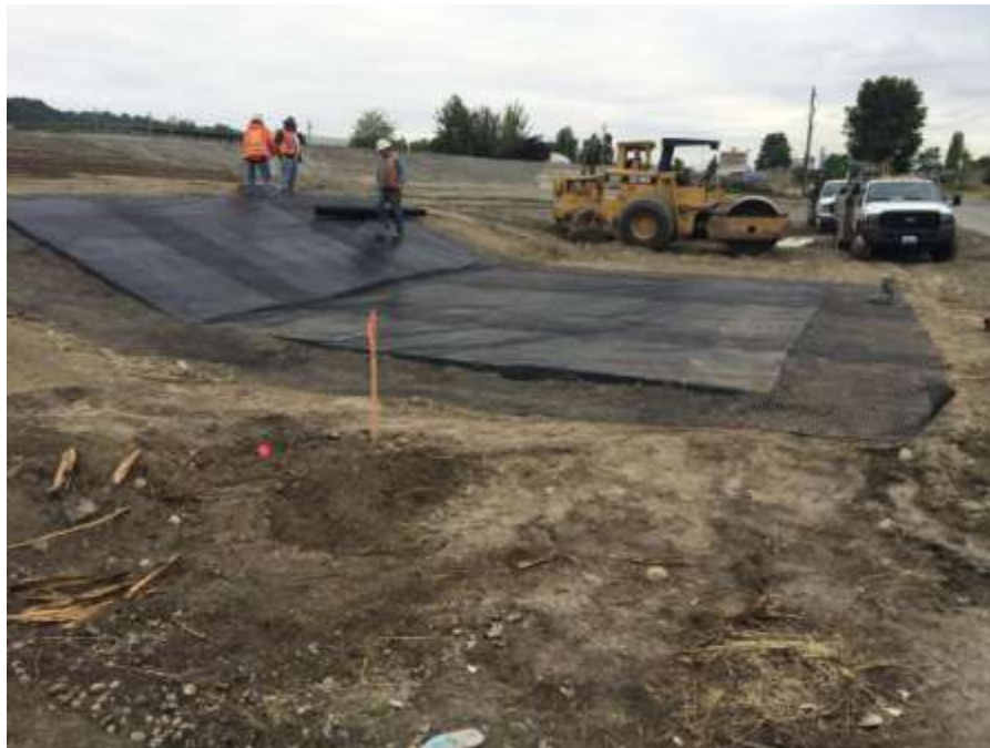
Photo 8: Geogrid reinforcement and chemically resistant liner atop Geofoam backfill
