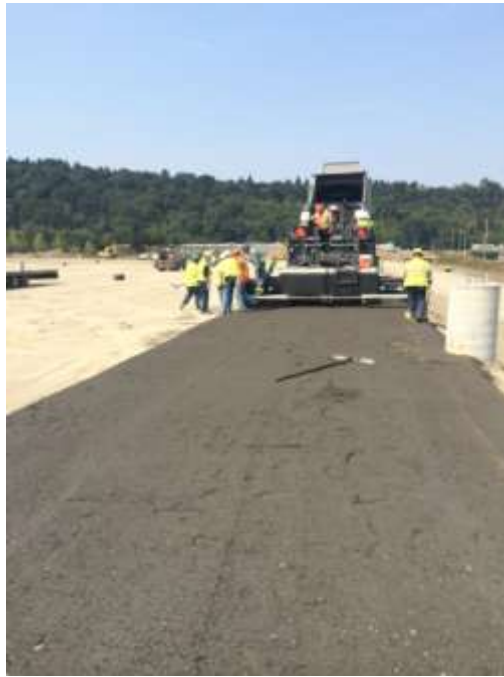
Photo 11: Beginning crushed rock installation
