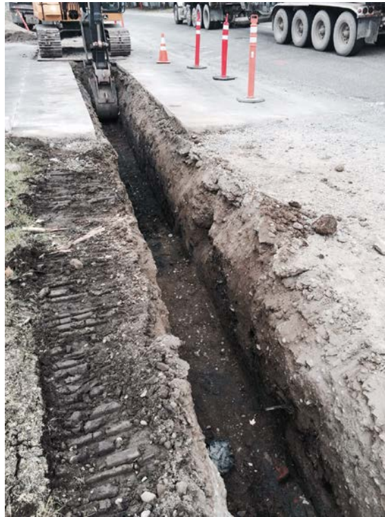
Photograph 13: Excavation for gas collection trench No. 5, looking north.
