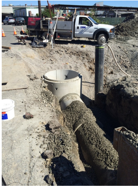
Photograph 1: Manhole MH-R4, looking north.
