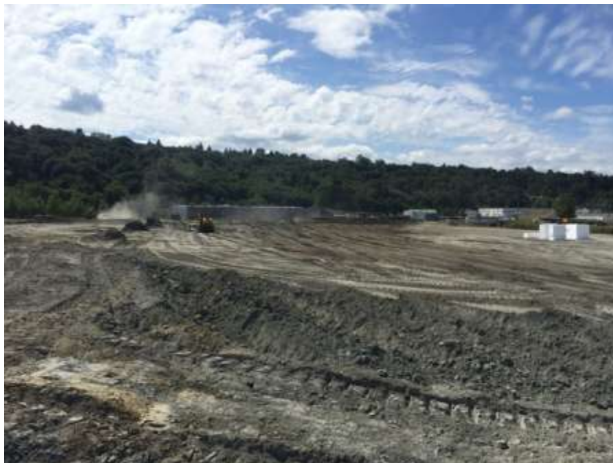
Photo 2: Backfilling operations atop landfill
