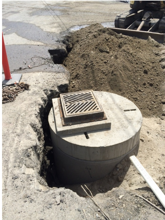
Photograph 3: Catch basin CB-27, looking south.
