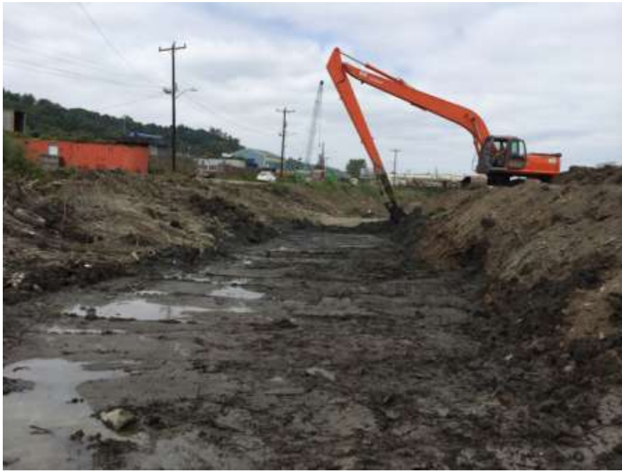
Photo 3: West Ditch soil solidification proceeding south to north
