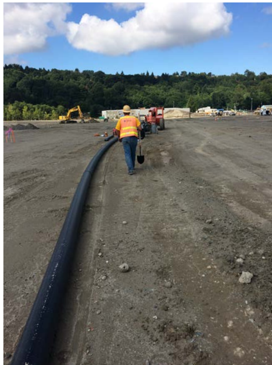
Photograph 18: Landfill gas main piping prior to installation, looking west.
