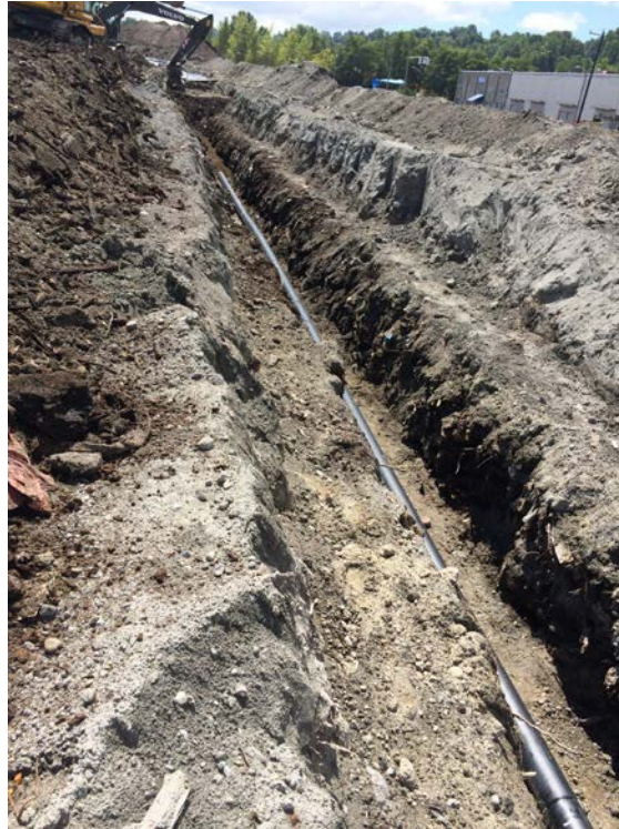
Photograph 21: Landfill gas main installation, looking south.
