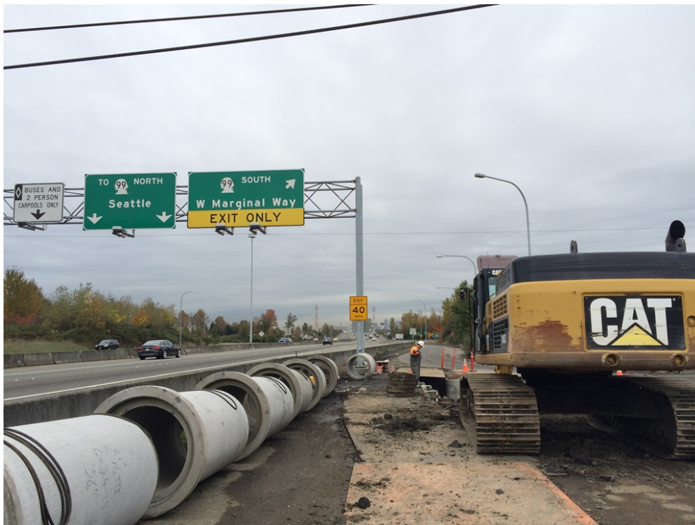
Photograph 2: Manhole SDMH-1, looking north.
