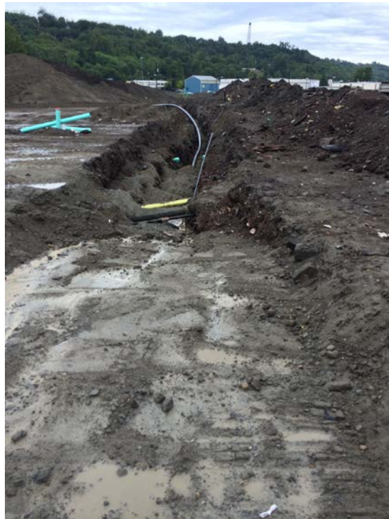
Photograph 20: Landfill gas main installation, looking northwest.
