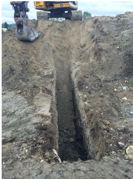
Photograph 10: Trenching through trash for installation of gas collection trench, looking south.
