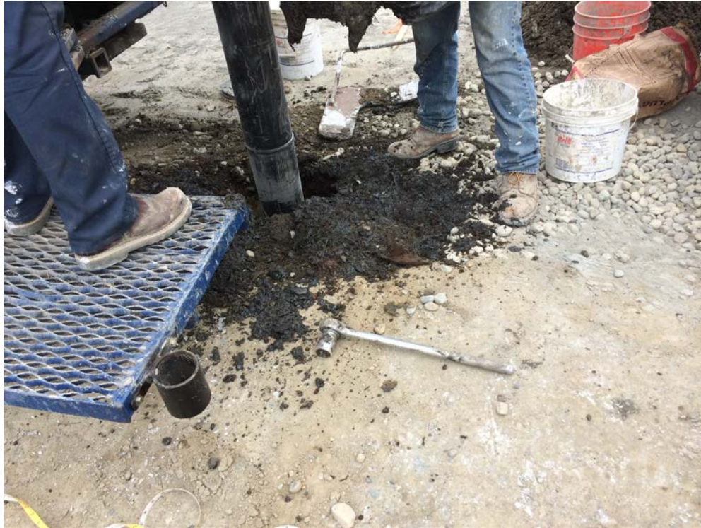
Photograph 7: Placement of gas collection well.
