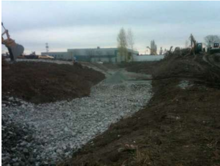
Photo 1: Quarry spalls at bottom of east-west bisecting ditch (former East-West Channel)
