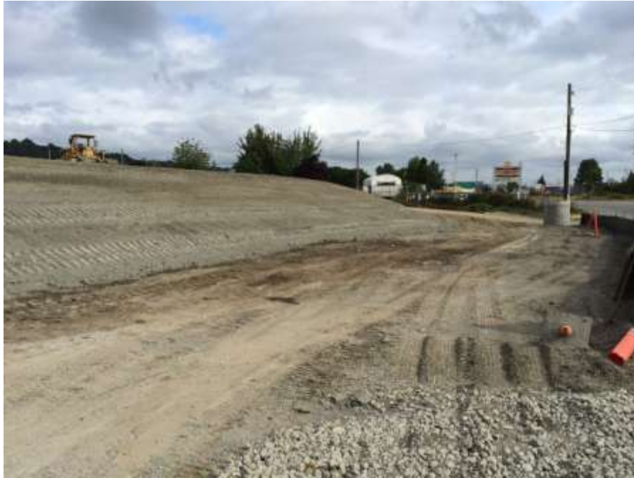
Photo 3: Grade raised approximately 12 feet in northeast corner of SPPD Property
