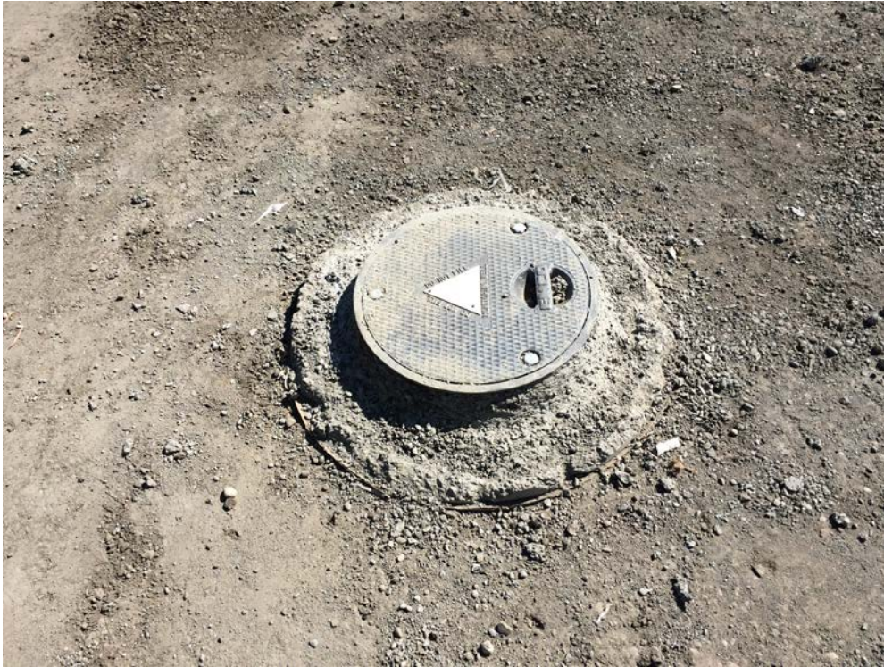
Photograph 35: Well head monument and cover following concrete placement.
