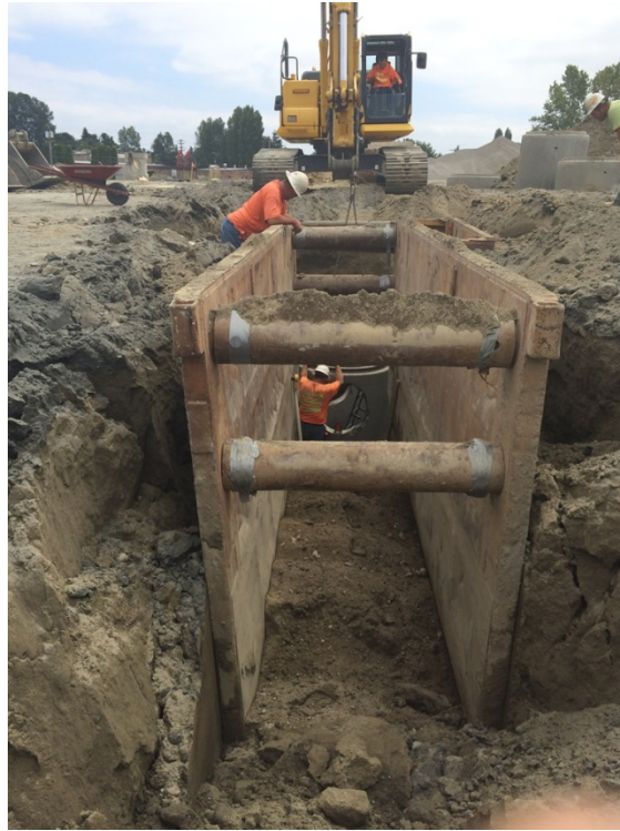
Photograph 5: Setting on-Site structures.
