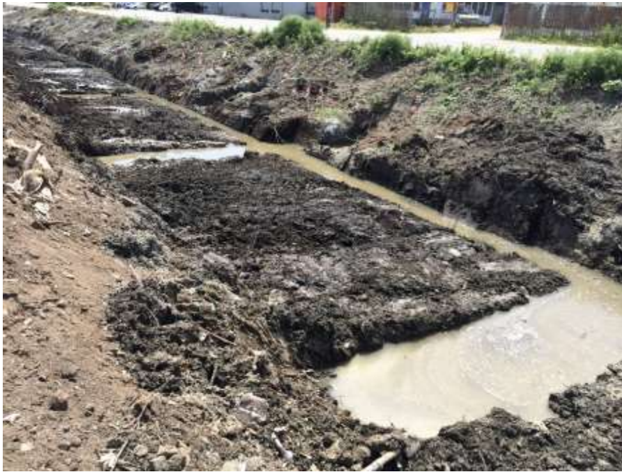
Photo 5: West Ditch soil solidification cross ditches to allow ground water cross flow
