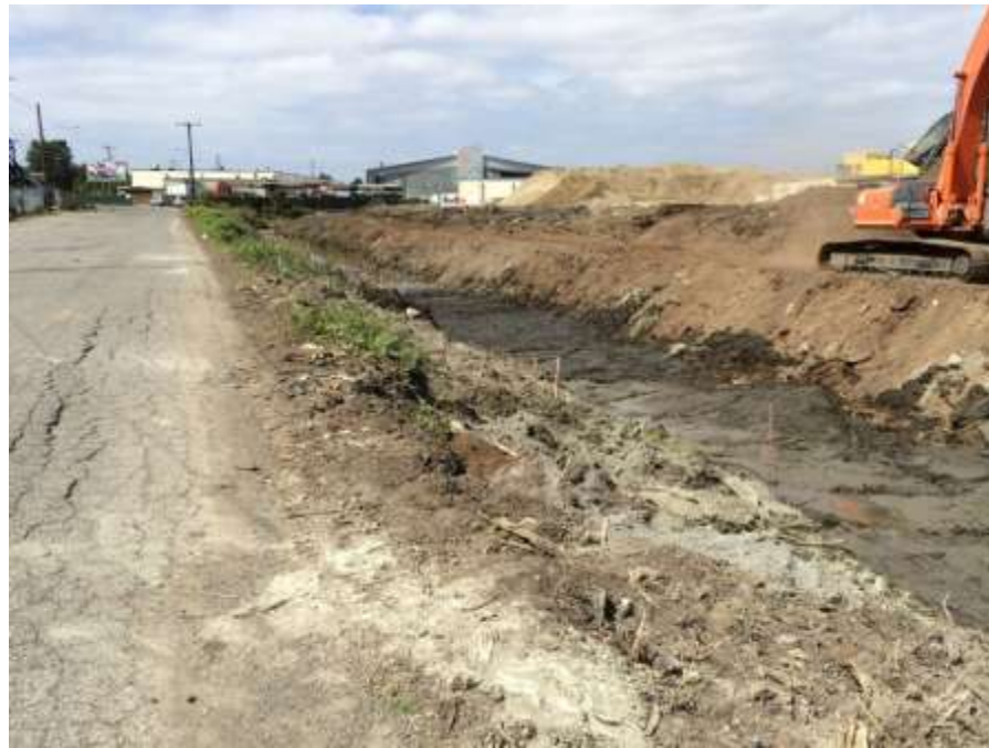
Photo 4: West Ditch soil solidification near midpoint
