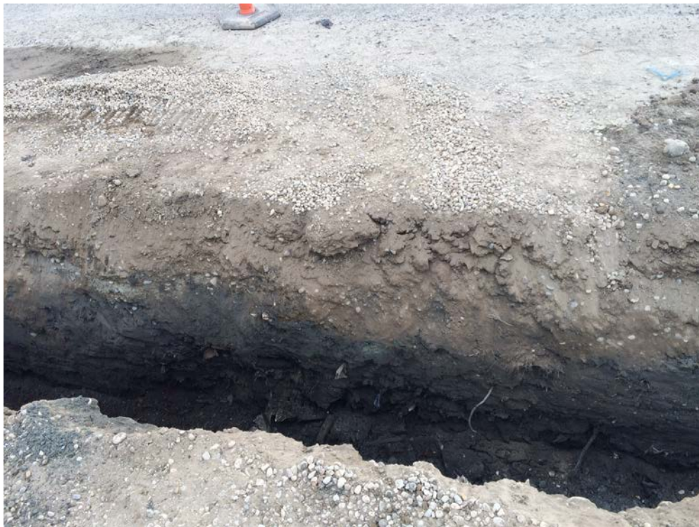
Photograph 12: Excavation for gas collection trench No. 2, looking east.
