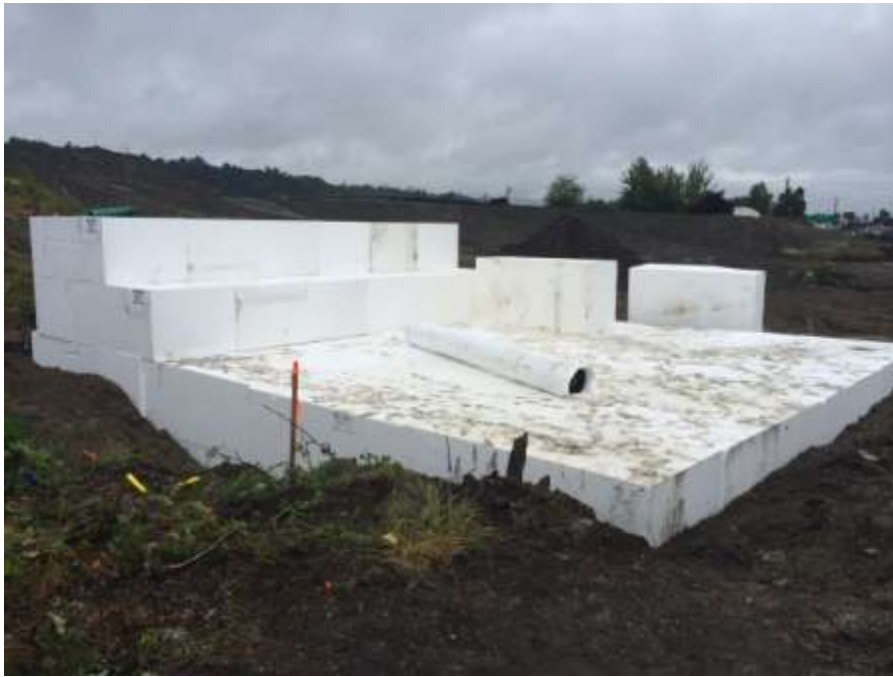
Photo 7: Geofoam backfill at east end of bisecting ditch (Former East-West Channel)
