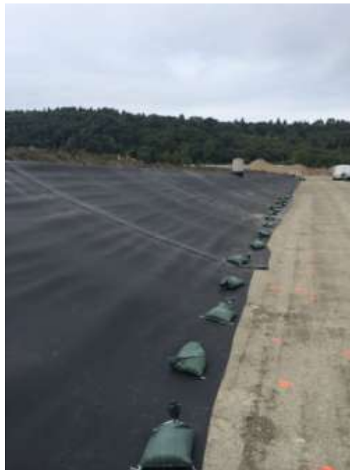
Photo 14: Low-permeability liner installation on north slope above north access road
