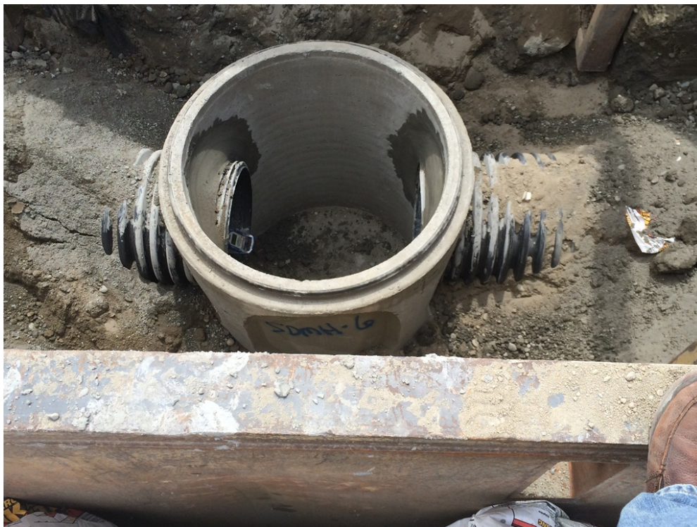
Photograph 4: Manhole SDMH-6 installation.
