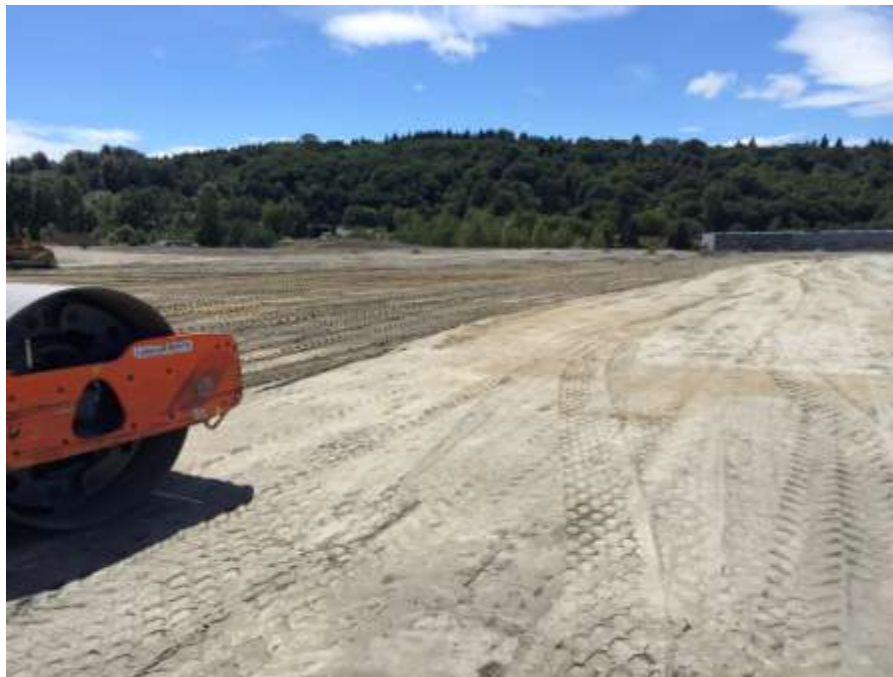
Photo 6: Finish grading and compaction atop landfill
