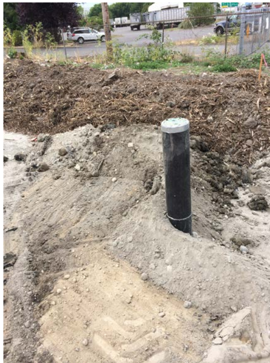
Photograph 8: Vertical collection well following installation, looking northwest.
