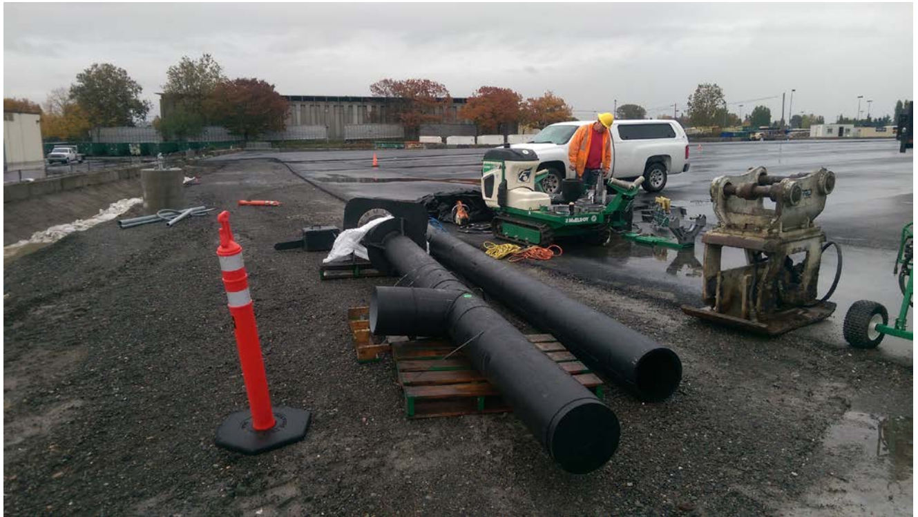
Photograph 19: North sump prior to installation.
