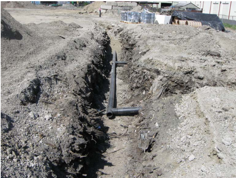
Photograph 30: Gas connector pipe installation and backfill placement, looking west.
