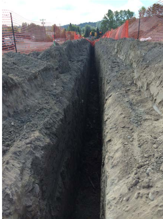
Photograph 11: Excavation for gas collection trench No. 1, looking south.
