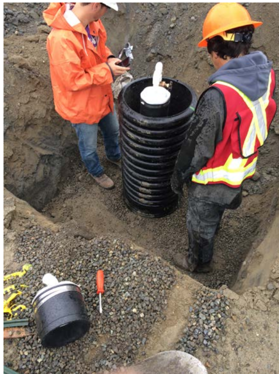
Photograph 32: Assembling gas collection well head.
