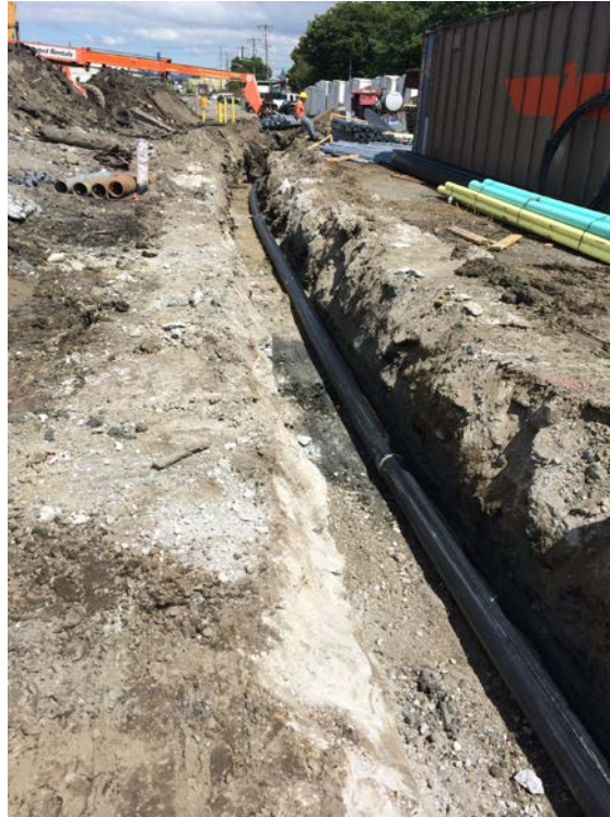
Photograph 17: Landfill gas main trench prior to placement of backfill, looking north.
