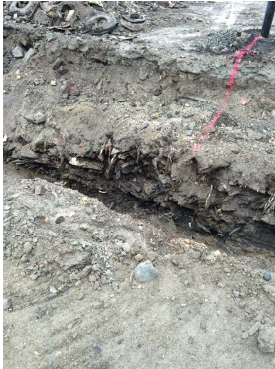
Photograph 25: Trenching for gas connector pipe.
