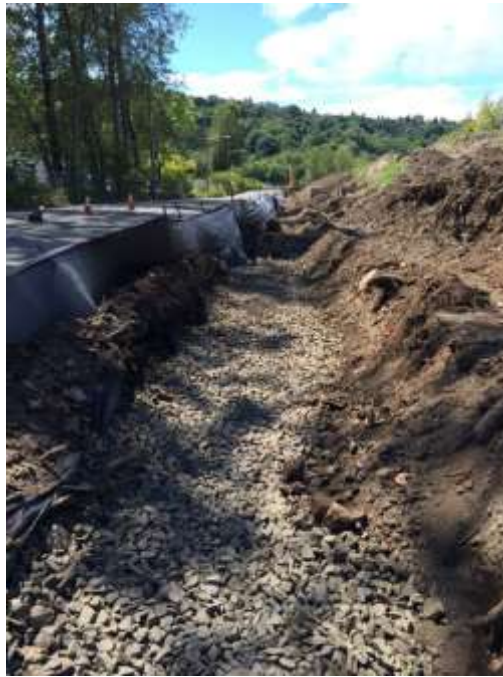
Photo 9: Subgrade improvement for gabion wall along south perimeter of SPPD Property
