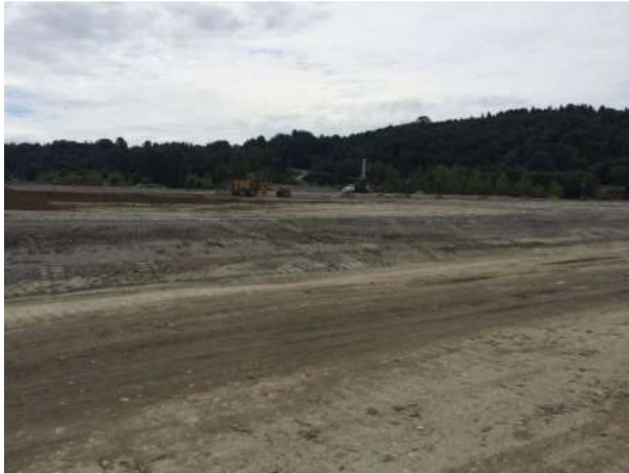
Photo 5: Finish grading atop landfill. North access road in foreground
