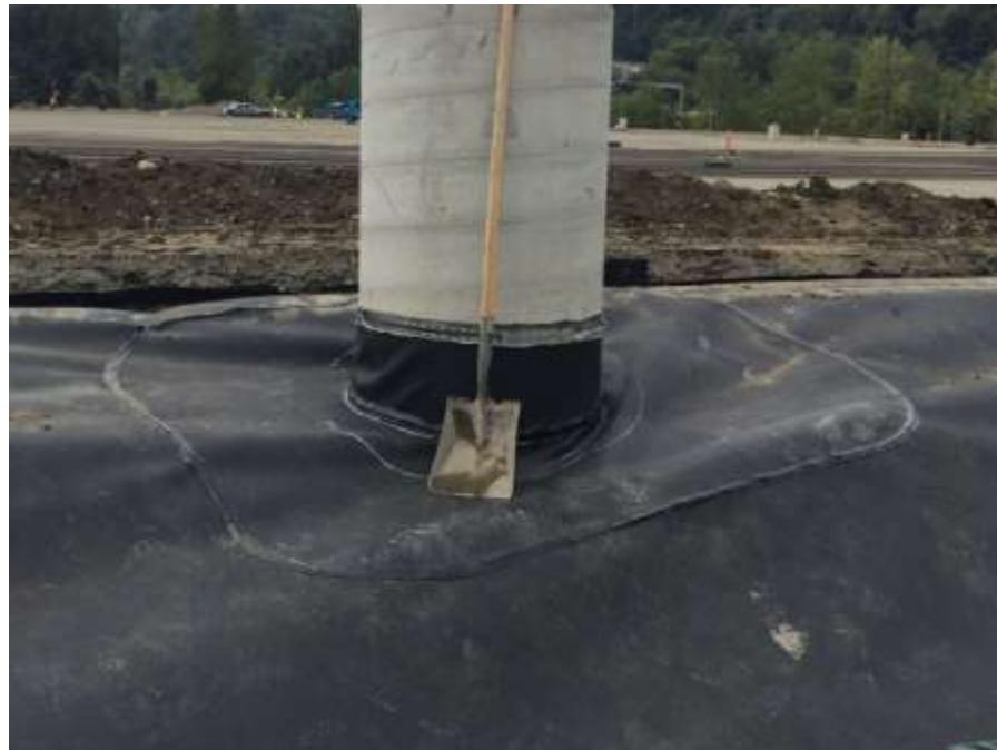
Photo 15: Low- permeability liner anchorage at top of slope
