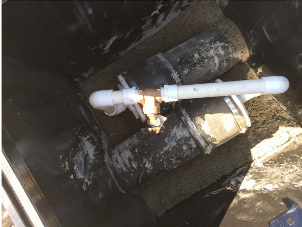
Photograph 31: Top of slope trench connector control assembly.
