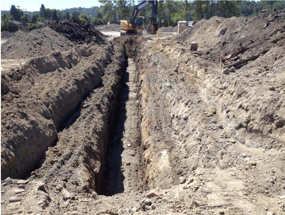
Photograph 15: Gas collection trench following backfill with gravel, looking south.
