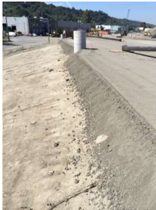
Photo 12: Full thickness (12 inches) of crushed rock atop landfill
