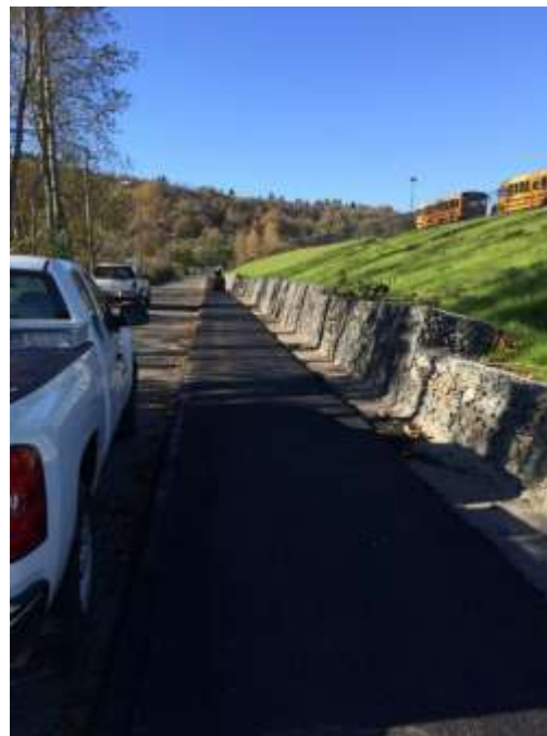
Photo 10: Completed gabion wall, backfill, asphalt walkway and hydro-seeded
