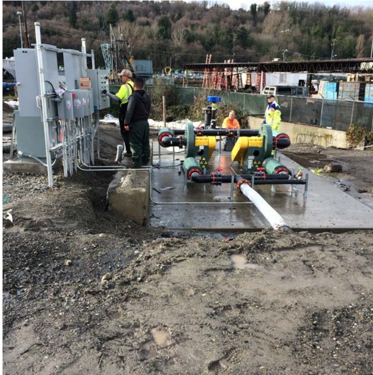
Photograph 1: North treatment compound.
