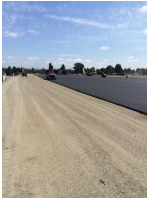
Photo 13: First 2- inch-thick lift of asphalt concrete cover cap
