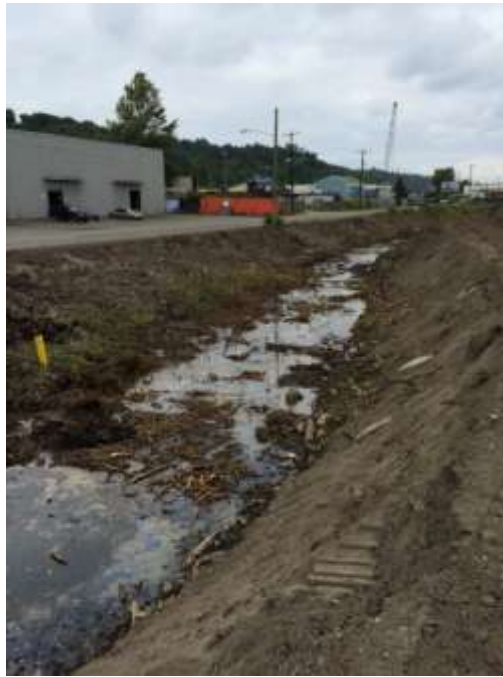
Photo 1: West Ditch after clearing and grubbing and prior to soil solidification
