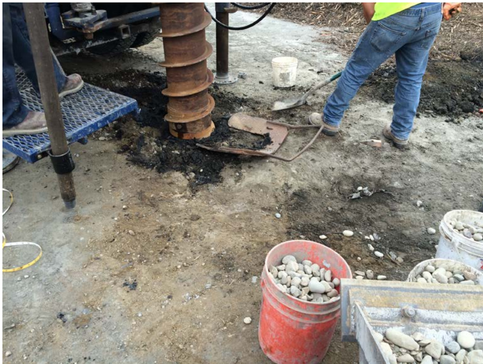
Photograph 6: Drilling for gas collection well installation.
