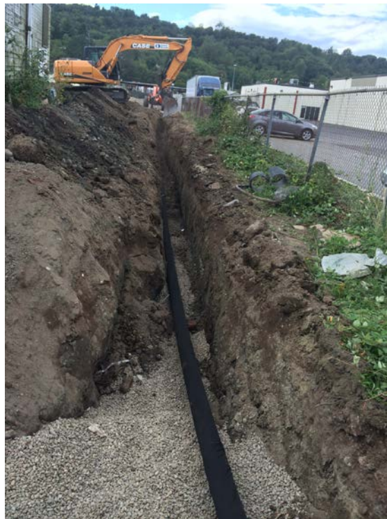
Photograph 14: Backfilling gas collection trench No. 22, looking west.
