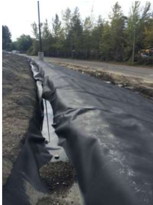
Photo 15: Low- permeability liner anchorage at top of slope
