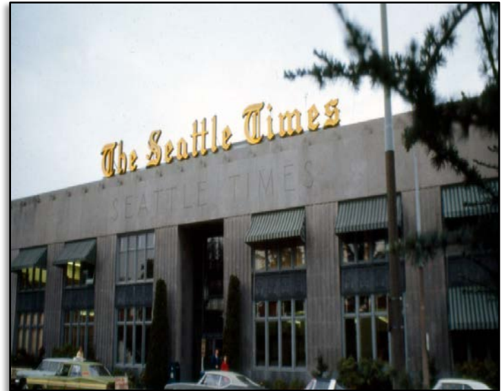
Historical View of Seattle Times Building
