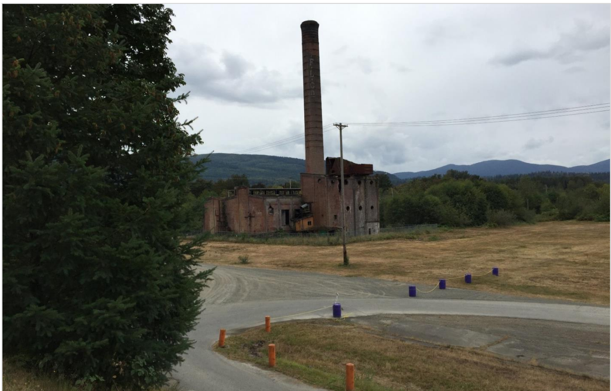
Exhibit 3.9-2. Historic Powerhouse – Viewed from DirtFish Offices (Viewpoint 1)
