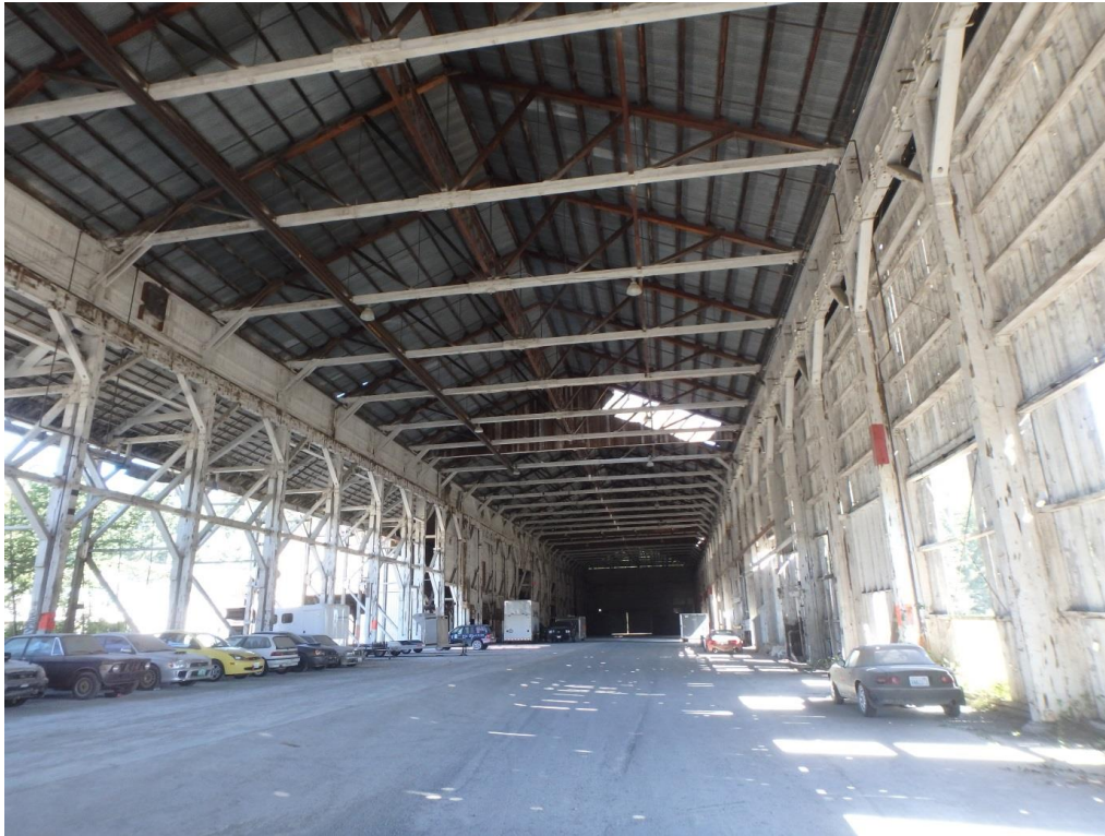
Exhibit 3.10-9. Crane Shed No. 3 Interior, Facing East
