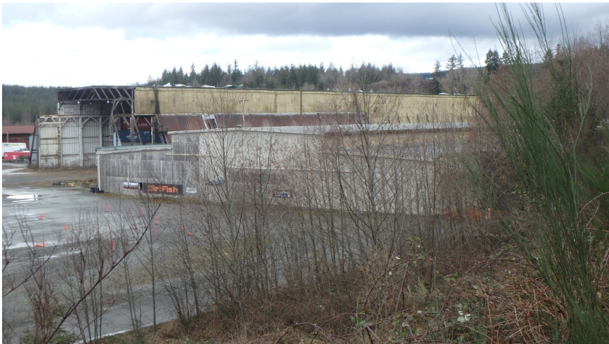
Figure 37. Finished Lumber Shed (right) and Package Lumber Shed south elevations.
