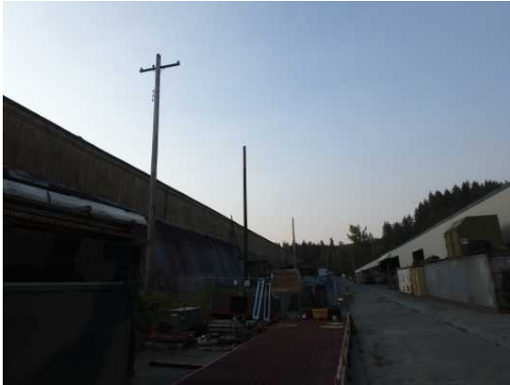
Power poles between Finished Lumber and Package sheds
