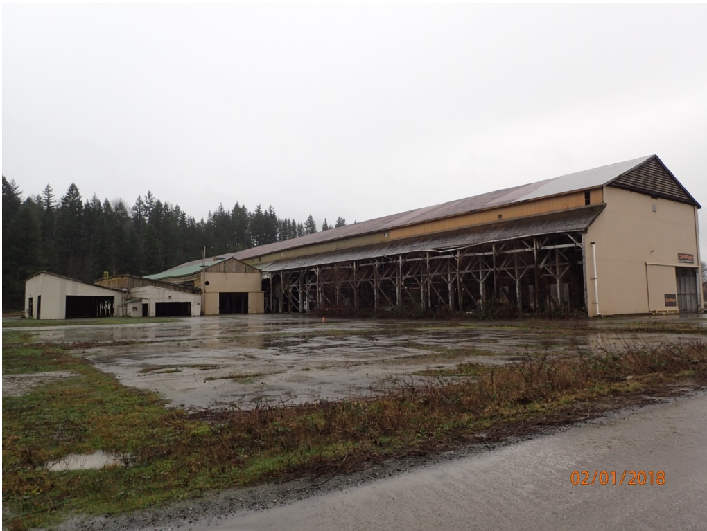
Figure 33. North and west elevations of the Planer Building, with Crane Shed No. 3 (right) and Planing Mill (left).
