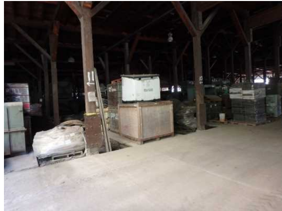
Interior w floor cutouts SW P5031445.JPG
