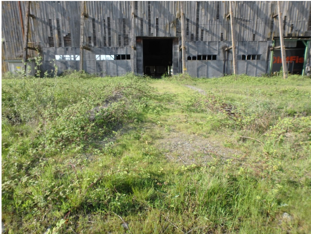
Figure 27. Rail bed approximately 270 ft. west of the east end of Crane Shed No. 3. Facing north.
