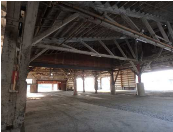
View of interior at the entrance from crane shed
