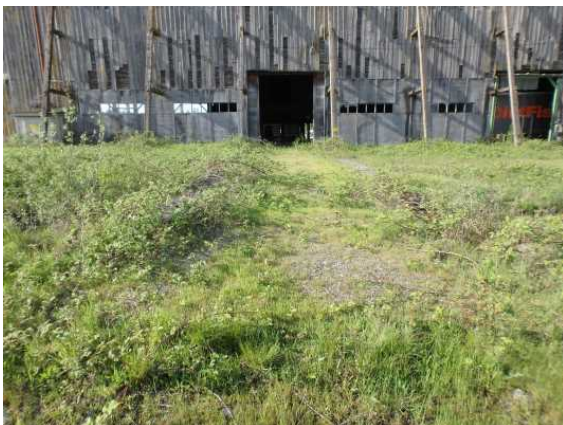
Rail bed between Transfer Shed and Crane Shed No. 3. Approximately 270 ft W of E end of Crane Shed No. 3.
