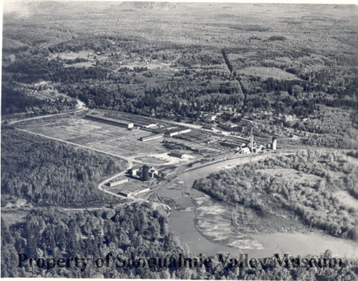
Figure 7. Photographic overview of the SFLCo mill site dated to between the 1930s and 1952 (SVHM PO 558.0120). Facing northeast.
