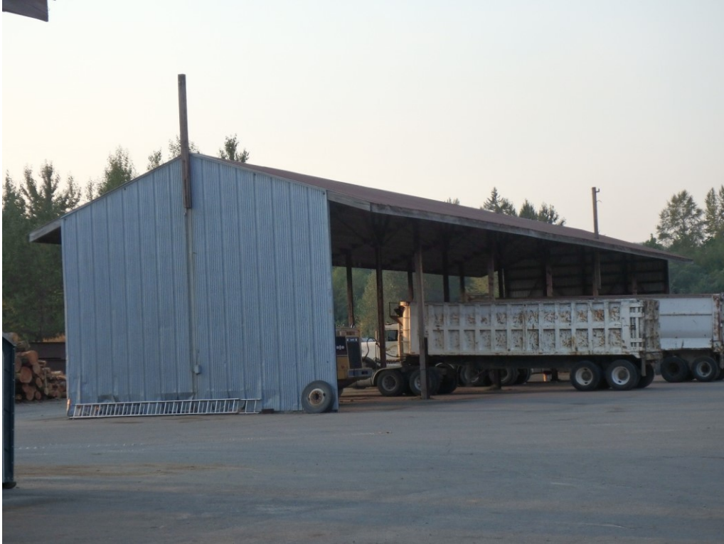
Figure 43. An example of the modern sheds west of the Package Lumber Shed.
