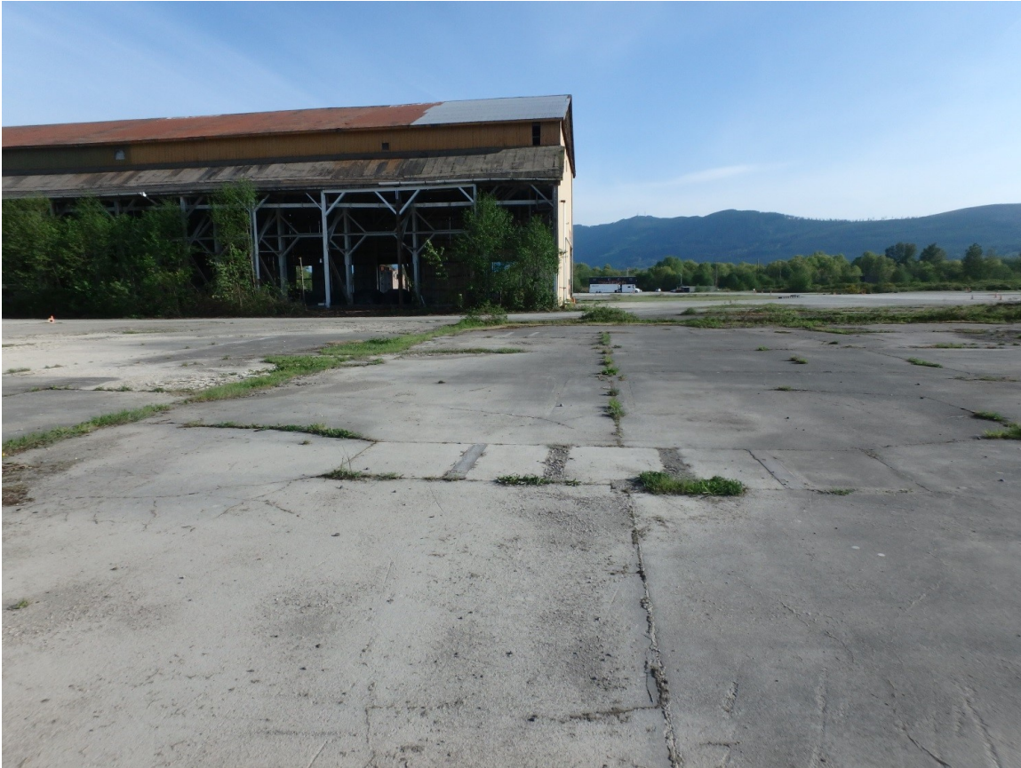
Figure 36. End Glue Plant (foreground), facing south, and Crane Shed No. 3 (background left).
