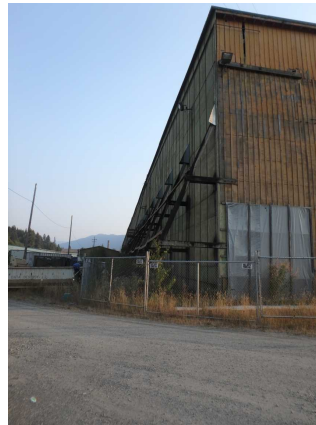
east elevation and corner of the north elevation
