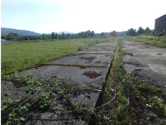
Transfer Shed foundation
