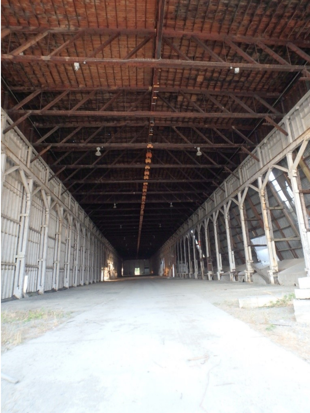
Figure 40. Interior of the Package Shed. Facing north.
