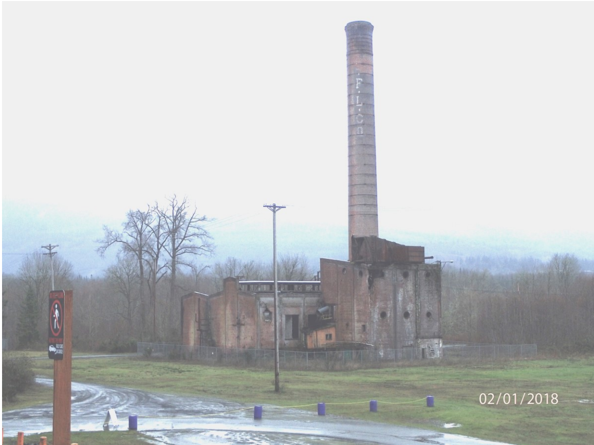
Figure 21. Power Plant north and east elevations. Taken February 2018 from the DirtFish Rally parking lot. Note: Holes in north wall (below chimney and left of utility pole).
