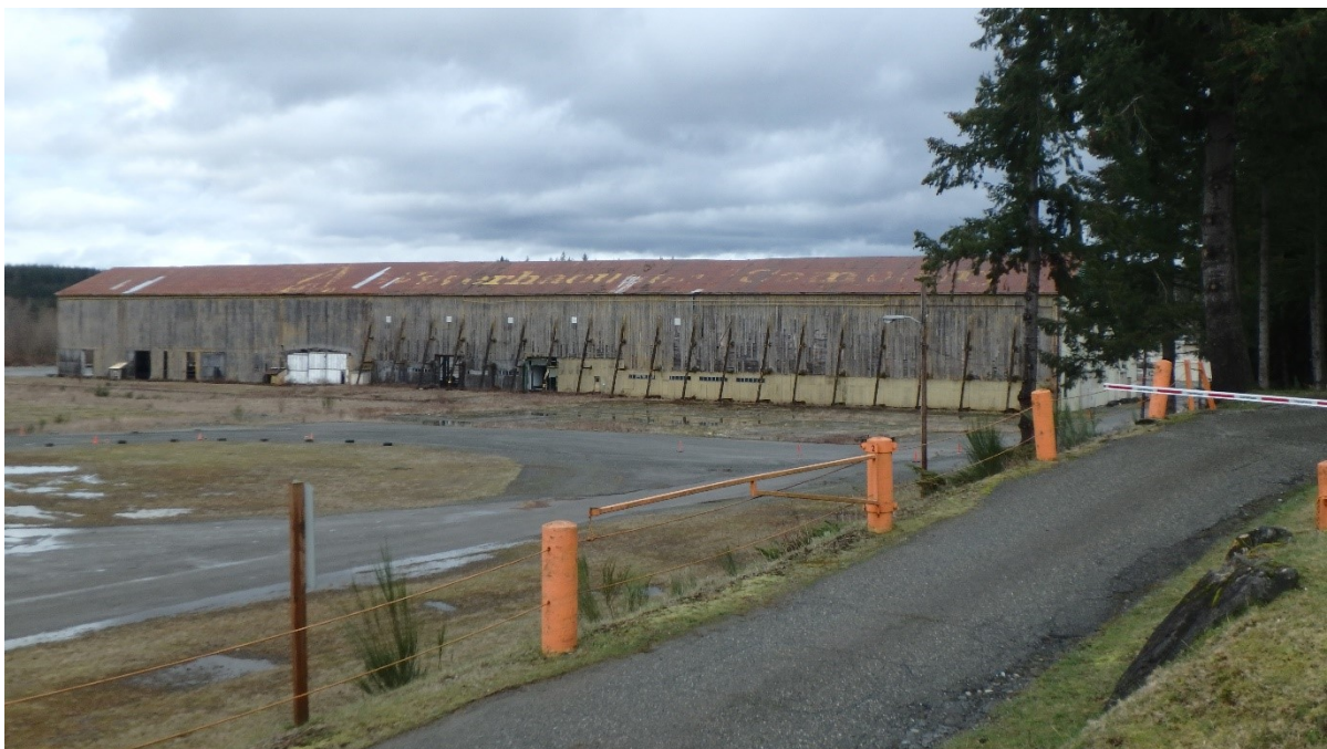
Figure 31. Crane Shed No. 3 south elevation.
