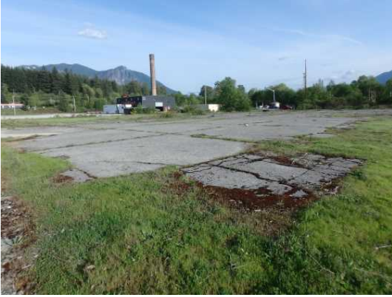
Blacksmith and Machine Shop foundation
