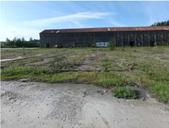
Dry Kilns foundation with Crane Shed No. 3 (background)
