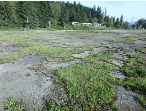
Storage-Salvage Shed foundation
