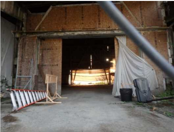
Detail of recent work in north portion
