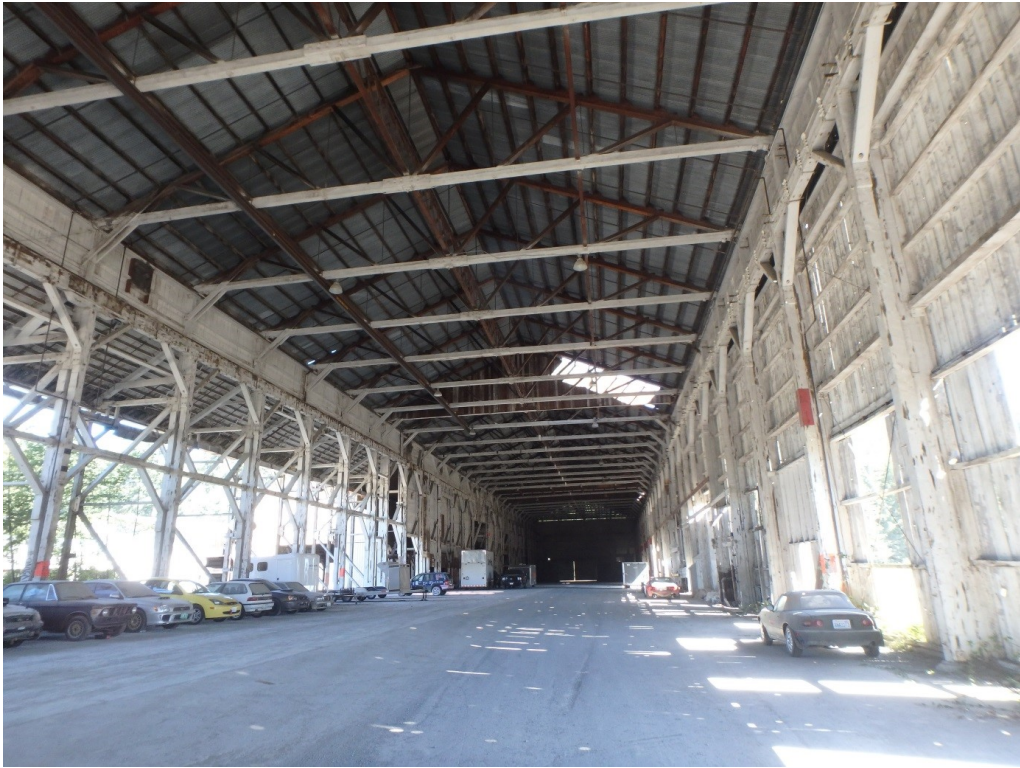
Figure 32. Crane Shed No. 3 interior. Facing east.
