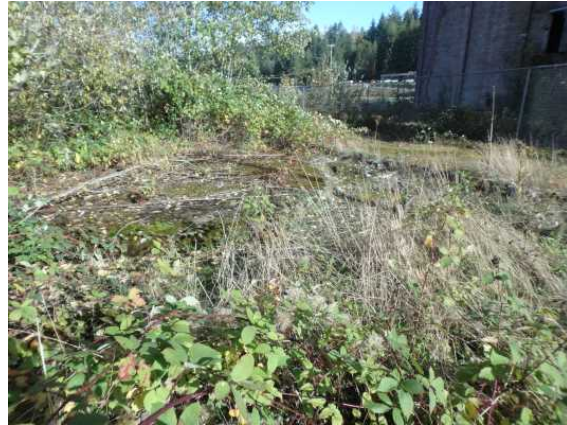
Fuel Vault foundation
