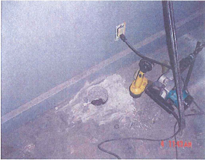
6-4-07 VIMS-5A Puget Sound Pipe (Facing South East) - Drilled concrete sump
