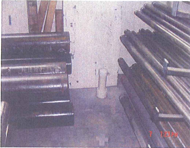
6-7-07 VIMS-1 Puget Sound Pipe (Facing North) – Capped Riser after excavation of sump
