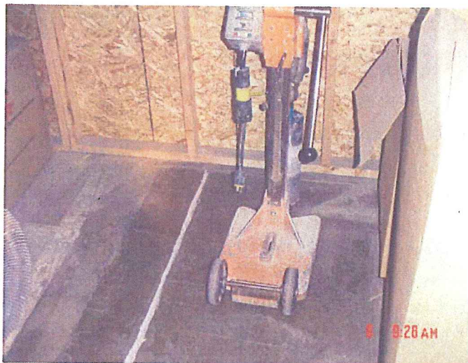
6-6-07 VIMS-3 Hudson Bay Warehouse (Facing West) - Drill set up to core out concrete
