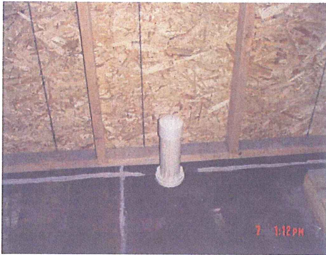
6-6-07 VIMS-3 Hudson Bay Warehouse (Facing West) – Capped Riser after excavation of sump
