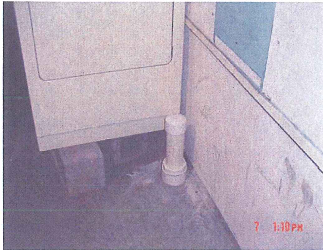
6-7-07 VIMS-5B Hudson Bay Warehouse (Facing Northeast) – Capped Riser after excavation of sump
