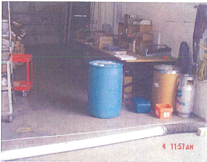
6-4-07 VIMS-1 Puget Sound Pipe Warehouse (Facing North) – Shows polyurethane sealing and installation vent piping from vacuum blower.
