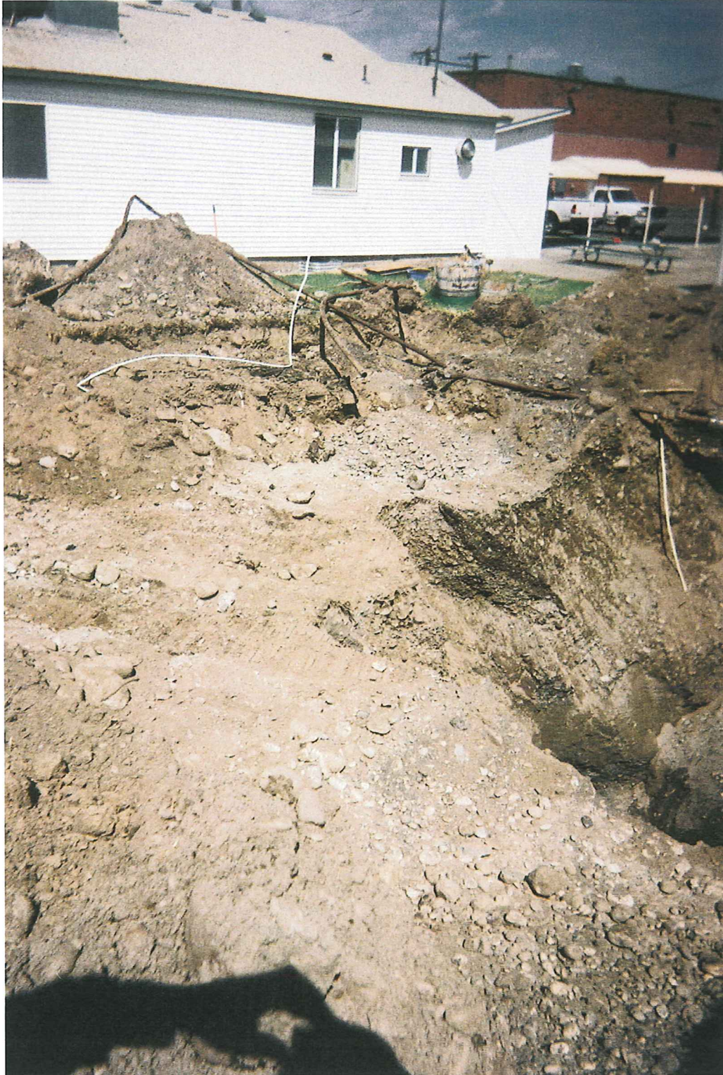
PHOTO 8: LOOKING NE ACROSS FINAL EXCAVATION
