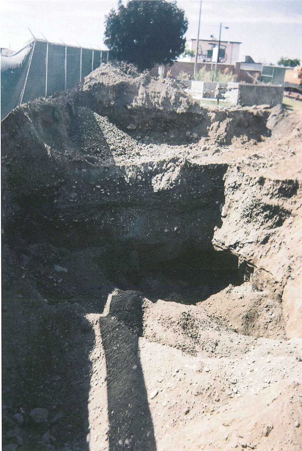
PHOTO 7: LOOKING WEST ACROSS FINAL EXCAVATION
