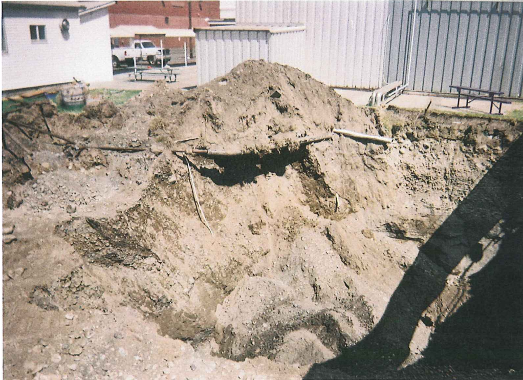
PHOTO 5: LOOKING NORTHEAST ACROSS EXCAVATION
