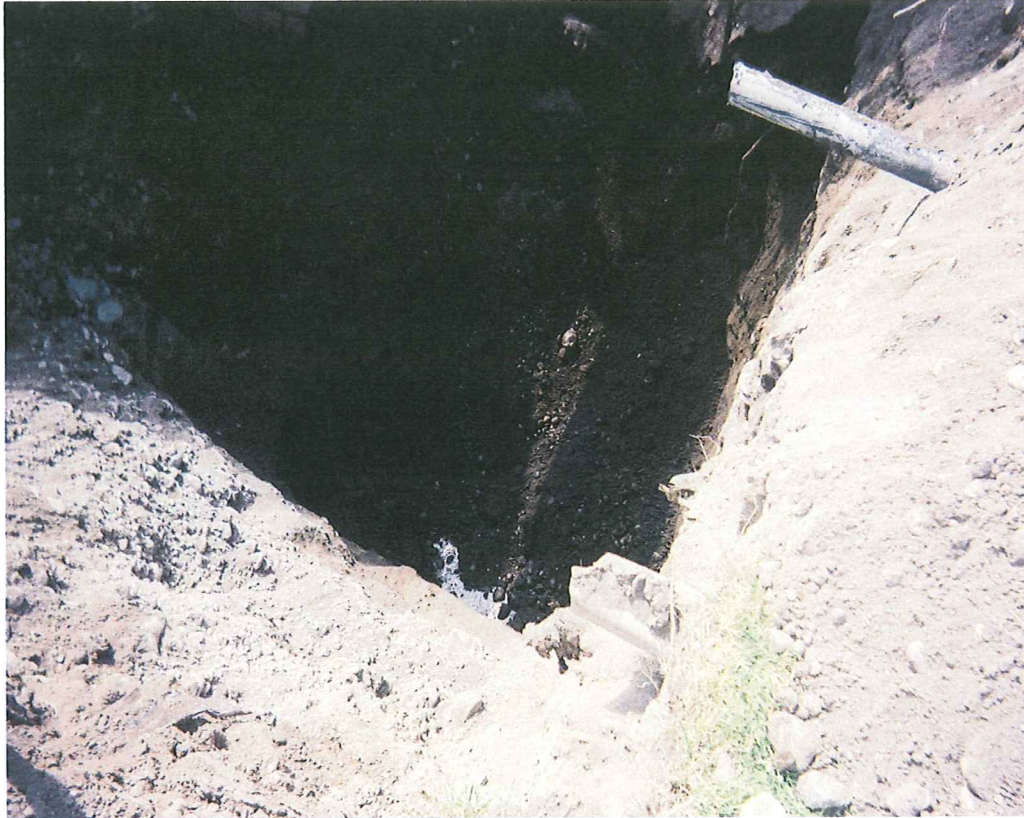
PHOTO 2: GROUNDWATER IN BASE OF EXCAVATION
