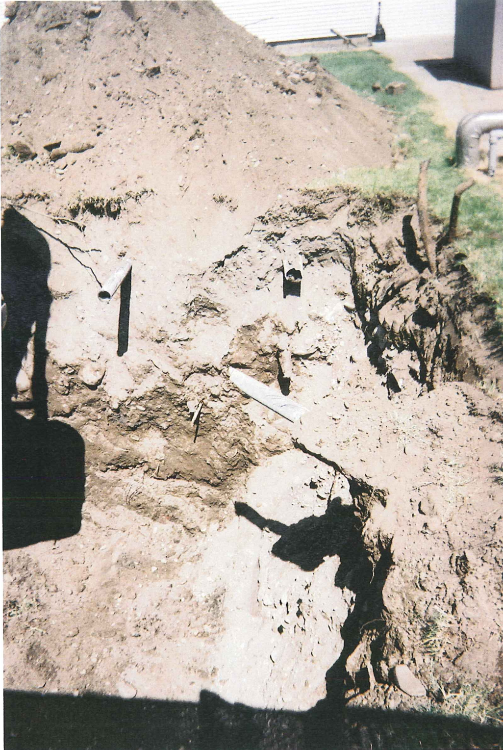
PHOTO 3: LOOKING NORTH AT OIL LINES & DRAINS DURING EXCAVATION PROCESS
