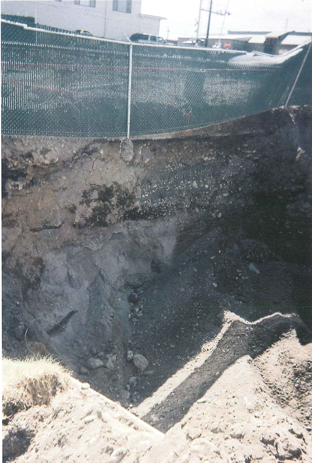
PHOTO 1: LOOKING SW AT FINAL EXCAVATION
