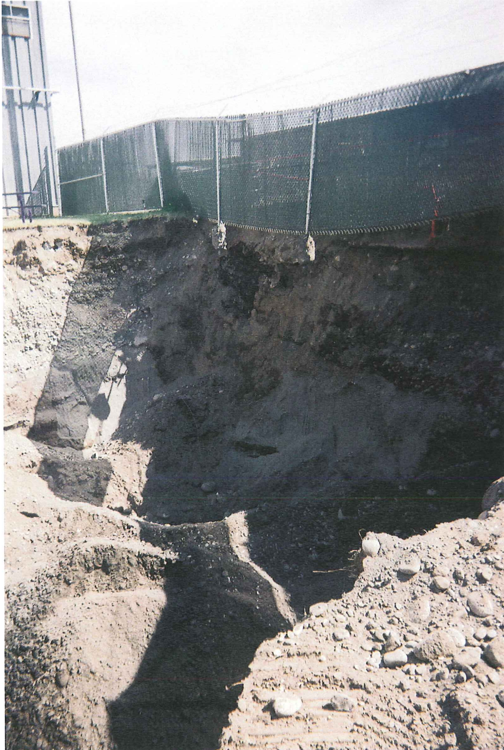
PHOTO 4: LOOKING EAST AT FINAL EXCAVATION
