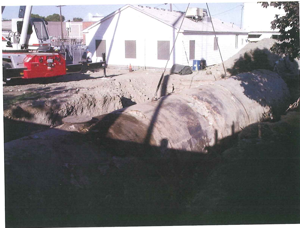
PHOTO 1: BEGINNING THE LIFT TO REMOVE TANK, LOOKING NORTH EAST
