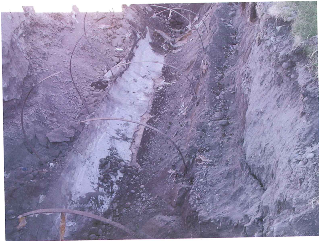
PHOTO 4: PIT BASE AFTER REMOVING TANK
