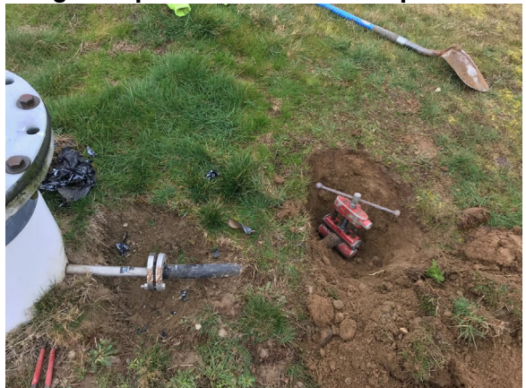
Replaced damaged 1-1/2" rubber gasket at flange adapter on condensate trap CS-10
