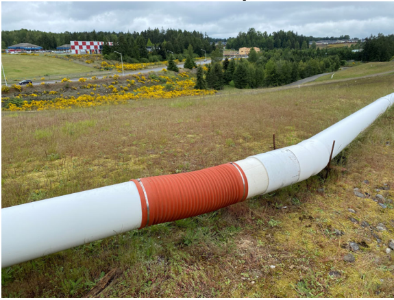
Installed 12"x3' Header Pipe at N-8 (1)
