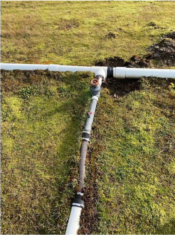
3" Tee and 3" LFG Hose Repaired at N-32 (1)
