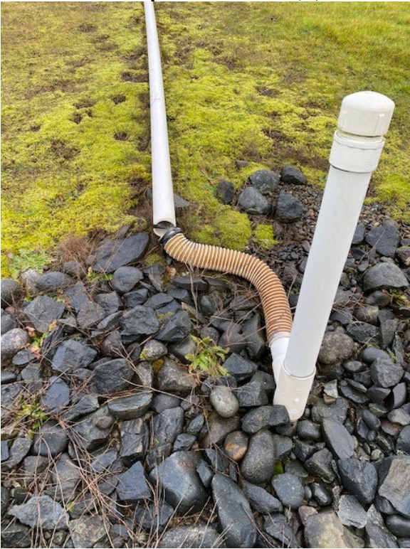
3" LFG Hose Replaced at N-57 (1)
