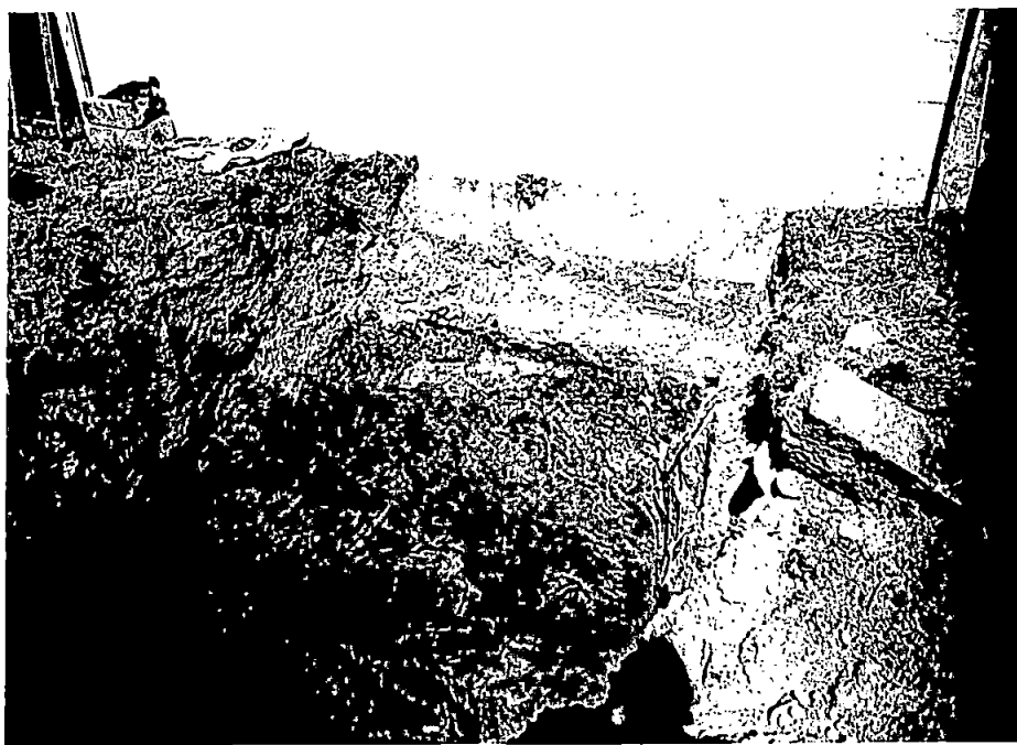
PCS "chased" to foundation, and extending under building
