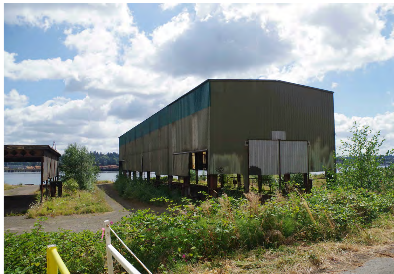
EXISTING ADJACENT ABANDONED STRUCTURE LOCATED SOUTH OF SITE
