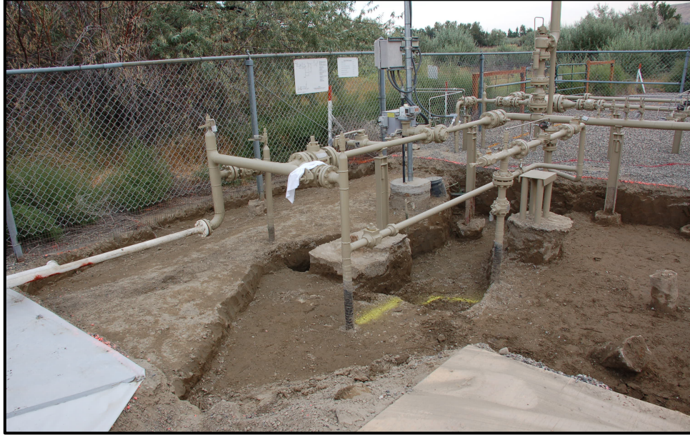
1. Look at initial excavation.
