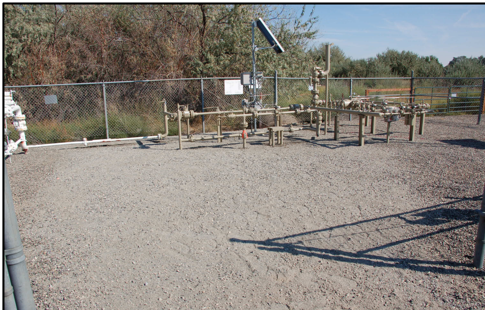
2. Looking at completed excavation.
