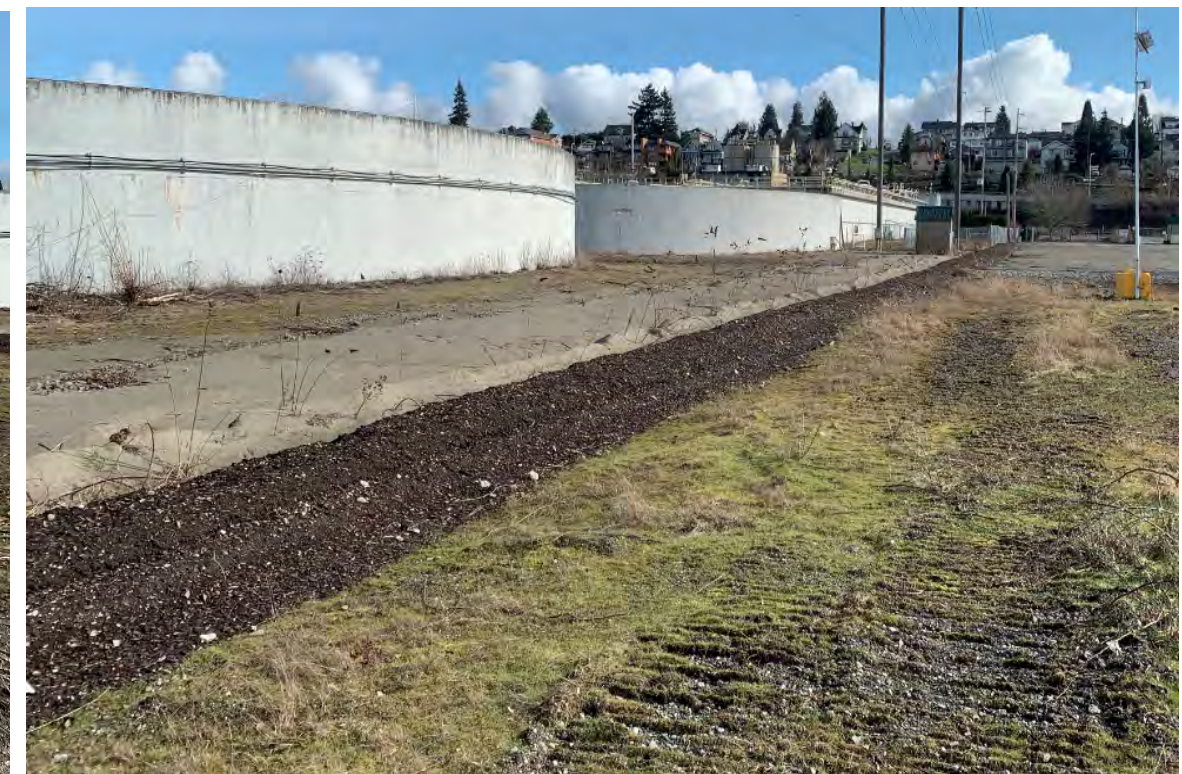
P6 - EXISTING CONCRETE BLOCK BARRIER AND BERM ALONG SITE'S NORTH SIDE. LOOKING NORTH EAST.
