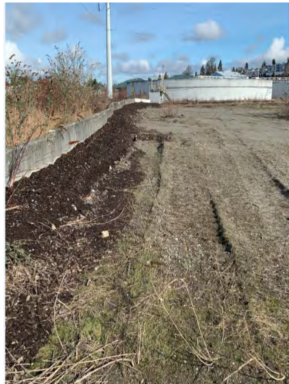
P4 - EXISTING CONCRETE BLOCK BARRIER AND BERM ALONG SITE'S WEST SIDE AT NORTH END. LOOKING NORTH.
