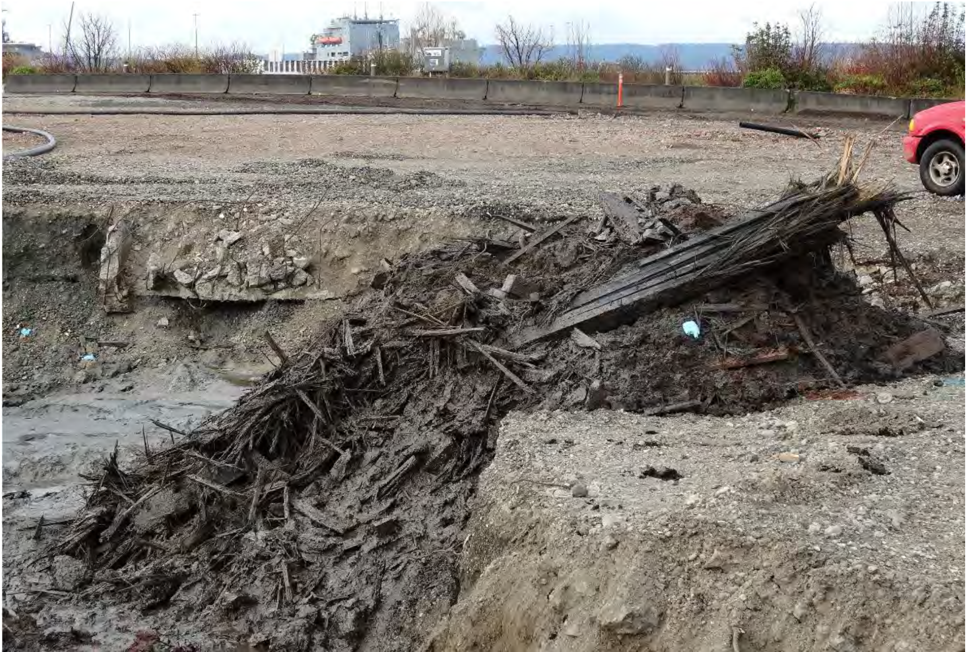
Excavation showing crushed material and wood debris
