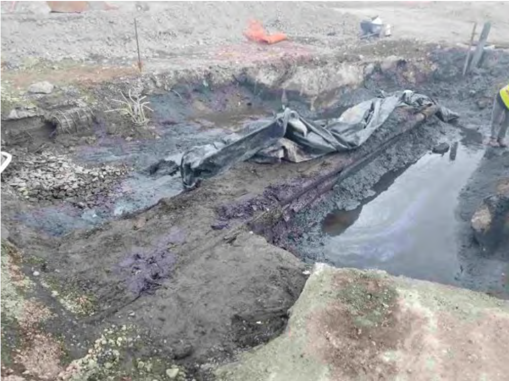
One Bunker C fuel pipe encountered within wooden conduit, stained soil with sheen on water, looking north
