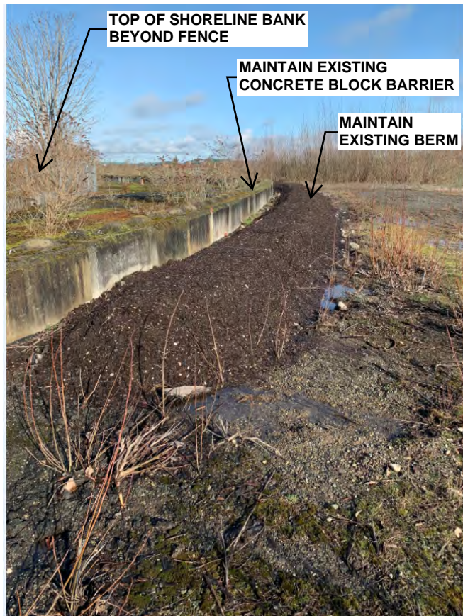
P1 - END OF BERM AT SOUTH END LOOKING NORTH. BERM WILL BE EXTENDED 85-FEET TO FORM A CONTINUOUS BARRIER WITH NO GAPS. BERM WILL TIE TO AN EXISTING CONCRETE BLOCK BARRIER.
