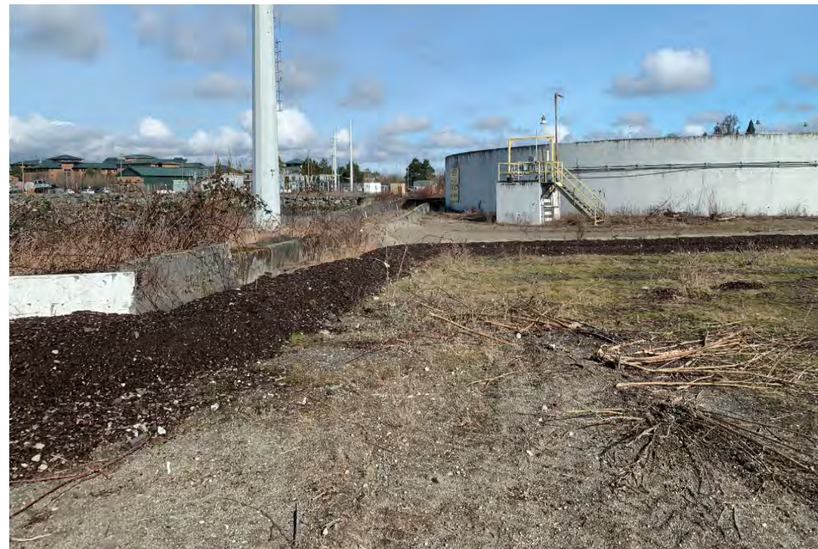
P5 - EXISTING CONCRETE BLOCK BARRIER AND BERM AT SITE'S NORTHWEST CORNER. LOOKING NORTH.
