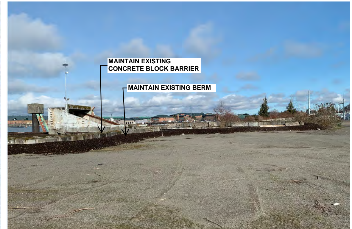
P3 - EXISTING CONCRETE BLOCK BARRIER AND BERM ALONG MIDDLE OF SITE'S WEST SIDE. LOOKING NORTH.
