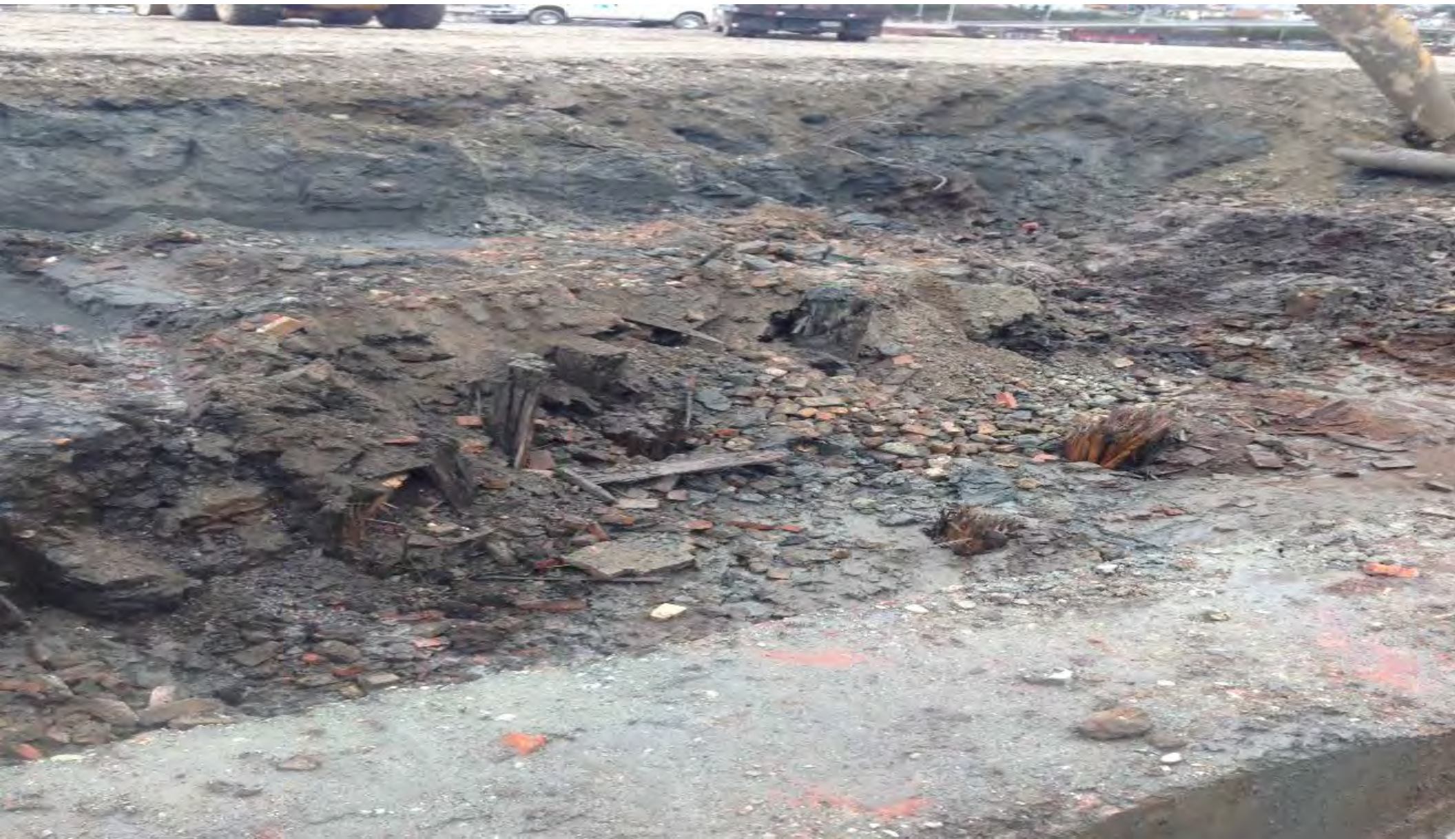
CN-B2 excavation: looking southeast showing brick, wood debris, and creosote piling remnants
