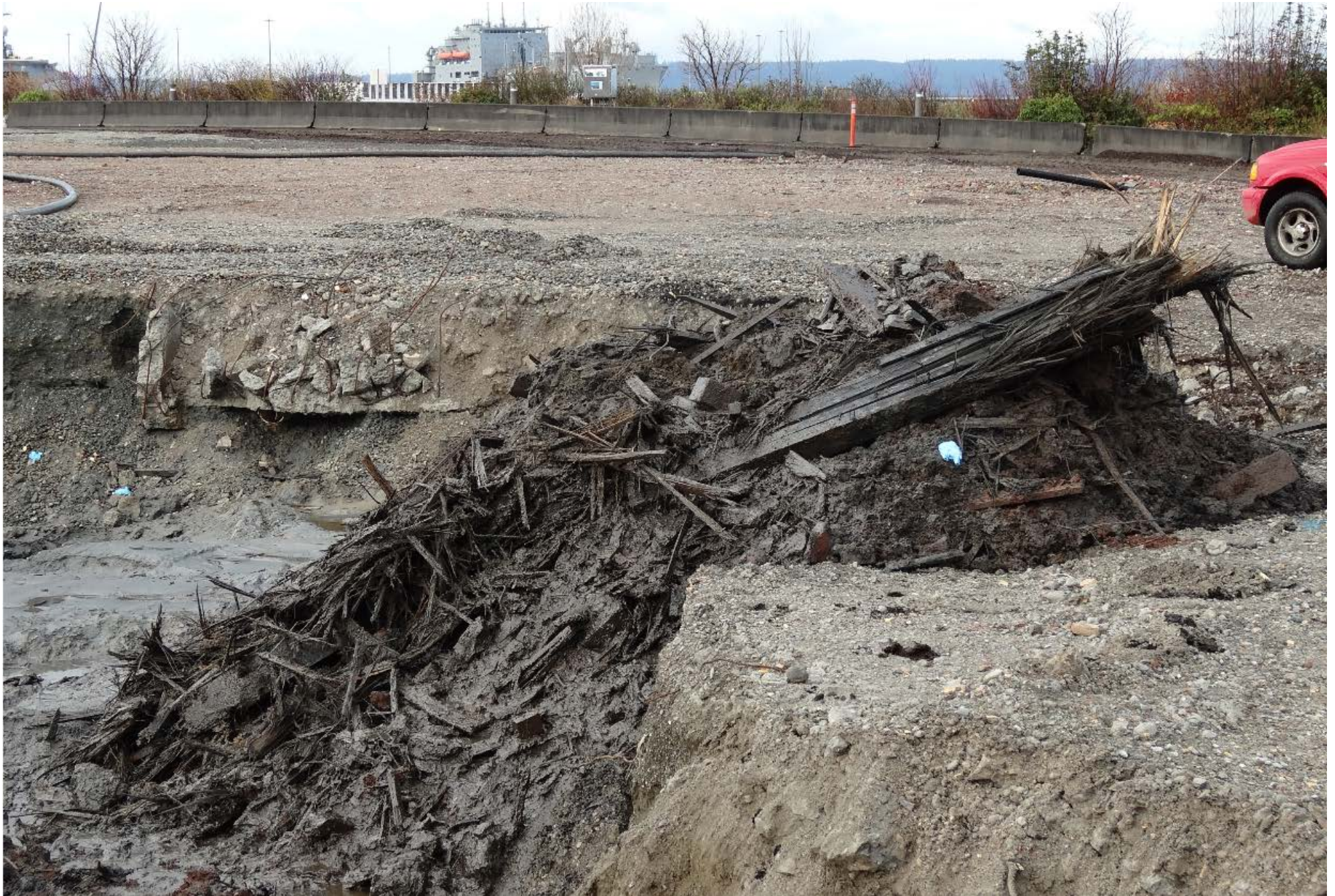
Excavation showing crushed material and wood debris
