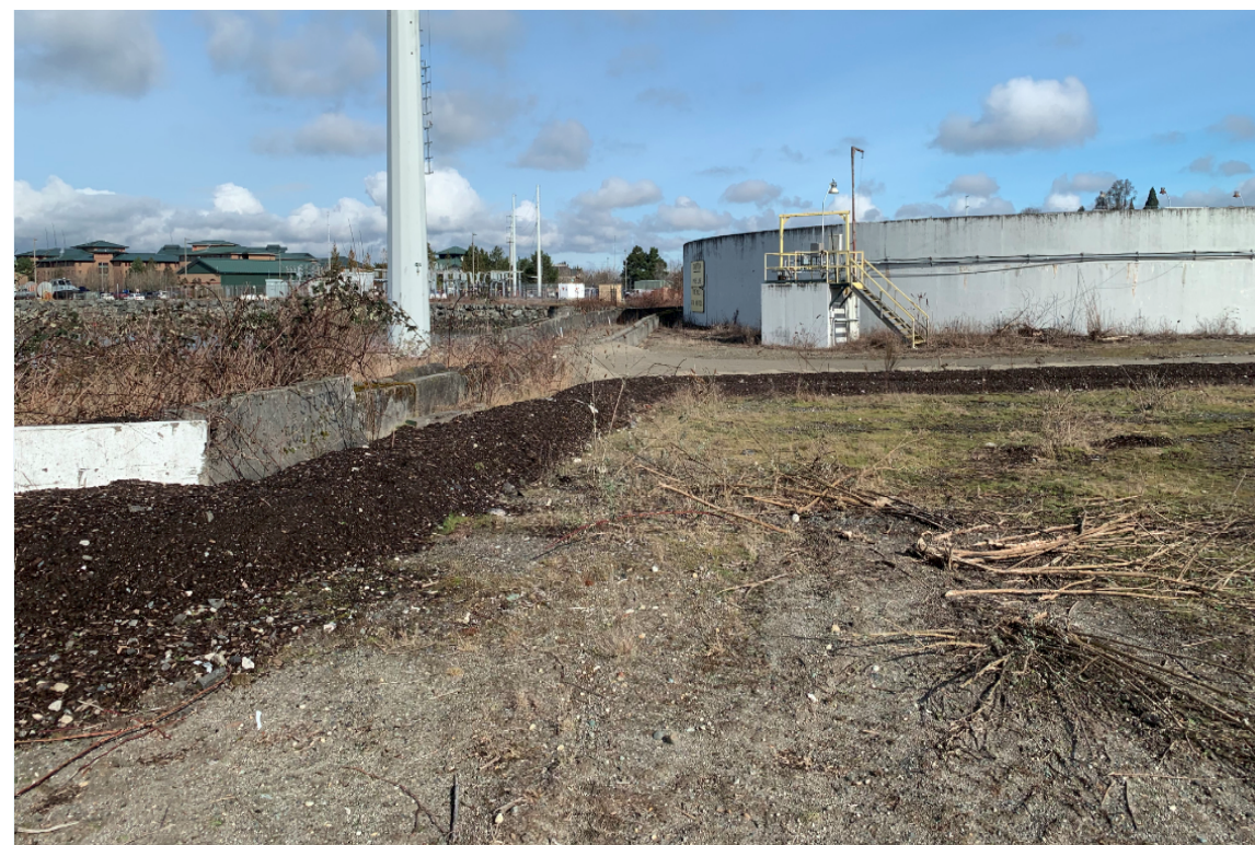
P5 - EXISTING CONCRETE BLOCK BARRIER AND BERM AT SITE'S NORTHWEST CORNER. LOOKING NORTH.
