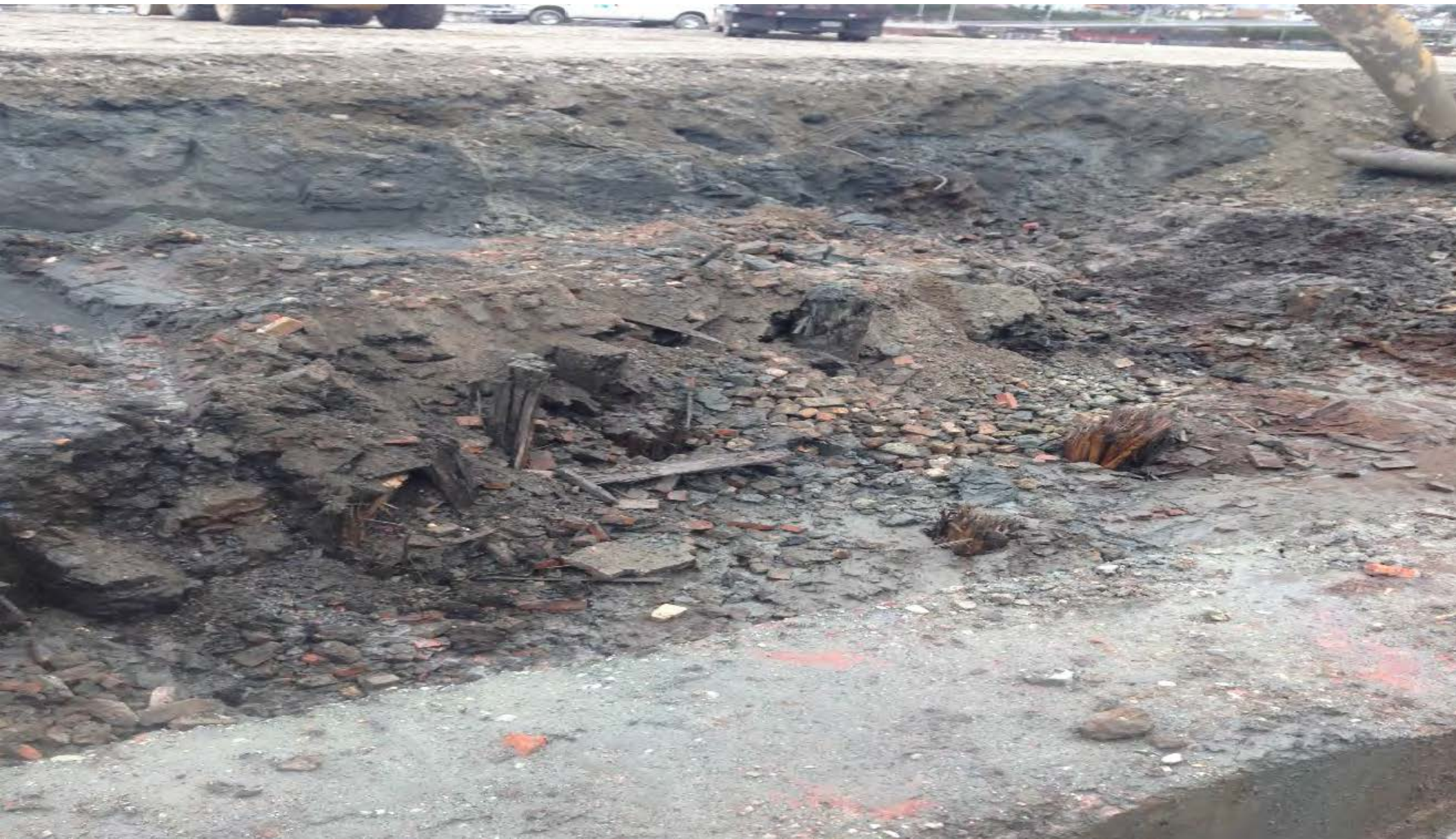
CN-B2 excavation: looking southeast showing brick, wood debris, and creosote piling remnants
