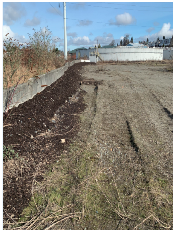
P4 - EXISTING CONCRETE BLOCK BARRIER AND BERM ALONG SITE'S WEST SIDE AT NORTH END. LOOKING NORTH.
