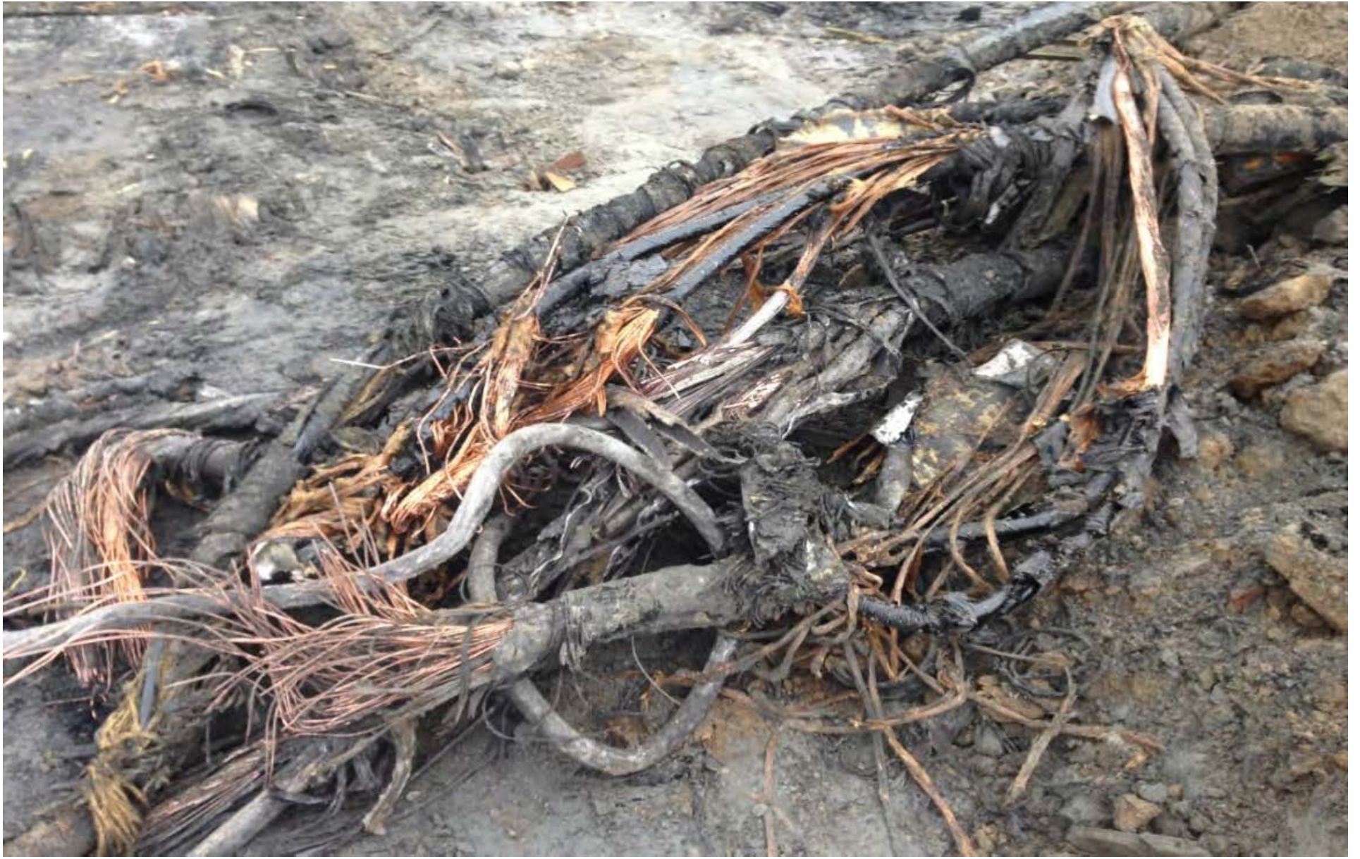
Boiler Baghouse Area excavation: copper wire in east end
