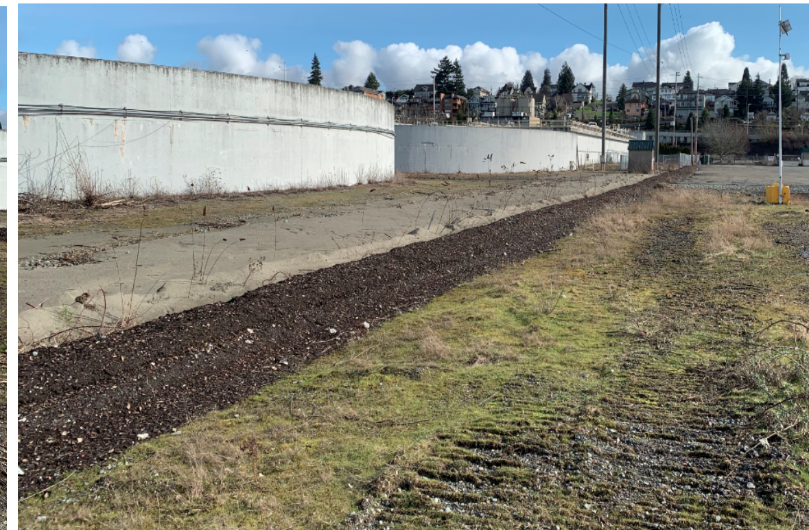
P6 - EXISTING CONCRETE BLOCK BARRIER AND BERM ALONG SITE'S NORTH SIDE. LOOKING NORTH EAST.
