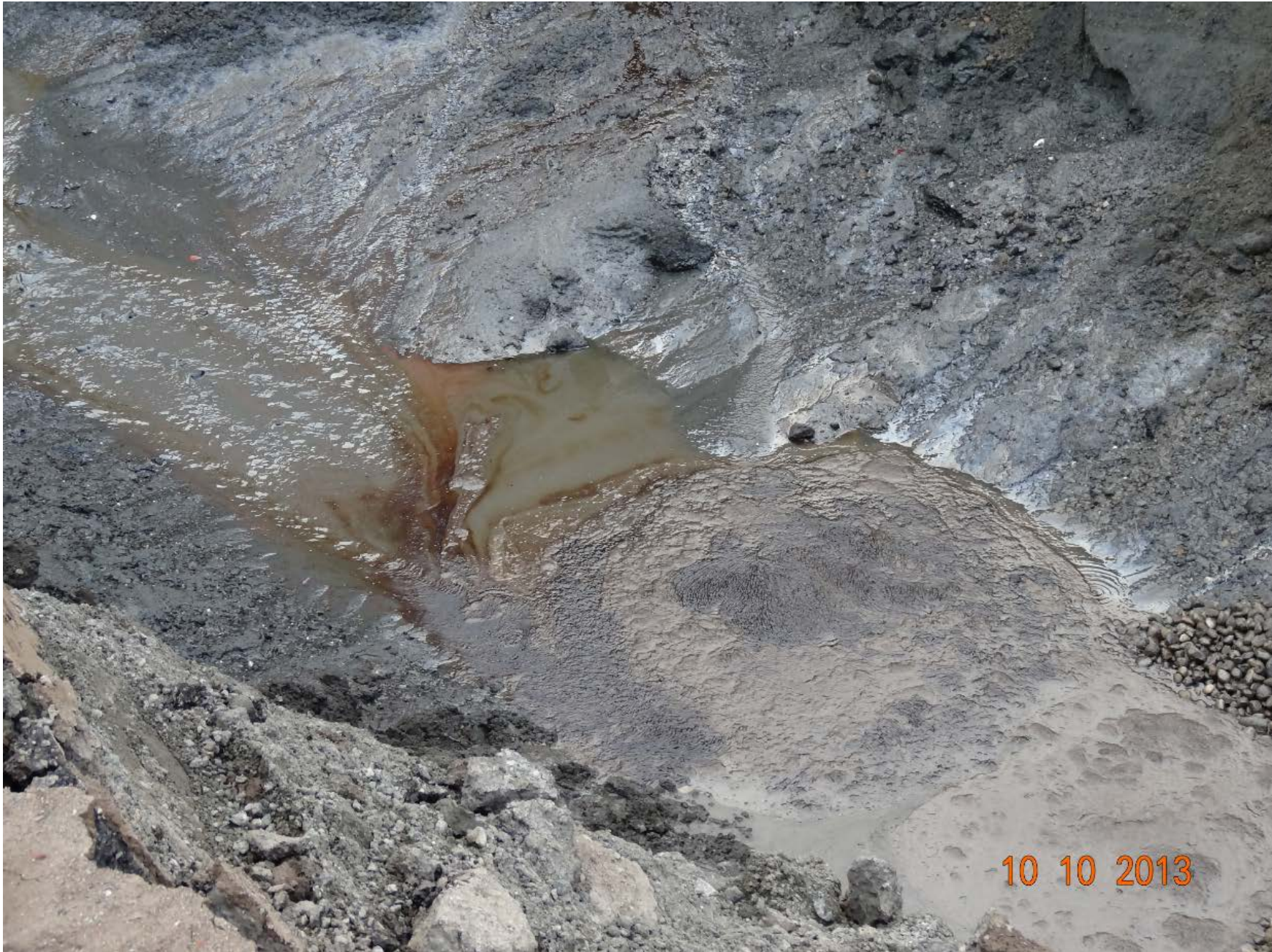
Bunker C ASTs excavation: bunker oil product
