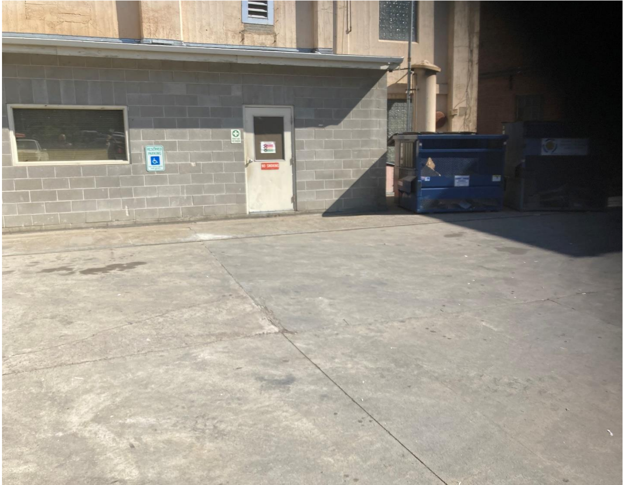
Photo 1: Boiler Room – from the southeast
