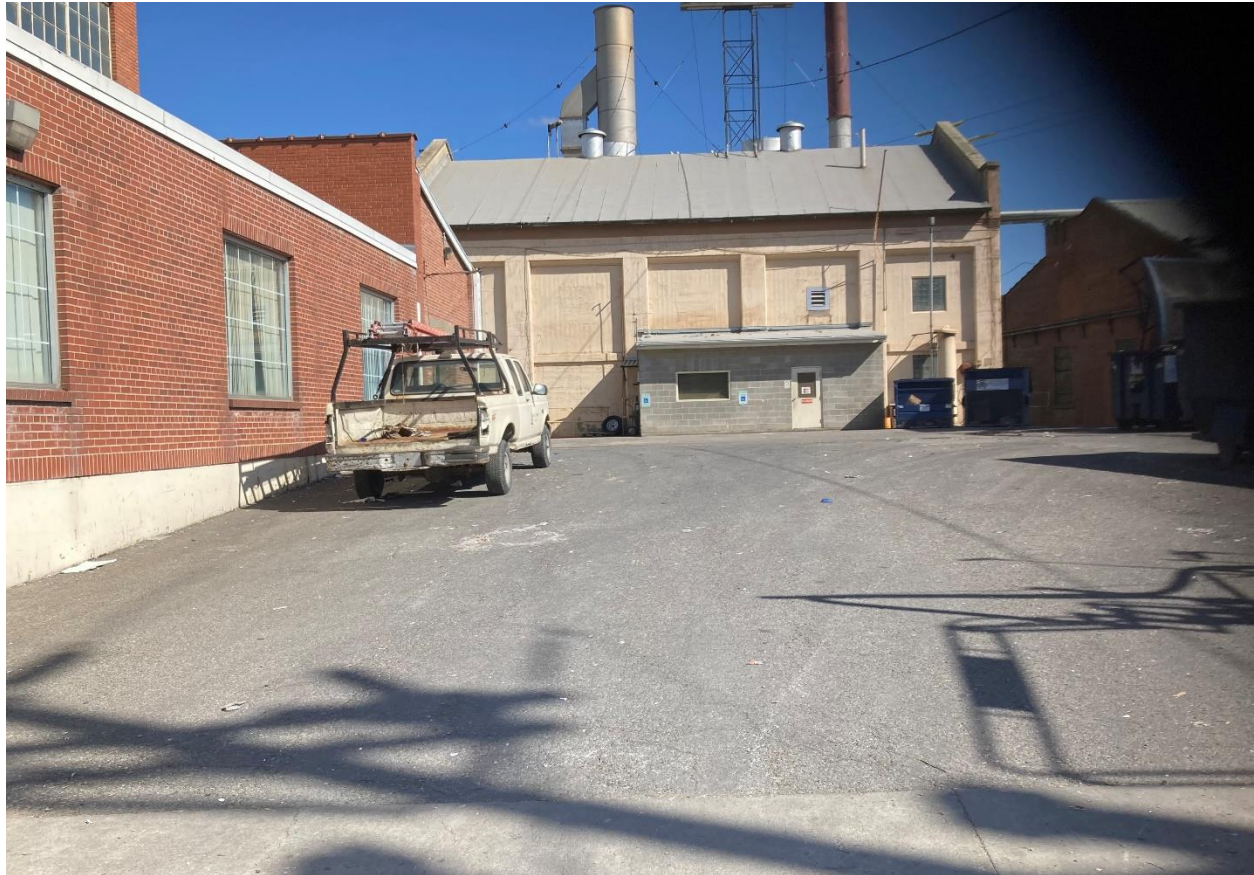
Photo 3: Boiler Room – from the south
