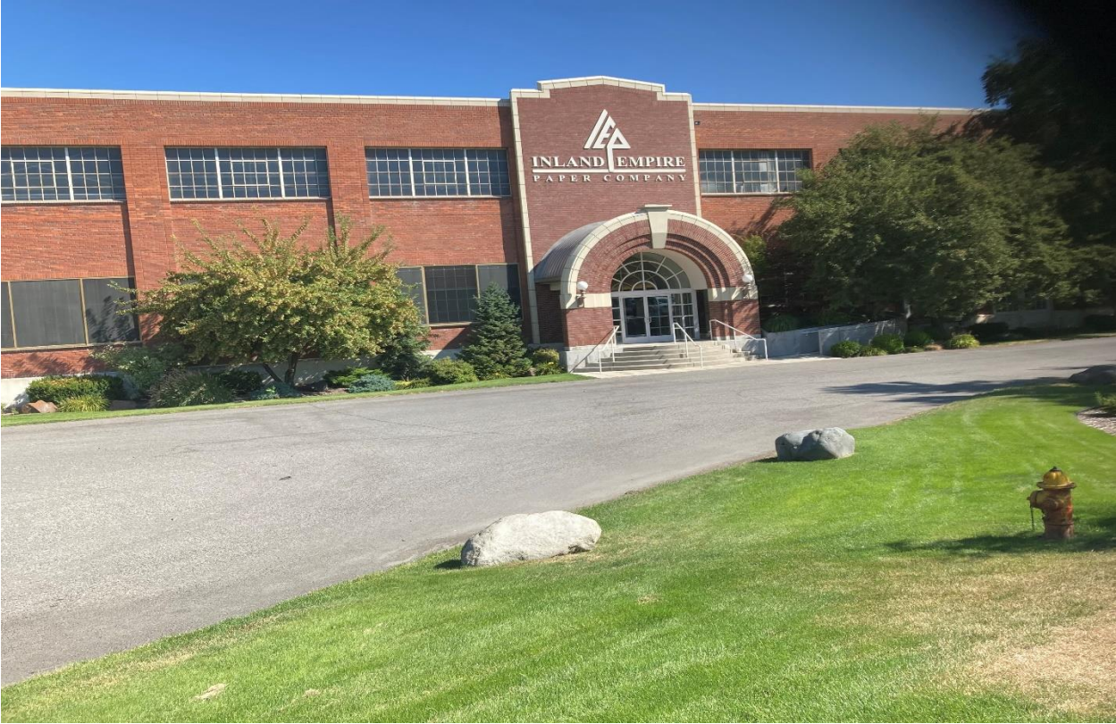
Photo 2: Site Entrance and Front of IEP – from the southwest
