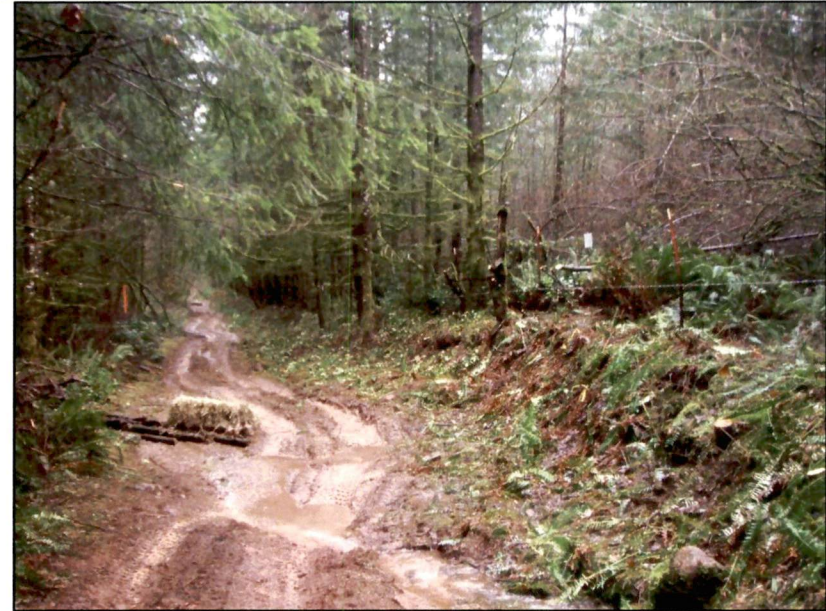
East View of Middle of Grid H-22
