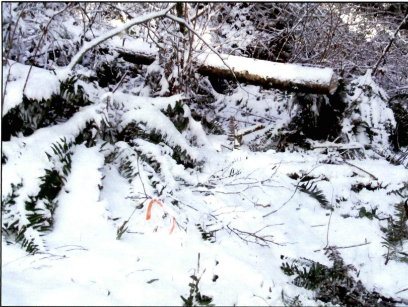
Collapsed Fence of Grid EE-27
