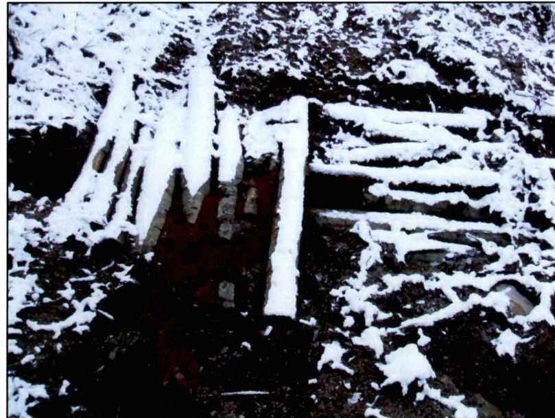
Middle View of Grid Y-18 (Bridge #2)
