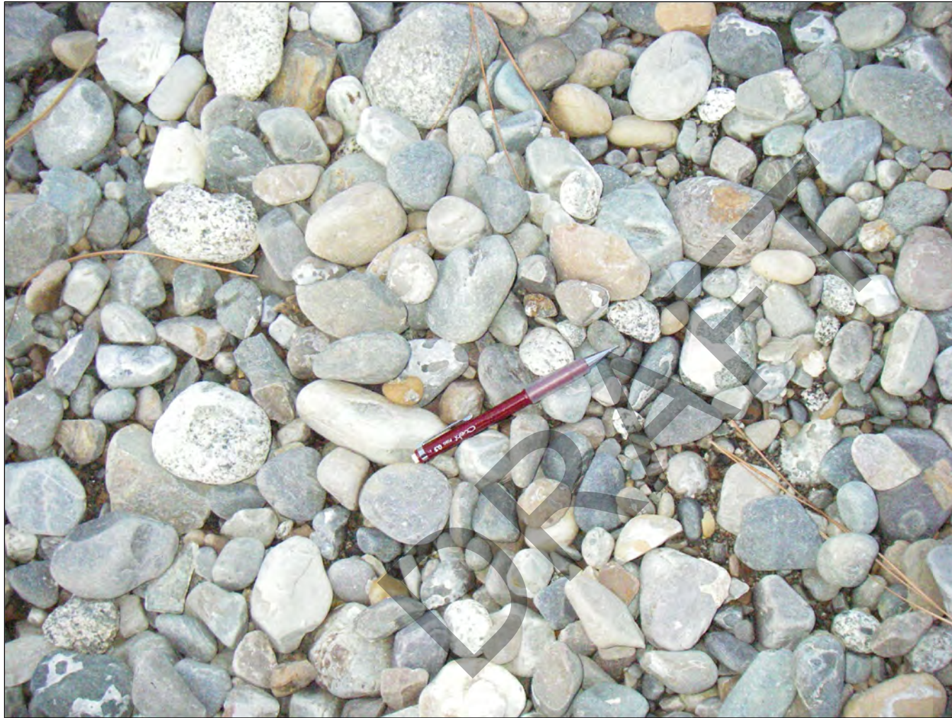
View of remaining capping material installed prior to the Spokane River high flow event in May of 2011 (pencil added for scale).
