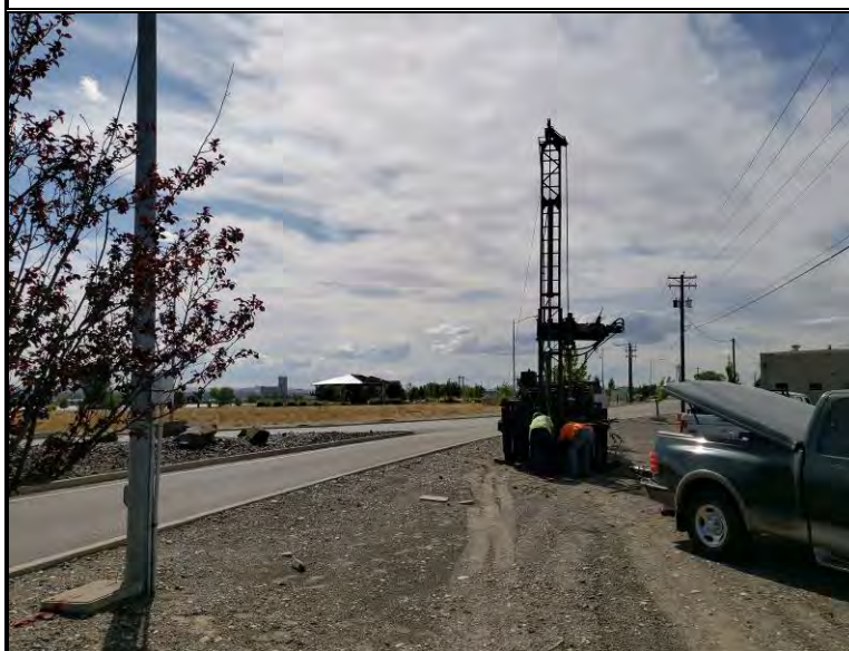
Drilling at borehole B-8, looking west
