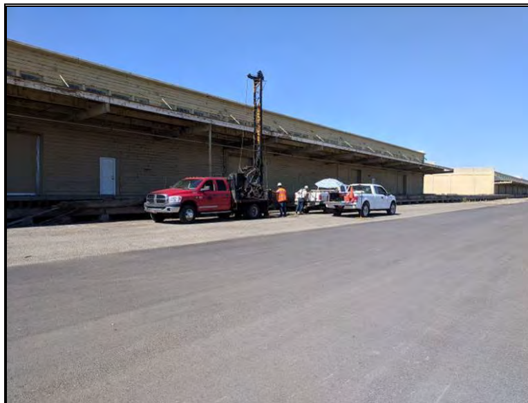
Drilling at borehole B-1, looking west
