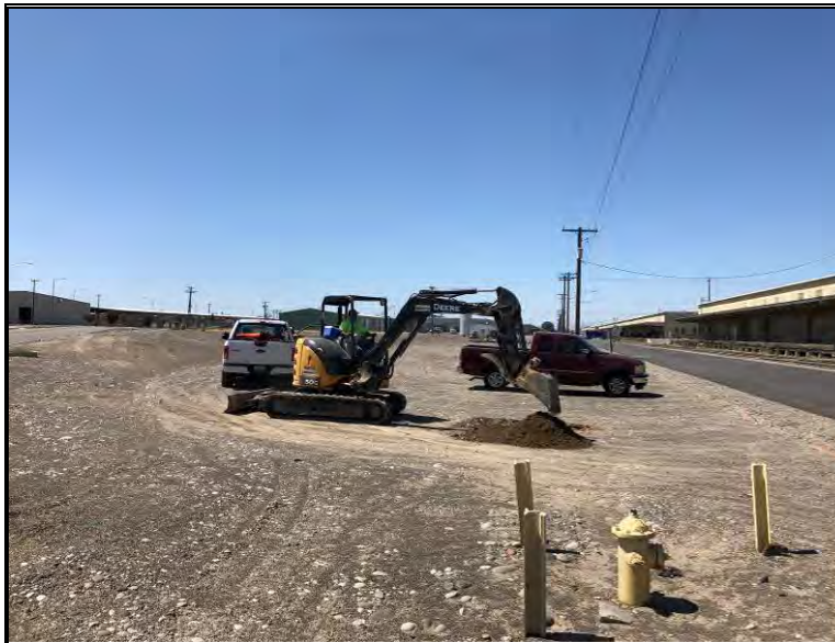
Excavation of test-pit TP-4, looking west
