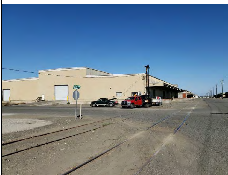
Drilling at borehole B-7/MW-2, looking east
