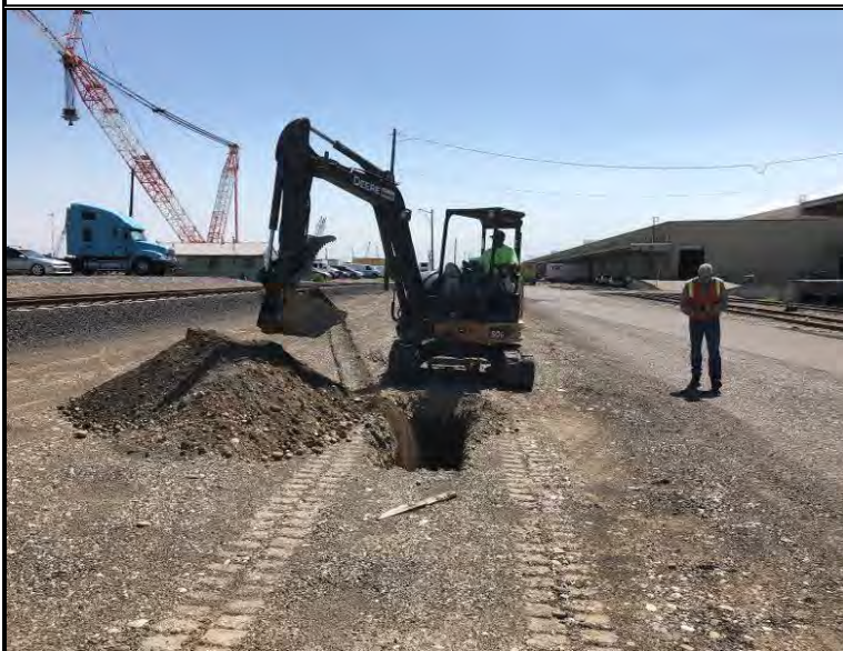
Excavation of test-pit TP-2, looking southeast
