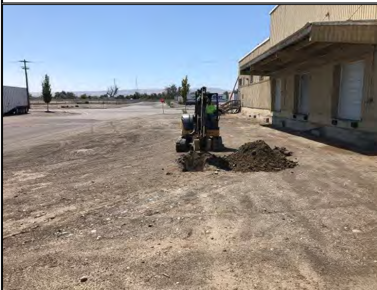
Excavation of test-pit TP-3, looking south
