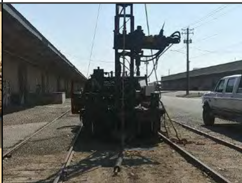
Drilling at borehole B-11, looking southeast
