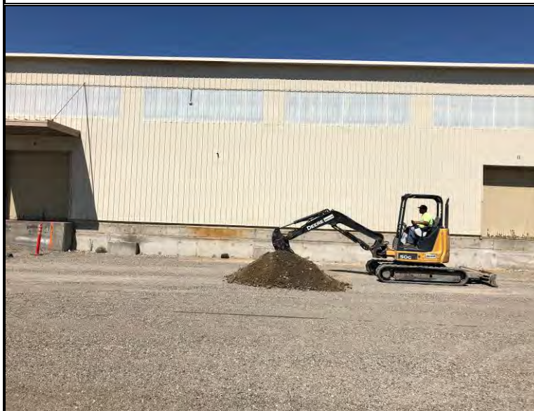
Excavation of test-pit TP-5, looking north
