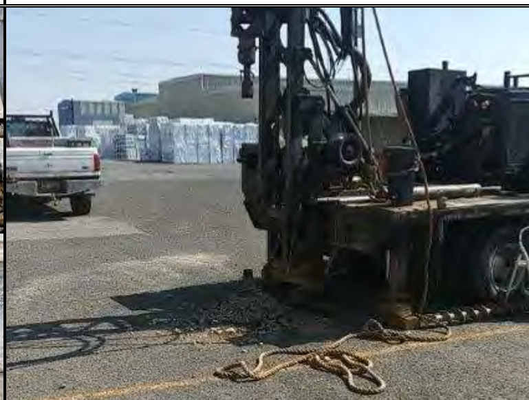
Drilling at borehole B-10, looking north
