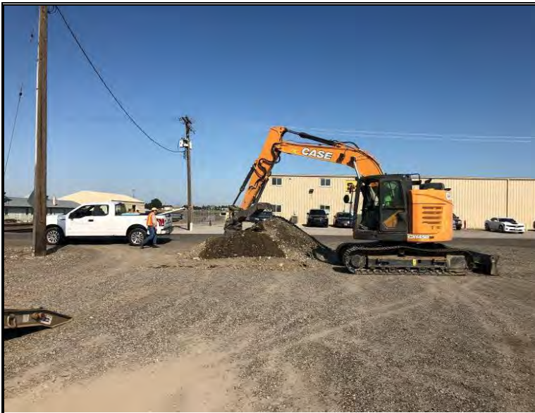
Excavation of test-pit TP-1, looking west
