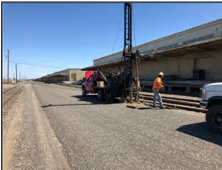
Drilling at borehole B-6, looking south/southeast
