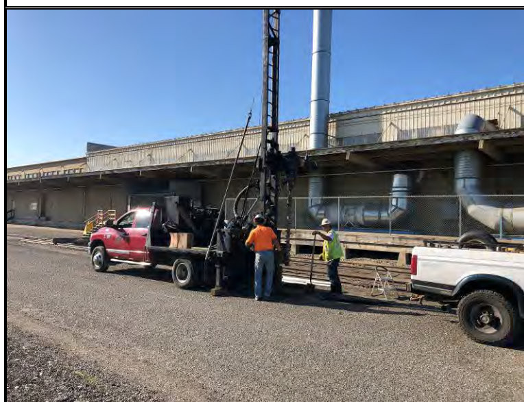
Drilling at borehole B-4, looking south
