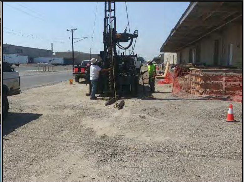
Drilling at borehole B-14, looking west
