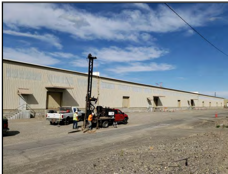
Drilling at borehole B-9, looking northeast
