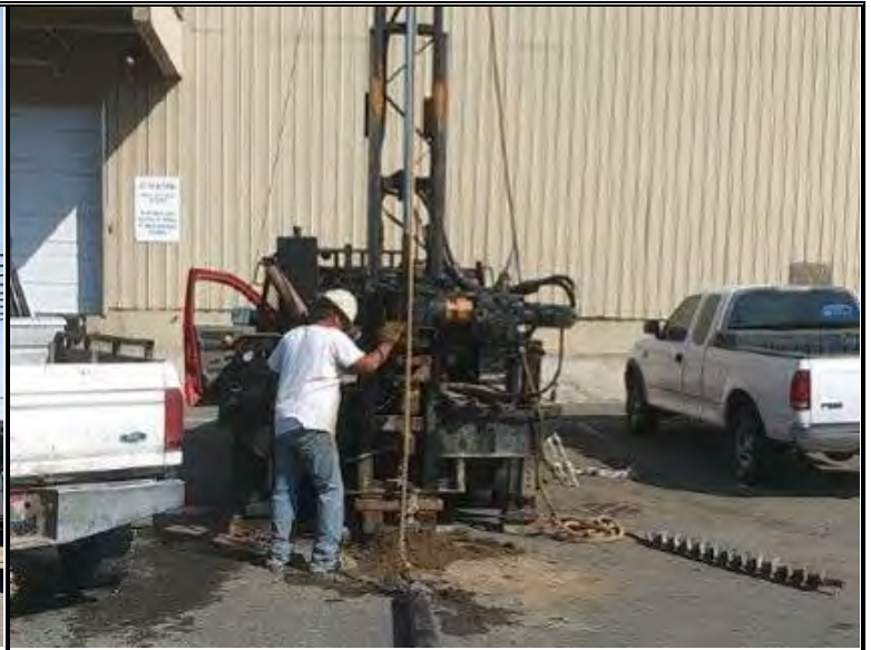
Drilling at borehole B-13
