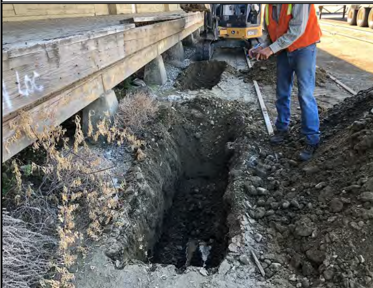
Test-pit P-8 after excavation
