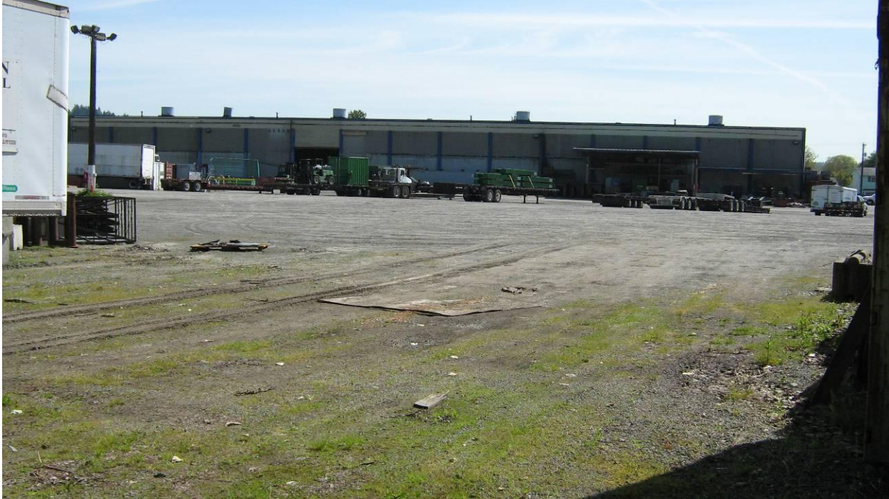
Photo 3: Slag Excavation Area Surface Cover – from the west
