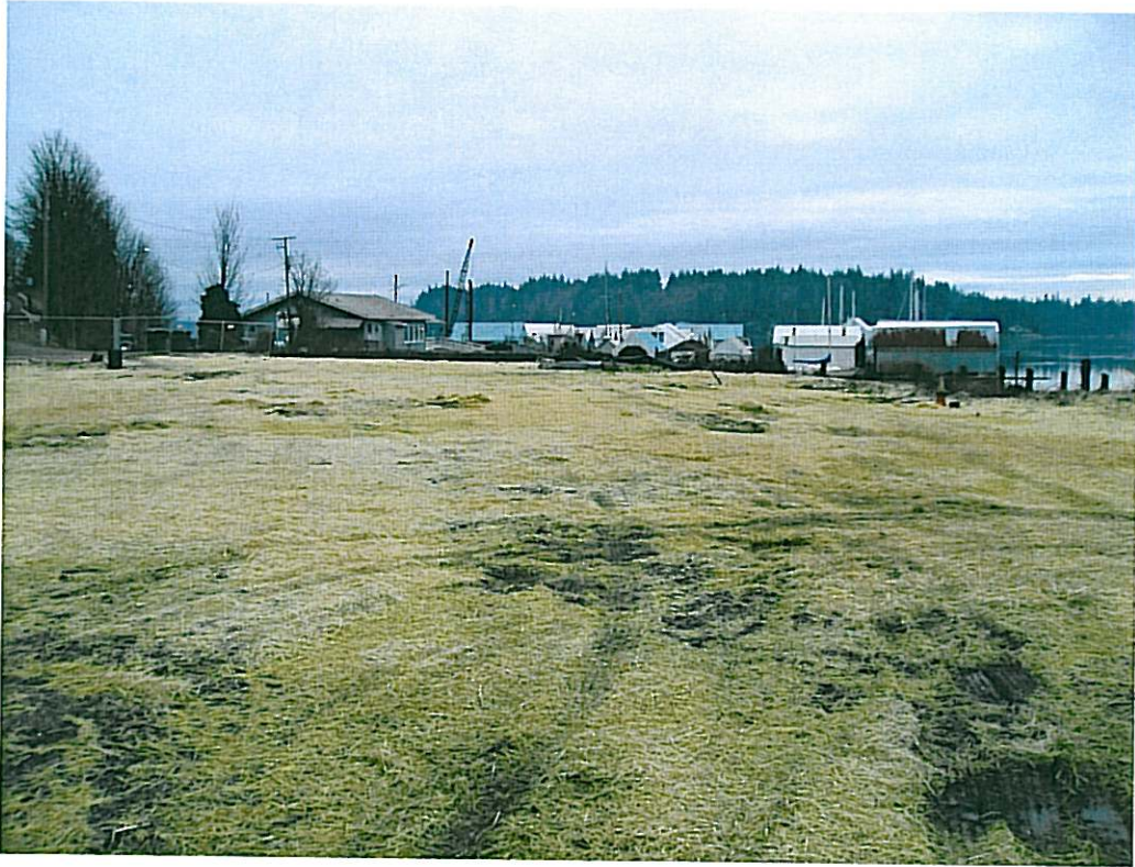
Photograph 1: Surface stabilization with straw.
