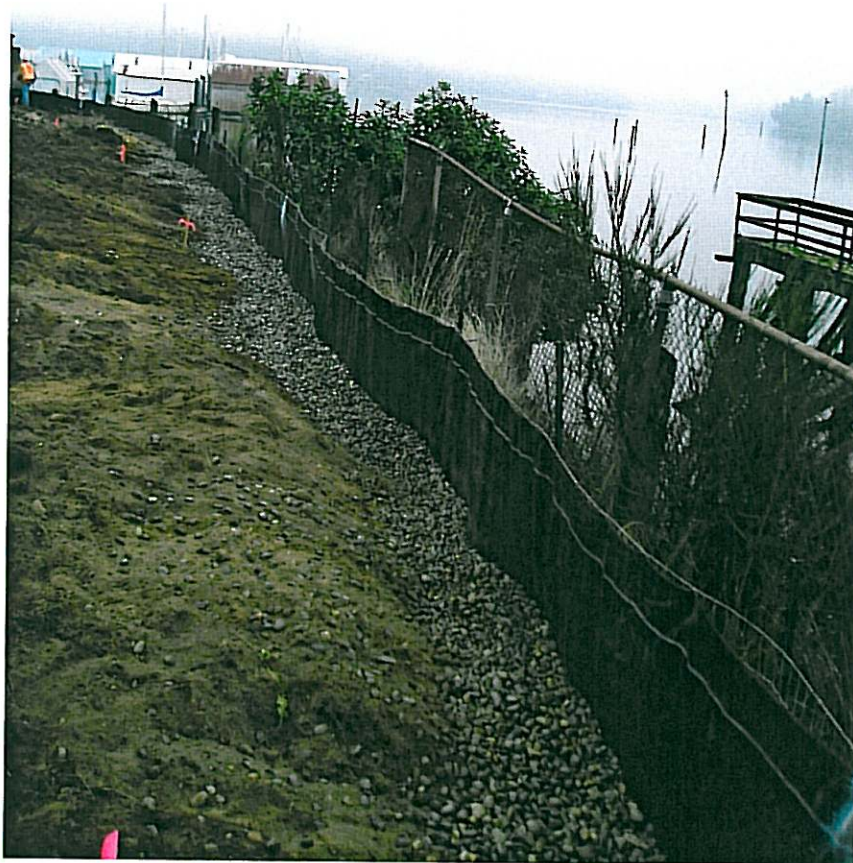
Photograph 3: Erosion control – Silt fence.
