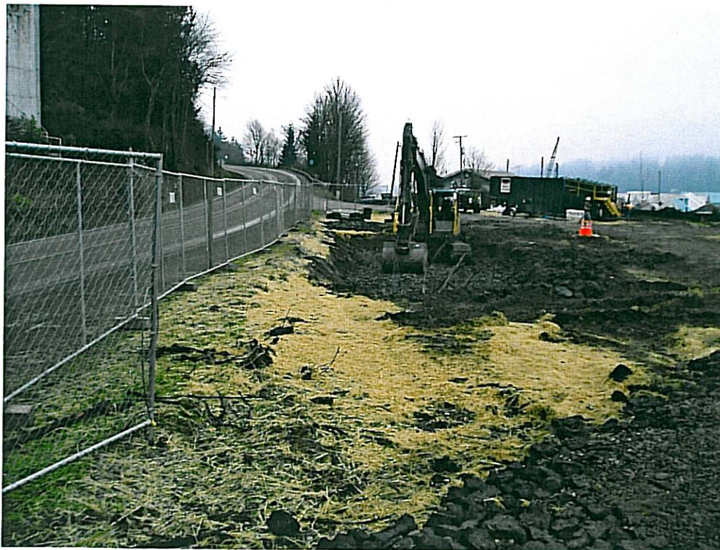
Photograph 7: Excavation and backfill along State Route 3.
