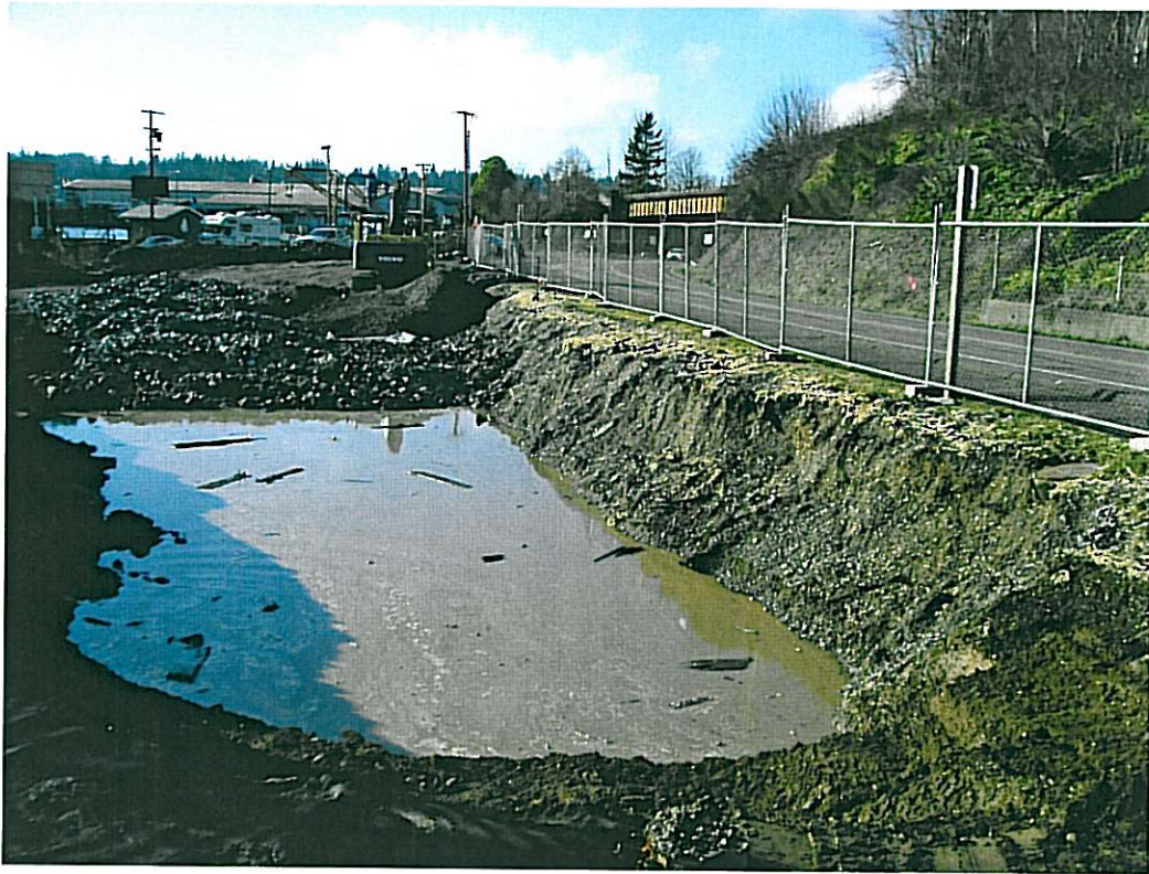
Photograph 12: Excavation along State Route 3.
