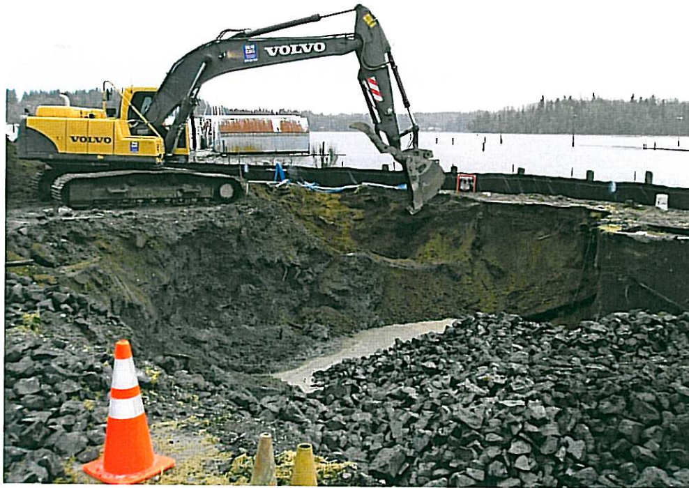
Photograph 8: Excavation on southeast portion of the Site.
