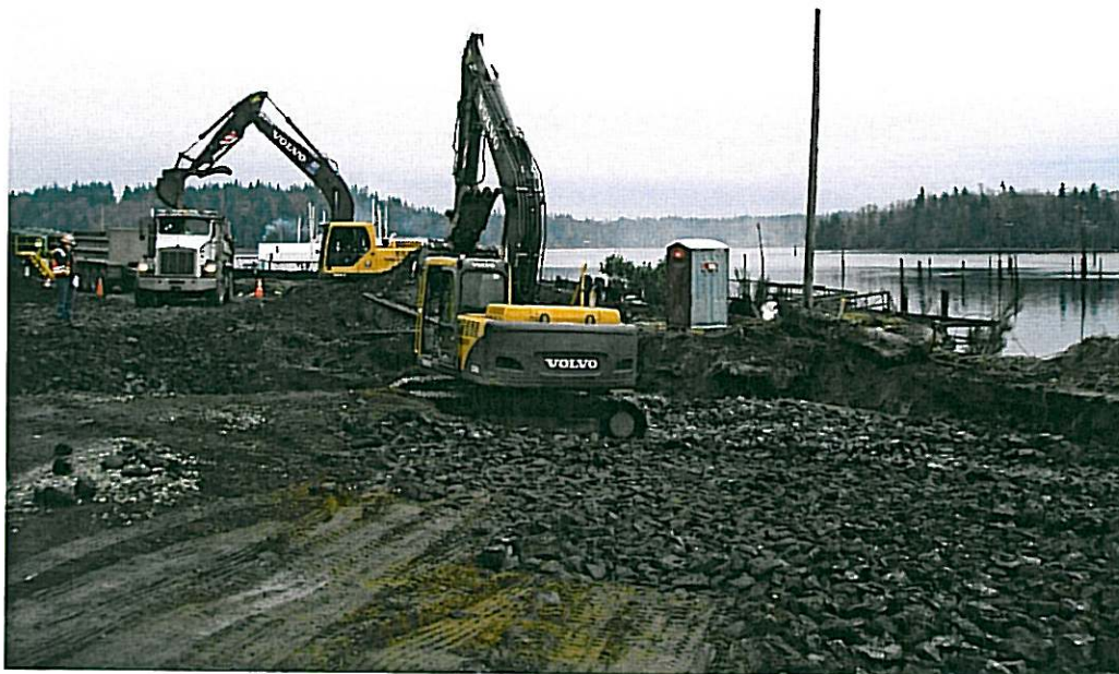
Photograph 11: Excavation on western side of the Site.
