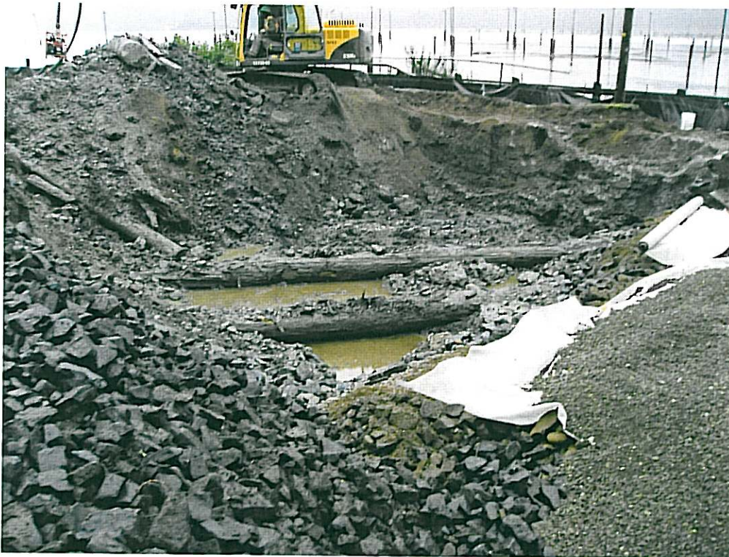
Photograph 14: Backfill showing quarry spalls, filter fabric, and crushed rock.
