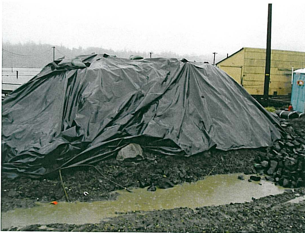
Photograph 6: Stockpile stabilization.
