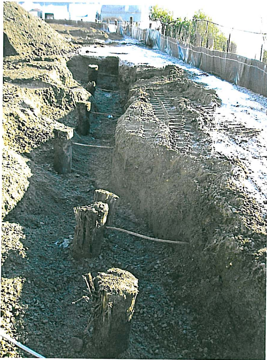
Photograph 16: Earth piles A.
