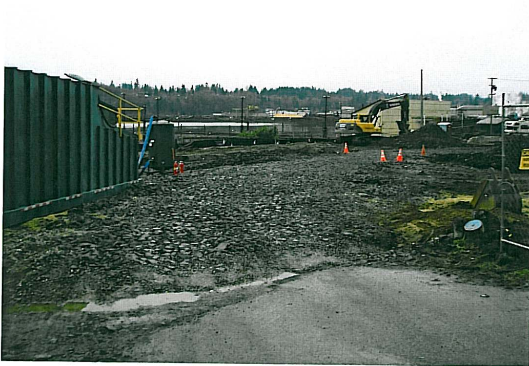
Photograph 2: Gravel construction entrance.
