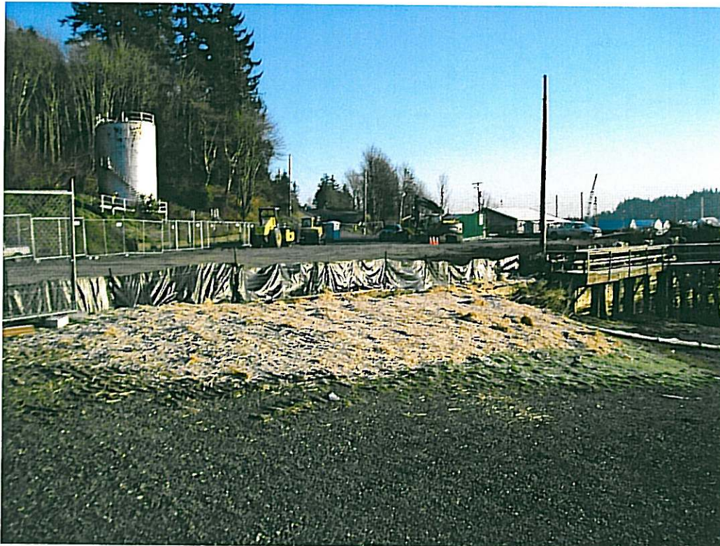
Photograph 21: Site restoration and surface stabilization.
