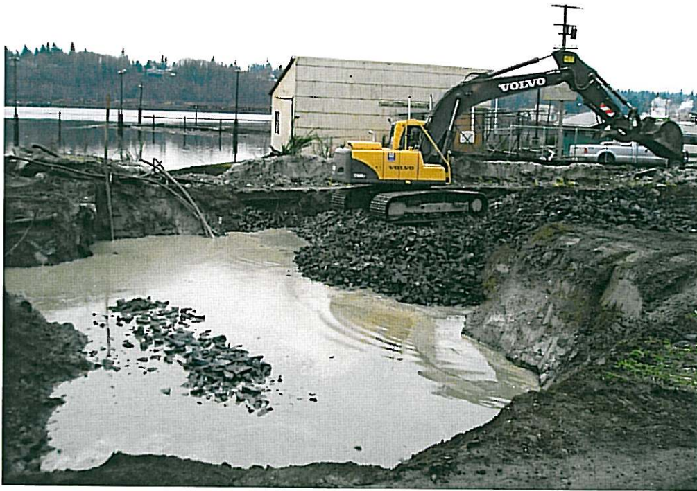
Photograph 10: Excavation on southwest side of the Site.
