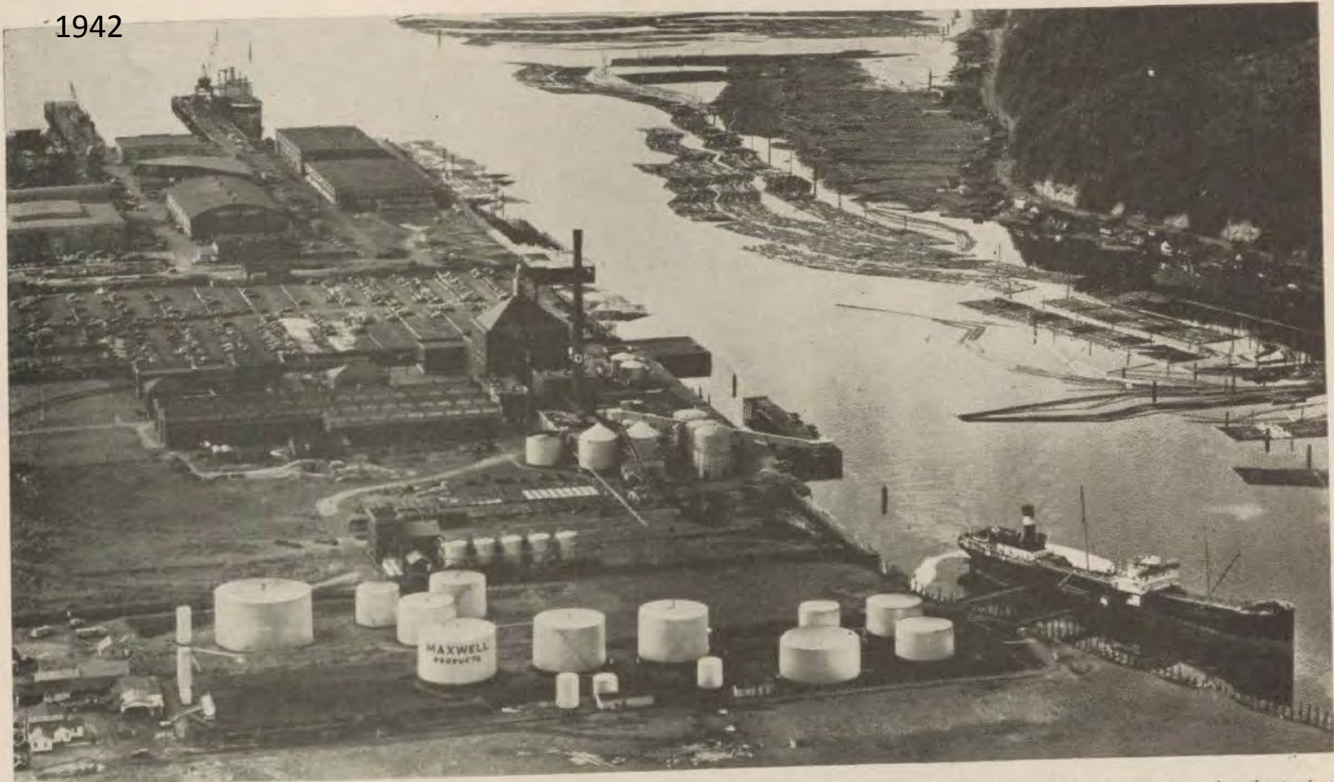
In the foreground is the 5,000,000-gal. terminal of the Maxwell Petroleum Corp., Independent oil marketer, on one of tributaries to Puget Sound, at Tacoma, Wash. A tanker from Los Angeles is discharging a load. The 5 vertical tanks immediately in the rear of the Maxwell plant, are the terminal of Fletcher Oil Co., an Independent marketer of Idaho, which supplies its business in eastern Washington from this depot. Log rafts shown on the opposite side of the stream, are a familiar sight in this territory
