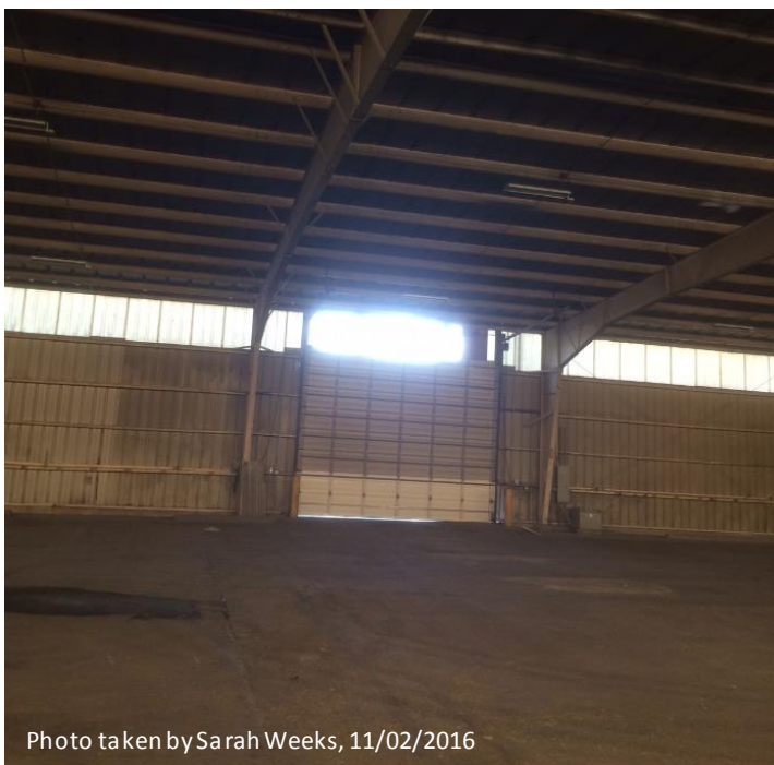
Figure 2. Missing panels above northwest garage door, looking northwest.
