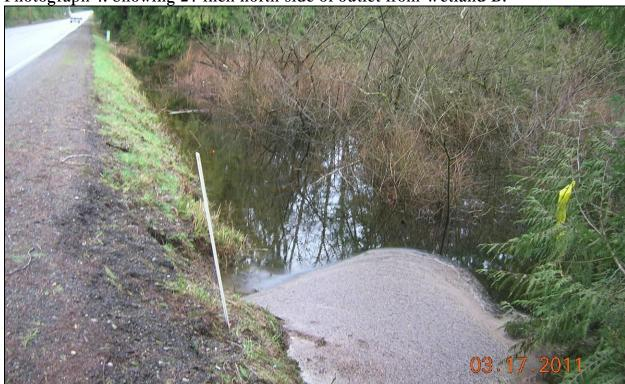
Photograph 5: Showing 24-inch outlet from Wetland B, south side of Seabeck
