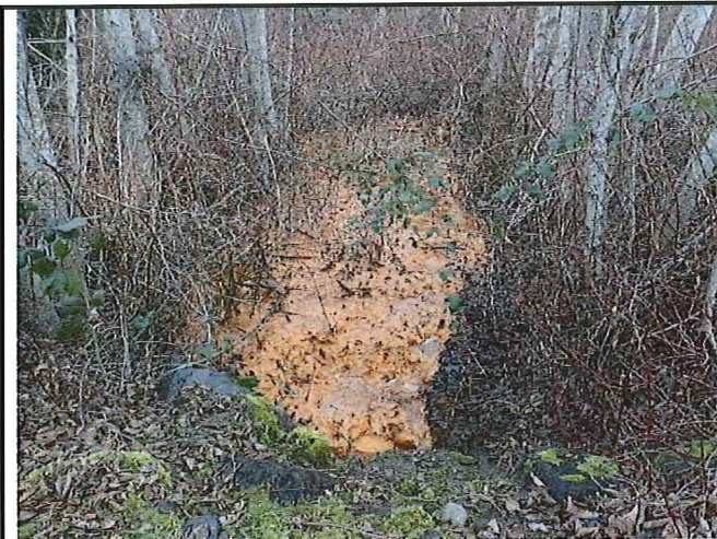
Photo #3: Orange residue flowed from the drainage ditch (north of 9th Pl W), entered the culvert, and drained to the native growth protection area (south of 9th Pl W) shown here on 2/1/2018 [P1310068.JPG].
