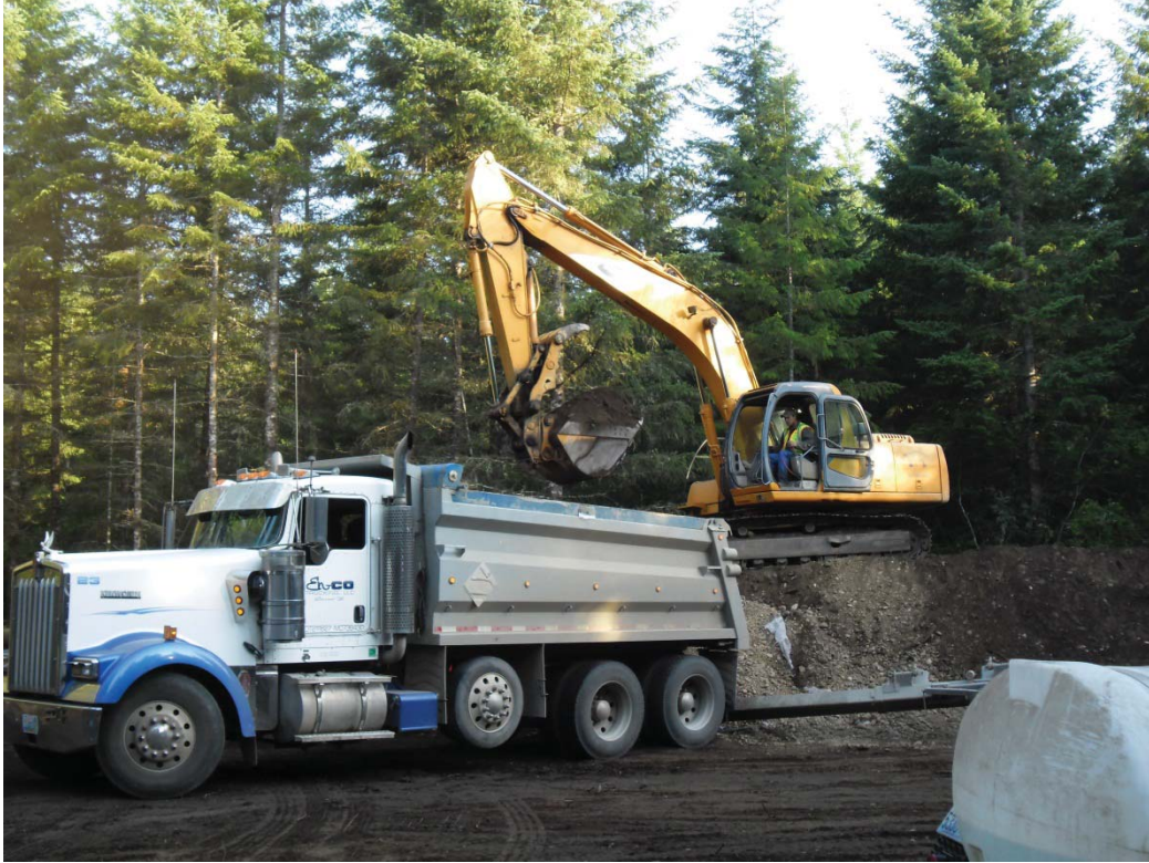
3. Loading out Bordeaux Dump excavated material.
