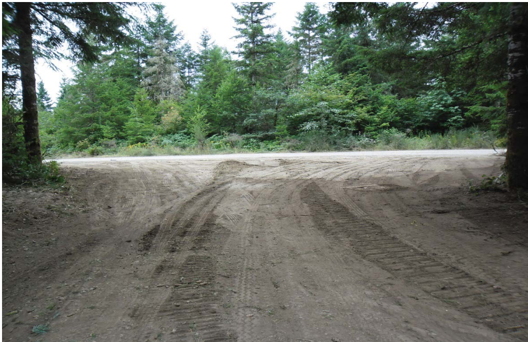
2. Entrance to Bordeaux Dump staging area and laydown yard.
