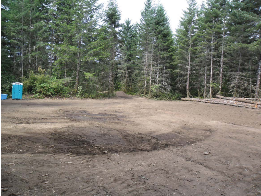
5. Bordeaux Dump stockpile yard cleared.
