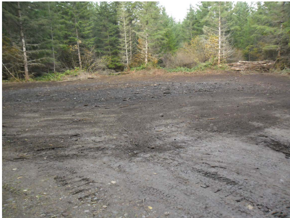
8. Bordeaux Dump staging area and laydown yard graded and reseeded.
