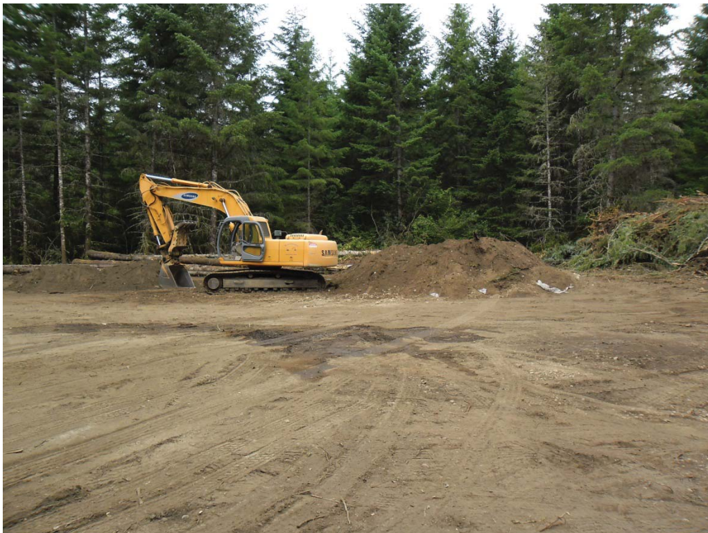
4. Bordeaux Dump stockpile greatly reduced.
