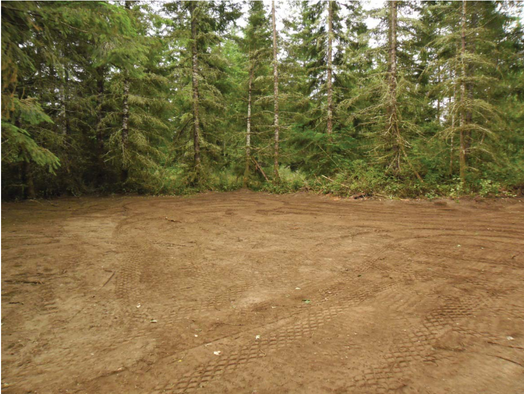
6. Bordeaux Dump excavation backfilled and with topsoil spread and rolled.
