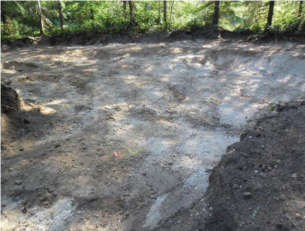
1. Bordeaux Dump area excavation with compliance sample locations.
