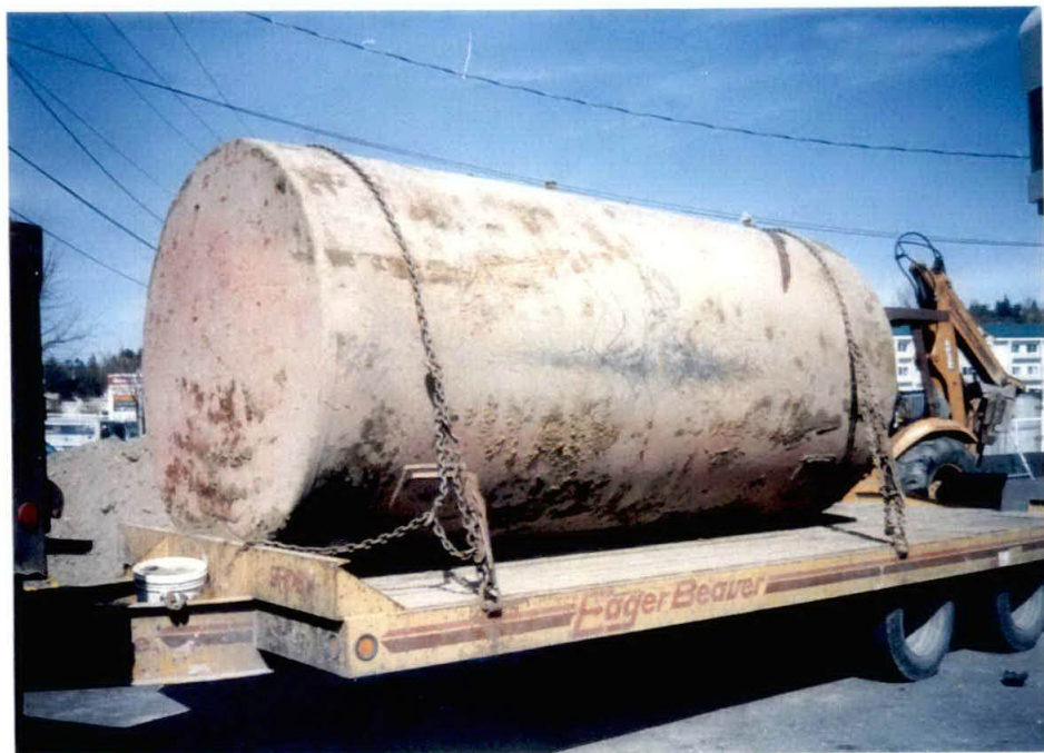
Removed 3,000 gallon UST in good condition.
