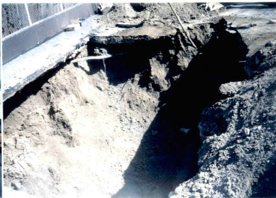
UST excavation, no soil contamination.
