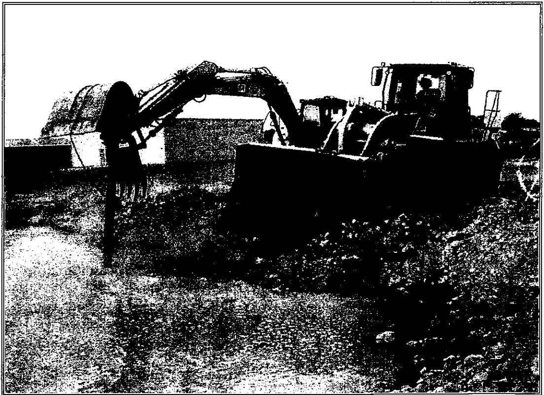
Backfilling of RegenOx ® treated 2008 excavation – July 2008.
