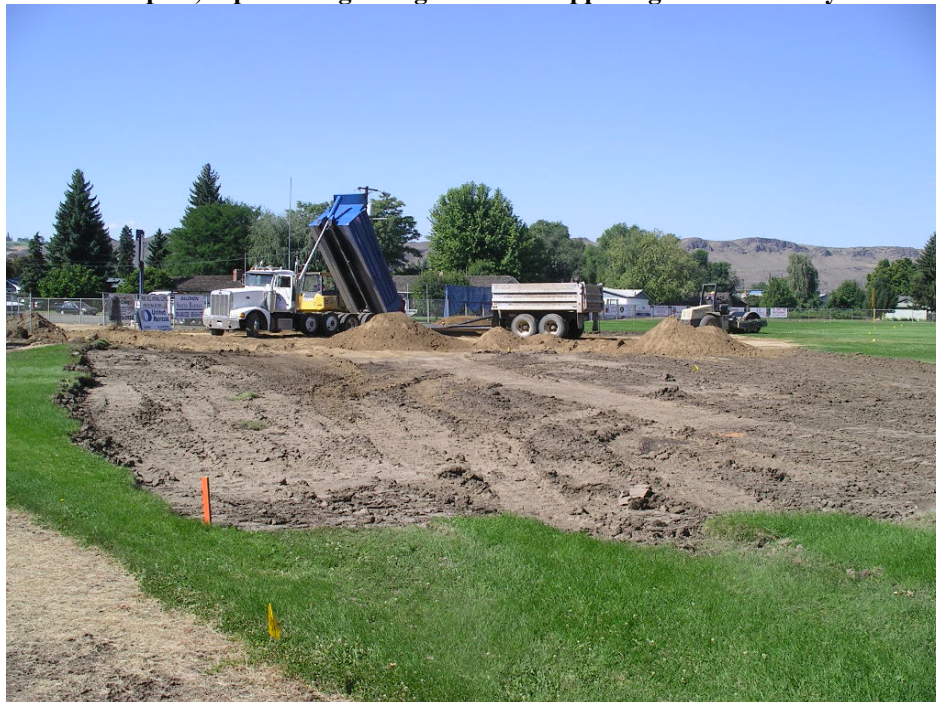
Photo D-3 Hotspot excavation and backfill at the baseball field
