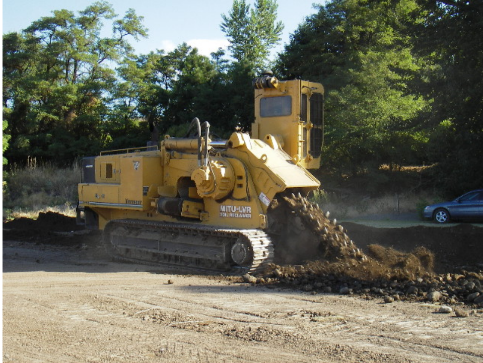
Photo D-1 Deep mixer in action at Naches Intermediate
