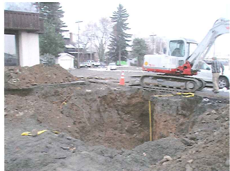
Yellow flagging tape used to mark the excavation extents prior to backfilling.
