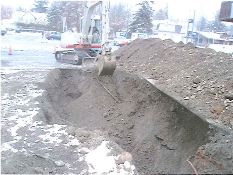
Sloughing soils undermining asphalt and concrete along the east boundary of the excavation
