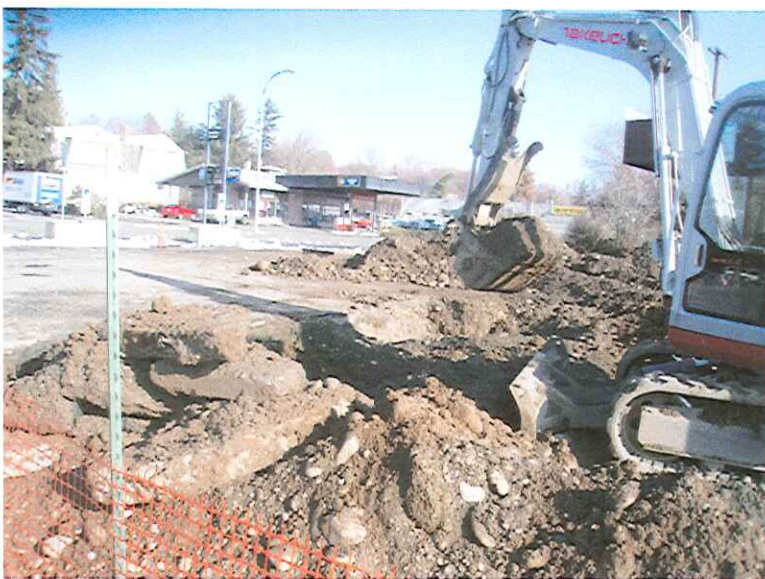
Backfilling of site soils neat the southwest portion of the excavated area.
