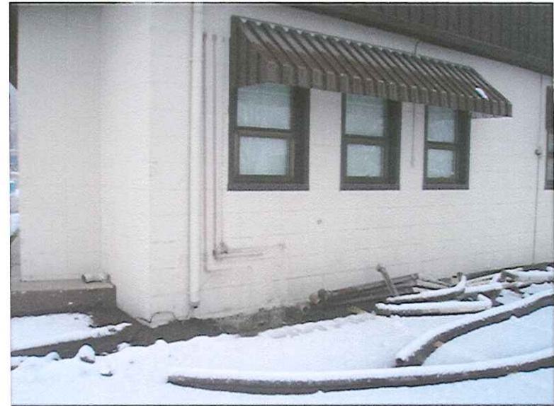
Southwest corner of the site building with remnant UST vent piping.
