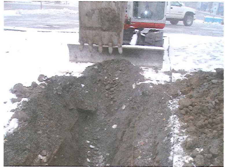
Excavation of imported backfill in the east trench of the excavation.
