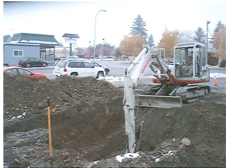
Excavation activities near the north center of the former UST basin.
