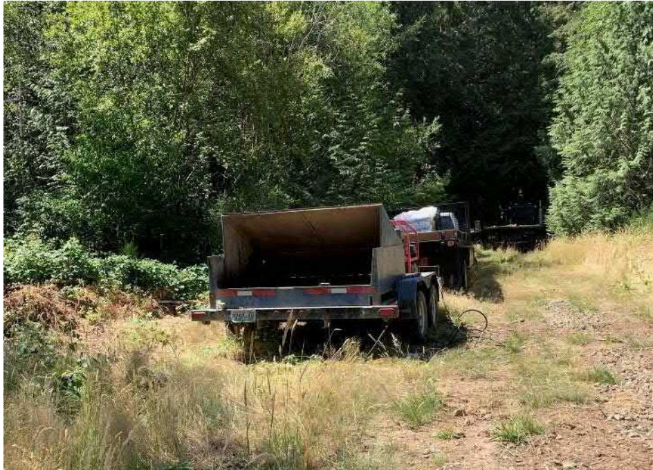
Photo 9: 7-13-21 Monitoring Well Installation – Showing the decontamination equipment set up.
