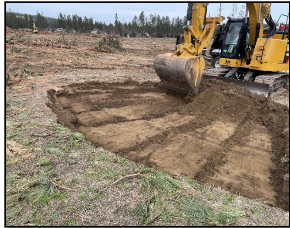
View of typical remedial excavation conducted for the mercury impacted onsite putting greens.
