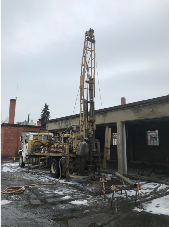
Installation of MW-5 by Broom Shed
