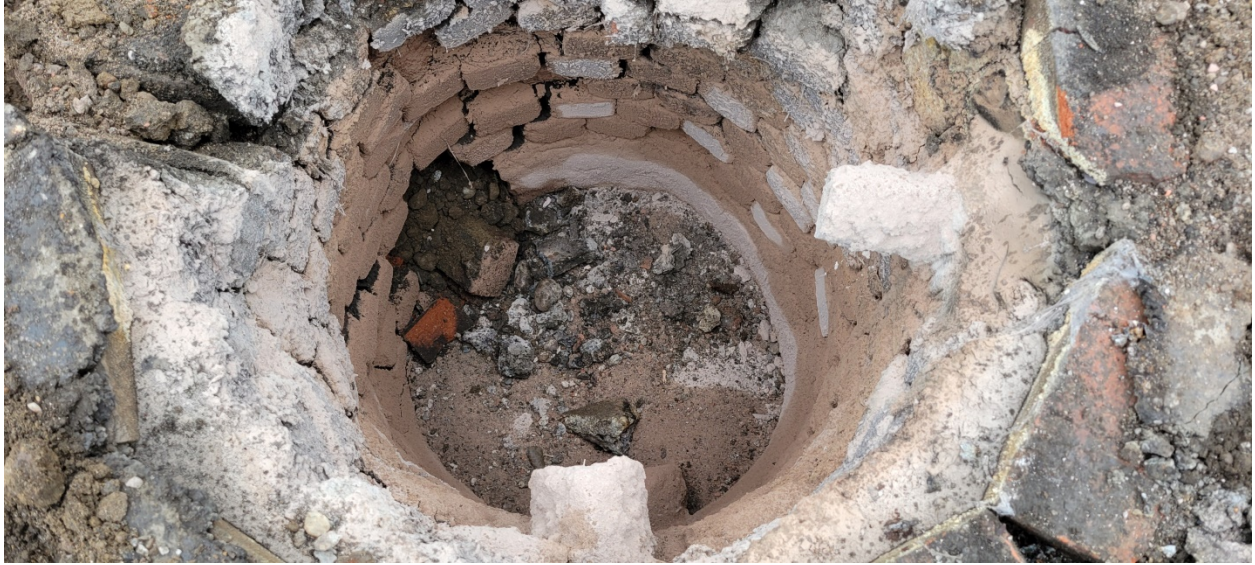
Inside old cesspool at Broom Shed building, May 2021
