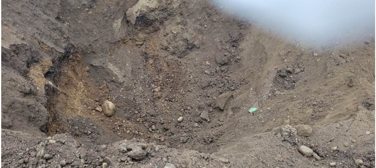
Soils below the cesspool after removal, May 2021
