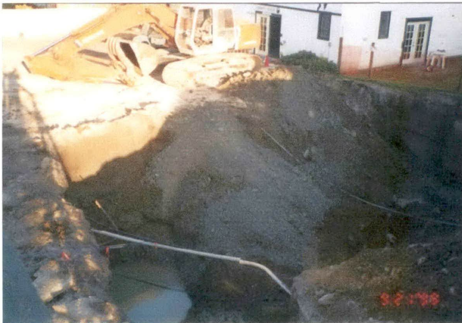
Figure 6. View of excavation from the patio of the Recreation Center. Ground water was observed on the south end of the excavation.
