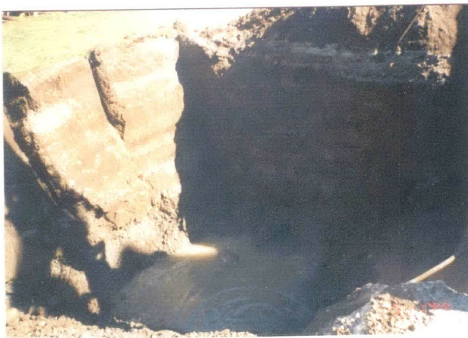
Figure 3. Photograph of north end of the excavation. Tank was located on the left side of the photograph. Ground water was observed at a depth of approximately 11.5 feet.
