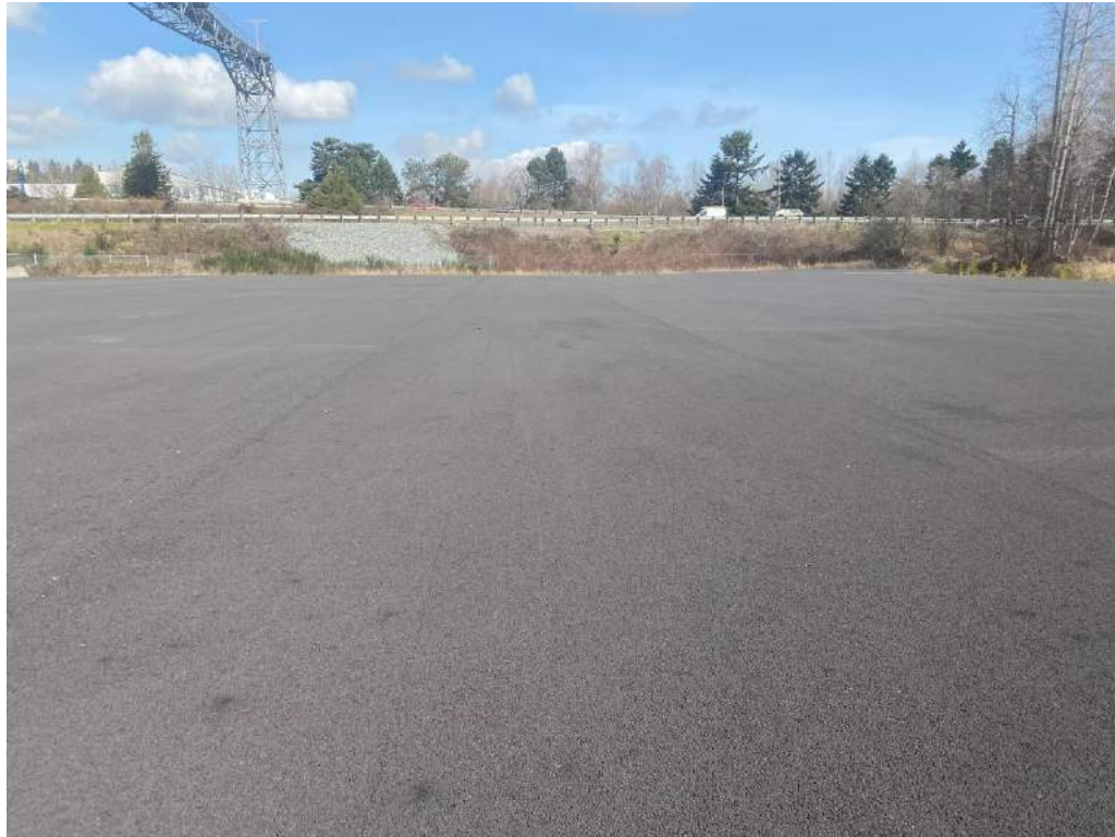
Photograph 9. Good cap conditions at stations DMCA 11 and DMCA 13 captured from the southeast corner of the DMCA.
