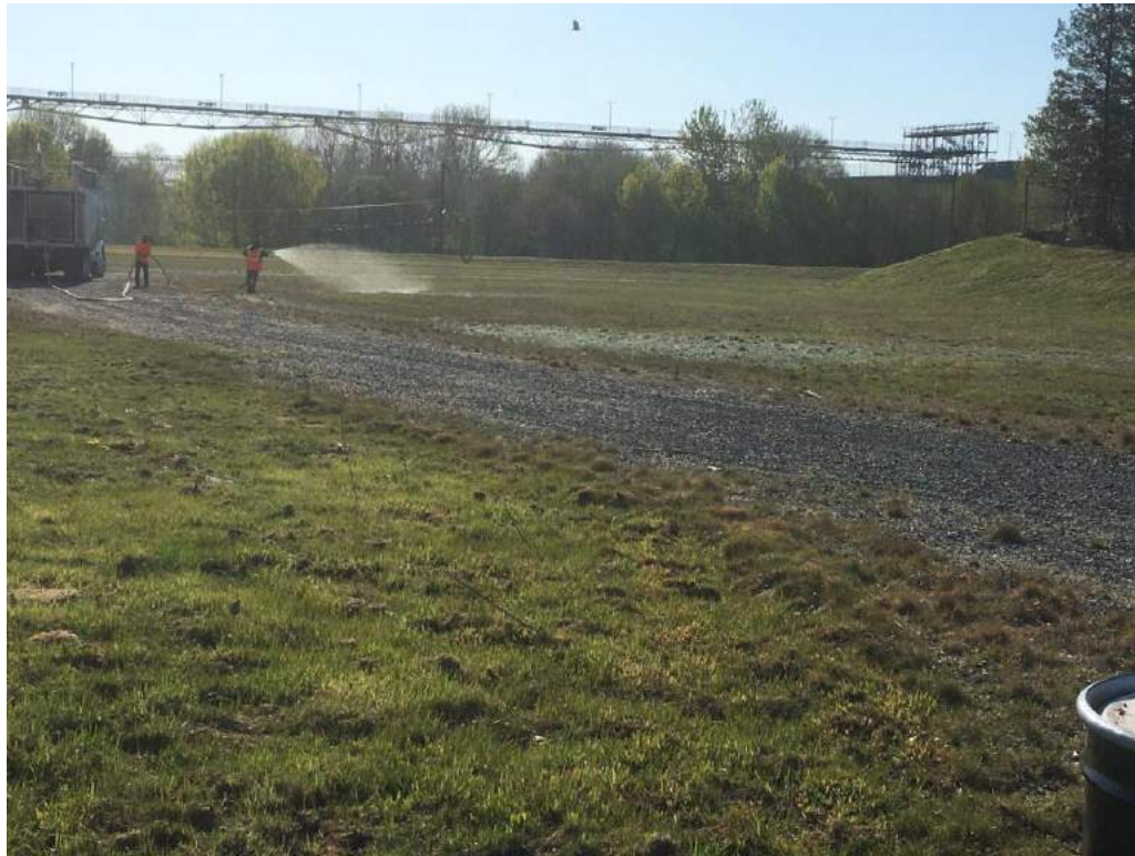
Photograph 1. Lora Lake Apartment parcel reseeding to address loss of barrier material.
