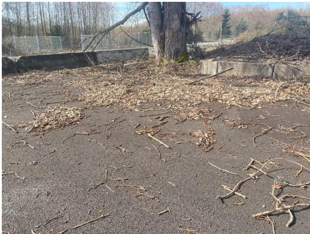
Photograph 8. Area underneath large tree, near station DMCA 09, requiring removal of debris.
