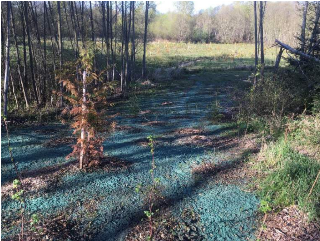
Photograph 3. Hydroseeding to restore Lora Lake temporary access road footprint.
