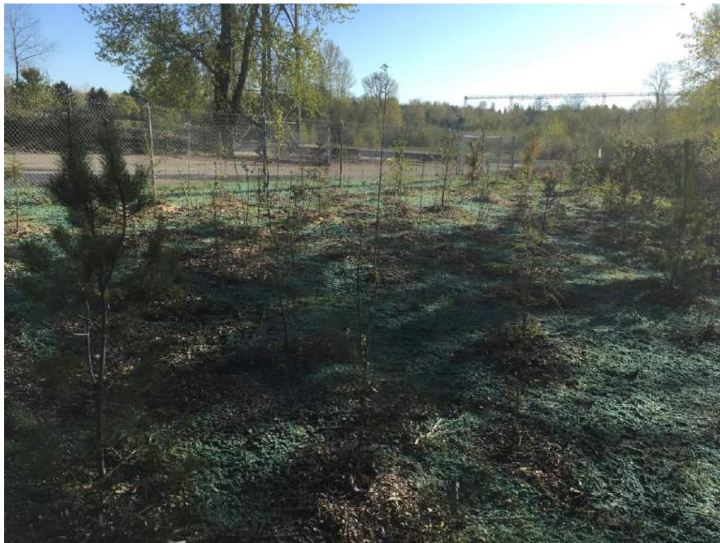
Photograph 2. Hydroseeding near Lora Lake.
