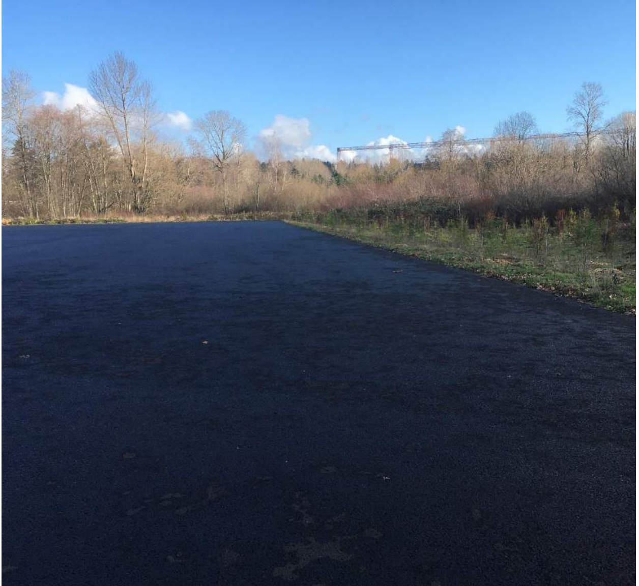
Photograph 7. Southern edge of the DMCA after removal of excess debris.
