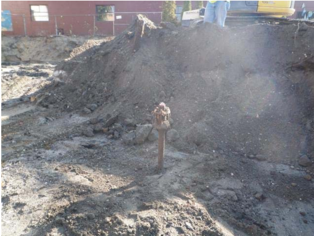
Photograph 9: Apparent water supply well encountered during excavation activities (east-central property area)
