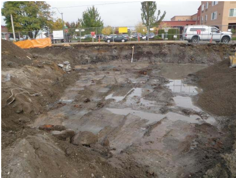
Photograph 2: Typical subsurface excavation conditions
