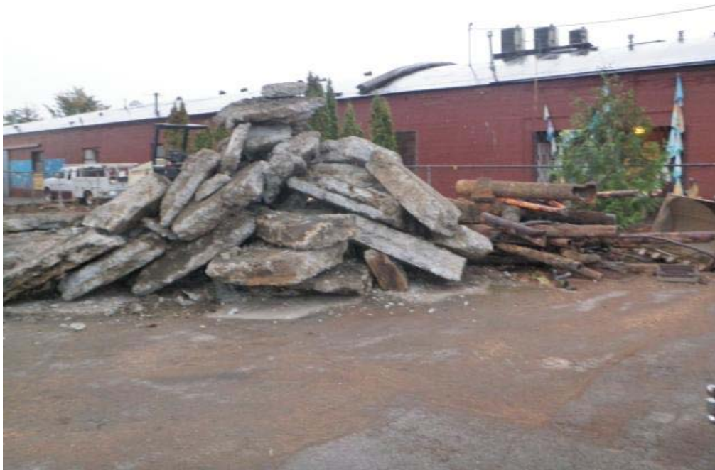
Photograph 6: Concrete footing/foundation and piping debris removed from excavation
