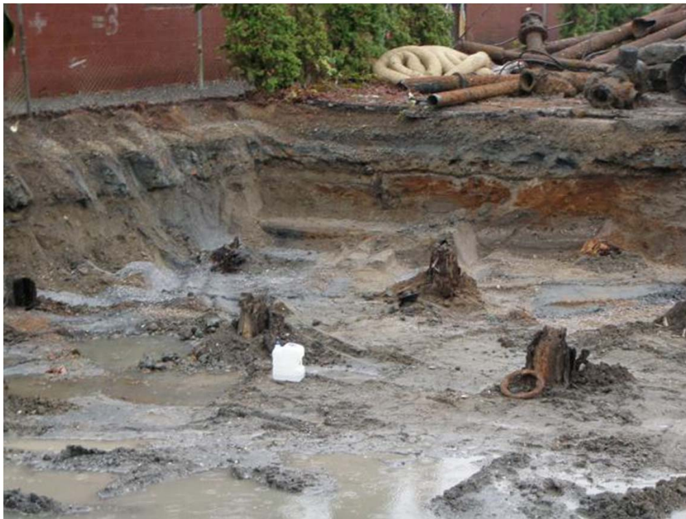
Photograph 8: Unpreserved wood piles (south-central area of property))
