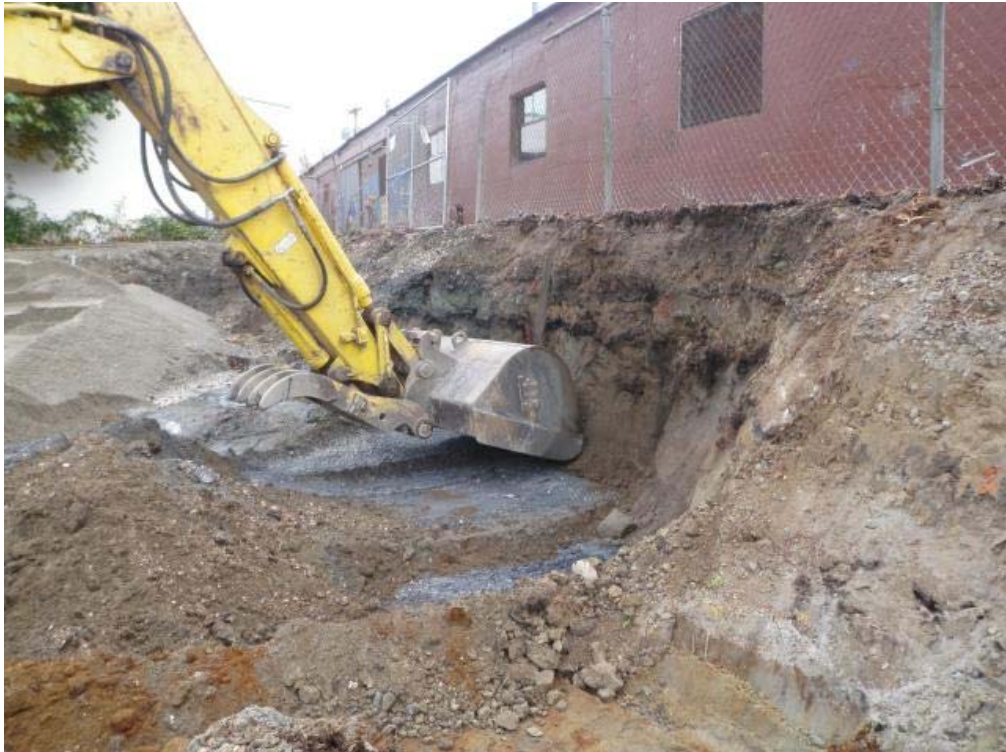
Photograph 3: Excavation sidewall vertical cut activities
