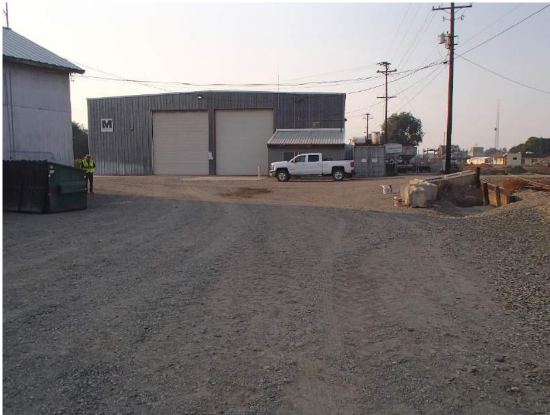
Photograph 9. Machine shop and area behind office building (looking north). August 2017.
