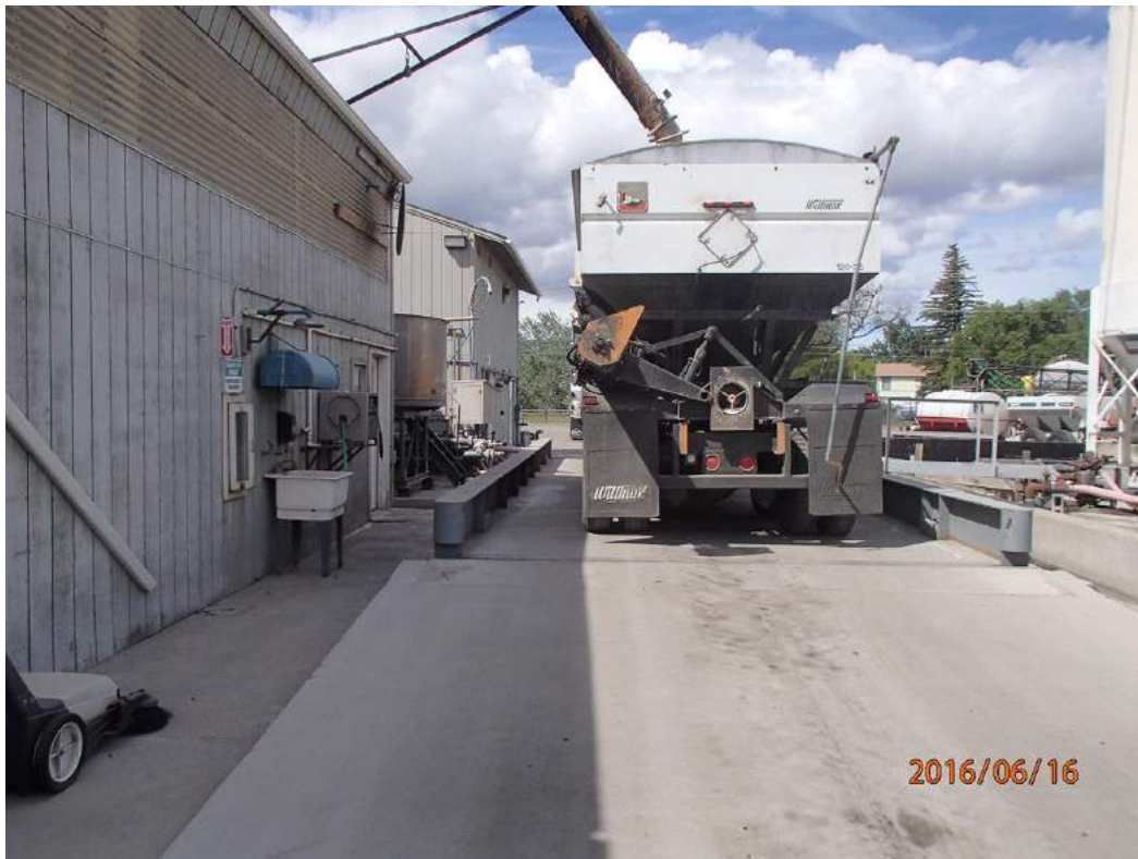
Photograph 5. Scale/truck filling area between bulk fertilizer building and AST containment area (looking west). June 2016.
