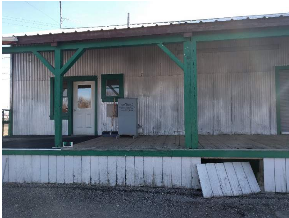
Photograph 1. Crawl space beneath the office building, looking east.
