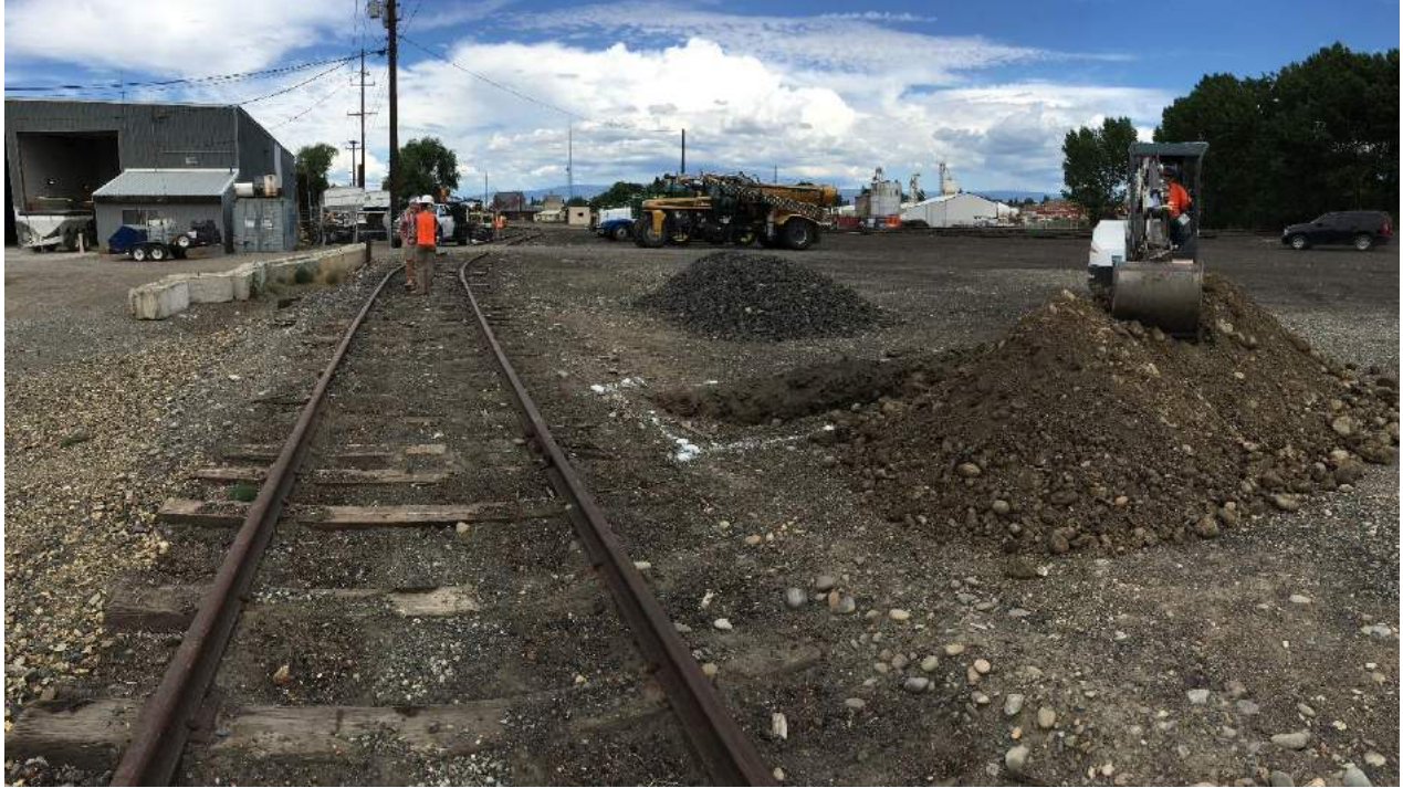
Photograph 21. Location of TP-1 adjacent to rail spur (looking north). June 2018.
