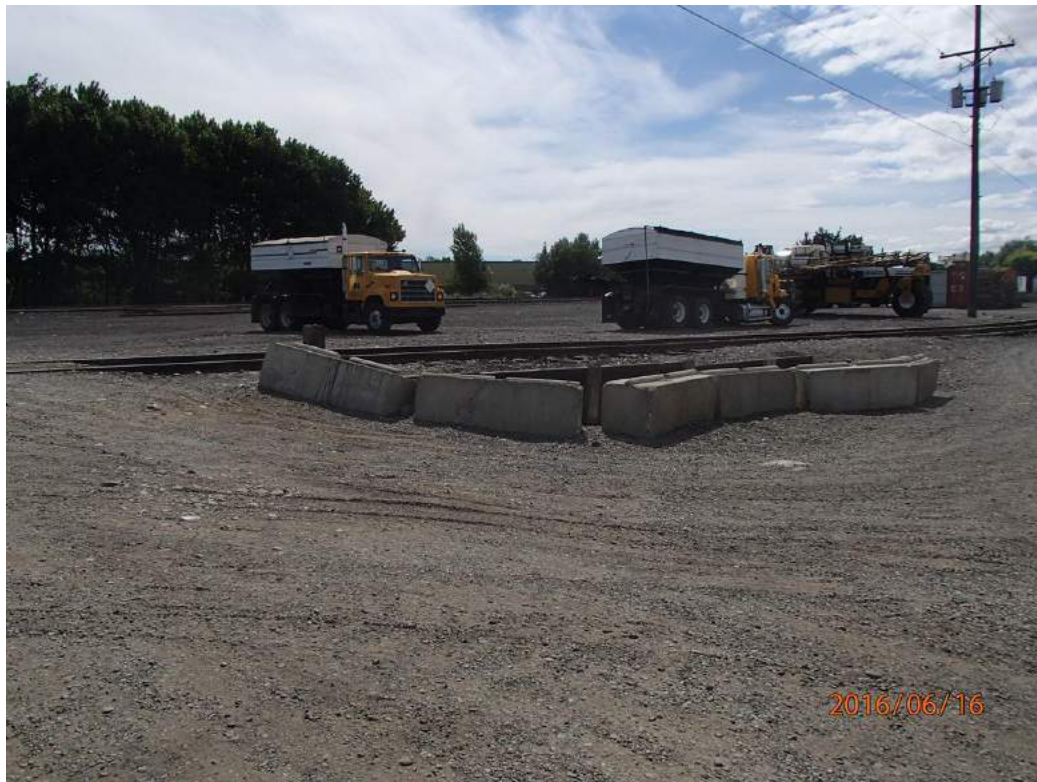
Photograph 12. Low spot near monitoring well MW-4 (looking southeast). June 2016.
