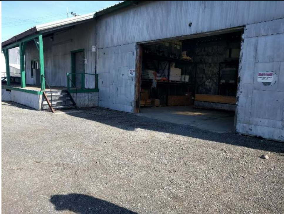
Photograph 1. Chemical storage area adjacent to office building (looking northeast). February 2016.
