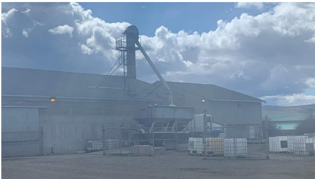
Photograph 6. Dust blowing off truck as it is being filled with dry fertilizer product. March 2020.
