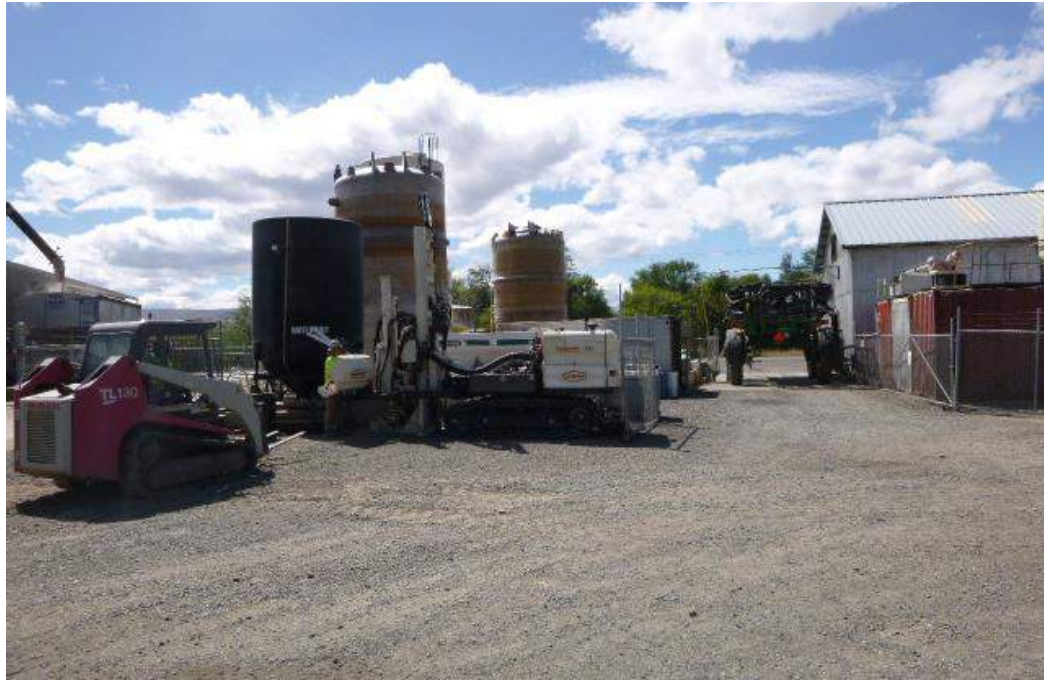
Photograph 7. AST containment area (during installation of MW-11; looking west). August 2016.
