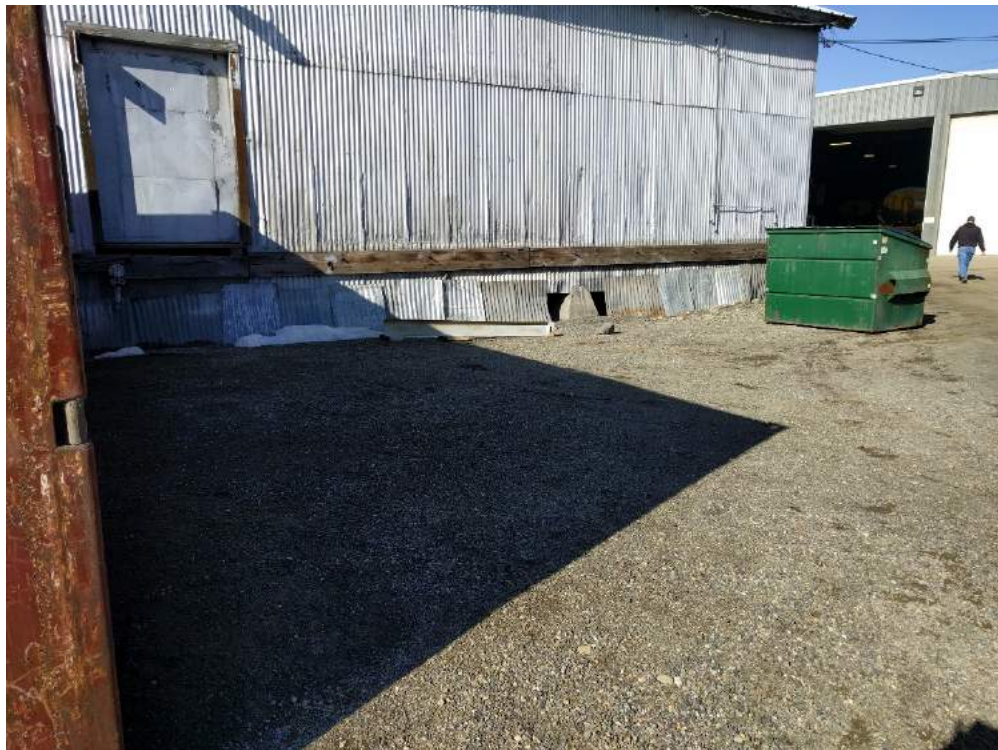
Photograph 2. Crawl space behind office building with dumpster for scale, looking northwest.
