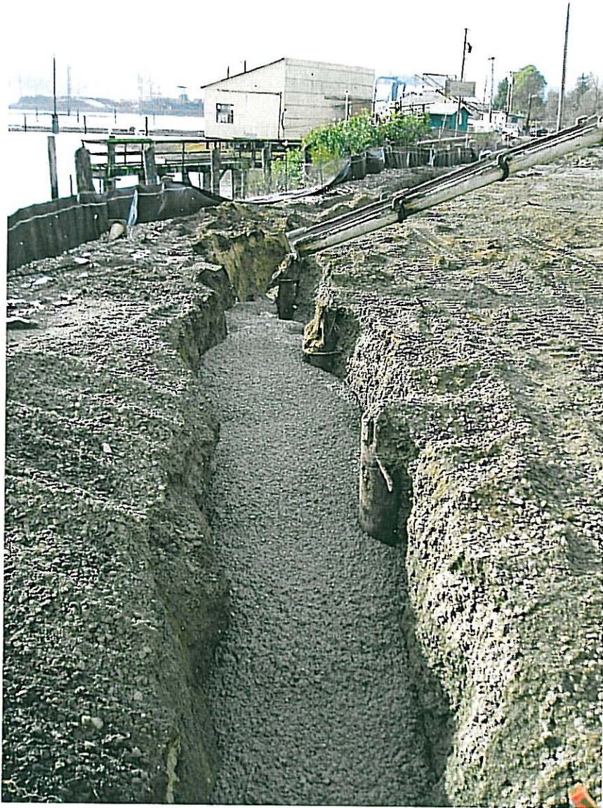
Photograph 17: Emplacement of concrete earth anchors.
