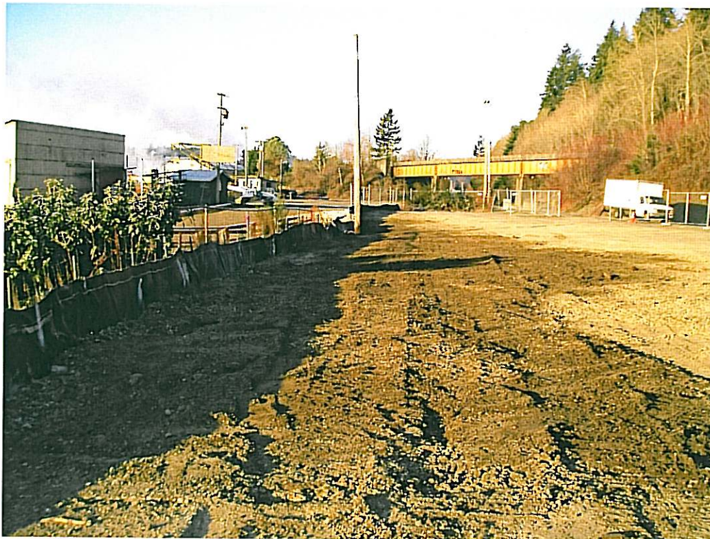
Photograph 19: Backfill and compaction.
