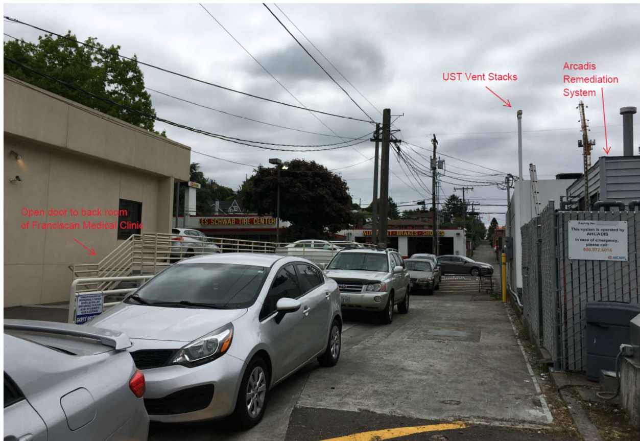
Photo 1: Alleyway between the UST facility (UST ID# 10140) and the Franciscan Medical Clinic
