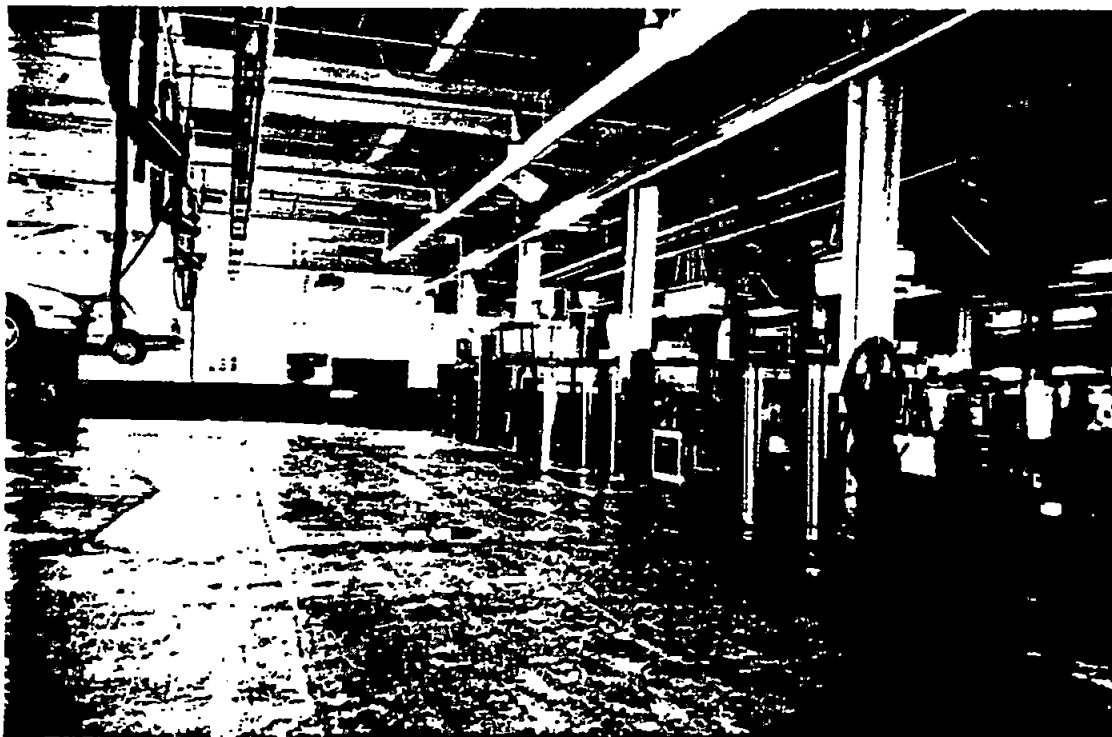
Photo 2 Hydraulic lifts in middle of building, look southwest.
