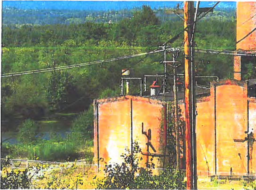
Mill Pond and powerhouse
