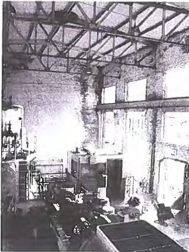
Turbine Room Interior
