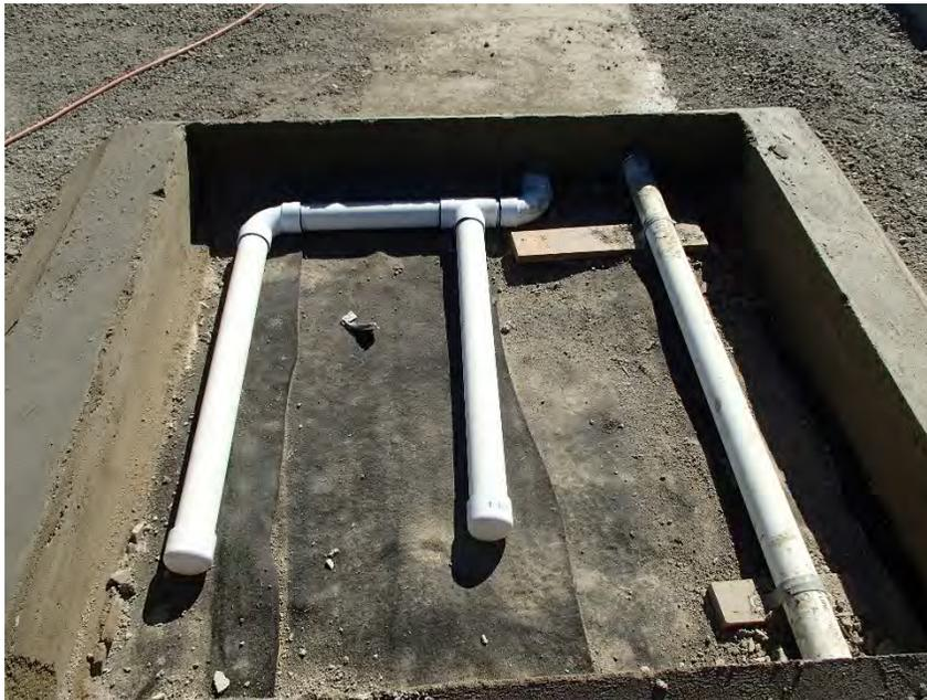
Photograph 9 Final pipe layout in Cell 5-A
