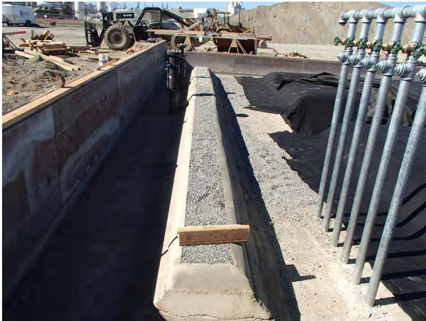
Photograph 12 Gravel backfill and bottom layer of geofabric
