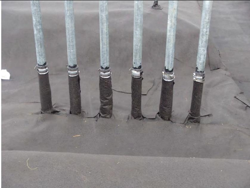
Photograph 21 Manifold top geofabric layer
