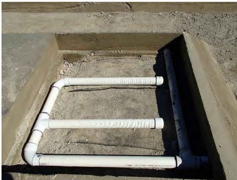
Photograph 10 Final pipe layout in Cell 4-AA
