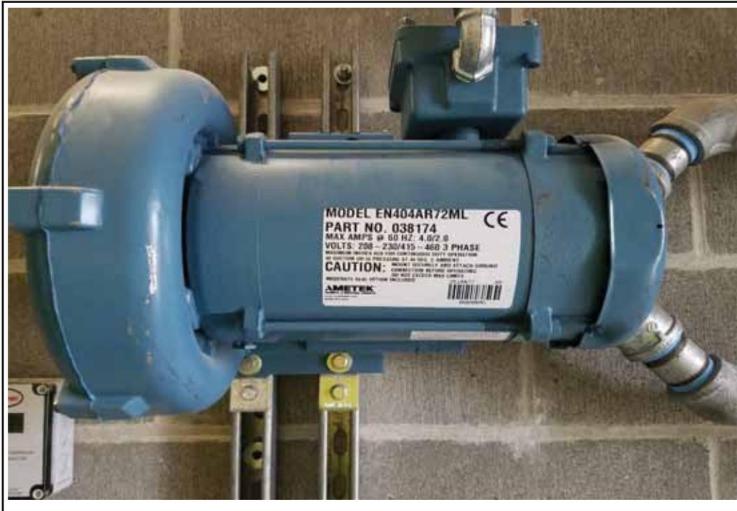
Photo 13: View of the Ametek Rotron EN404AR72ML regenerative blower that induces the vacuum and air flow from the sub-slab recover pipes.
