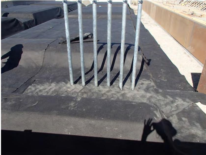
Photograph 13 Bottom layer of geofabric
