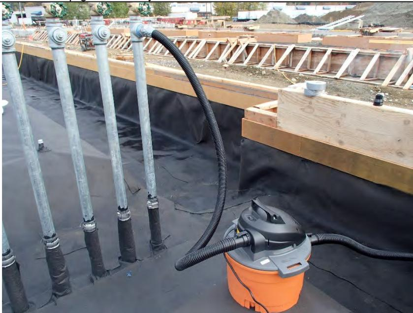
Photograph 22 Smoke testing liner
