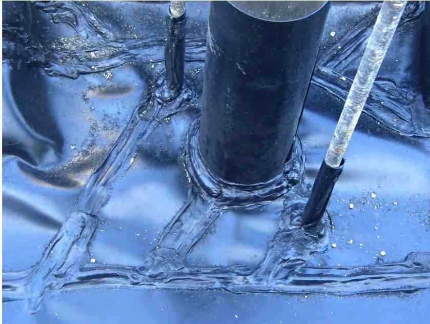
Photograph 15 Liner boot welds
