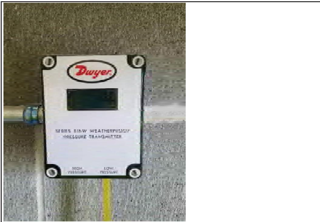
Photo 12: View of Dwyer differential pressure transmitter and screen. Transmitter reads in inches water column vacuum.
