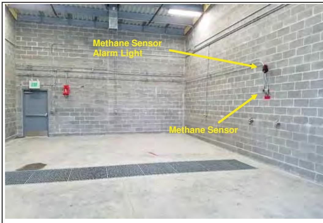
Photo 6: View of room "D" (from plans) looking to the west. Note the methane sensor and associated alarm light on the north wall (right side).
