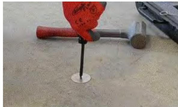
**Figure 5.** Tightening the Secured Cover.
