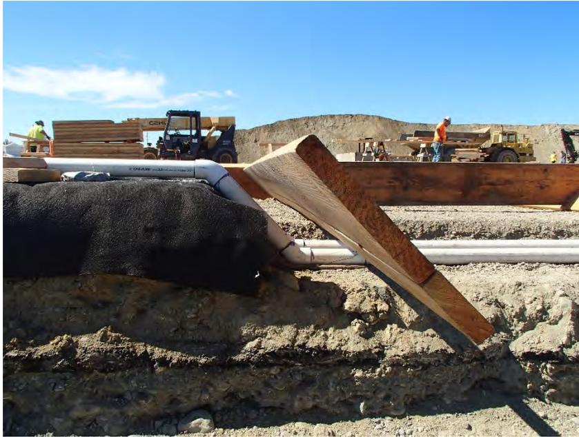
Photograph 5 Pipe crossing at future grade beam location
