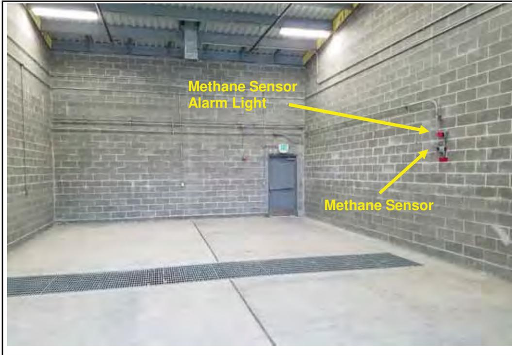
Photo 7: View of room "C" (from plans) looking to the west. Note the methane sensor and associated alarm light on the north wall (right side).
