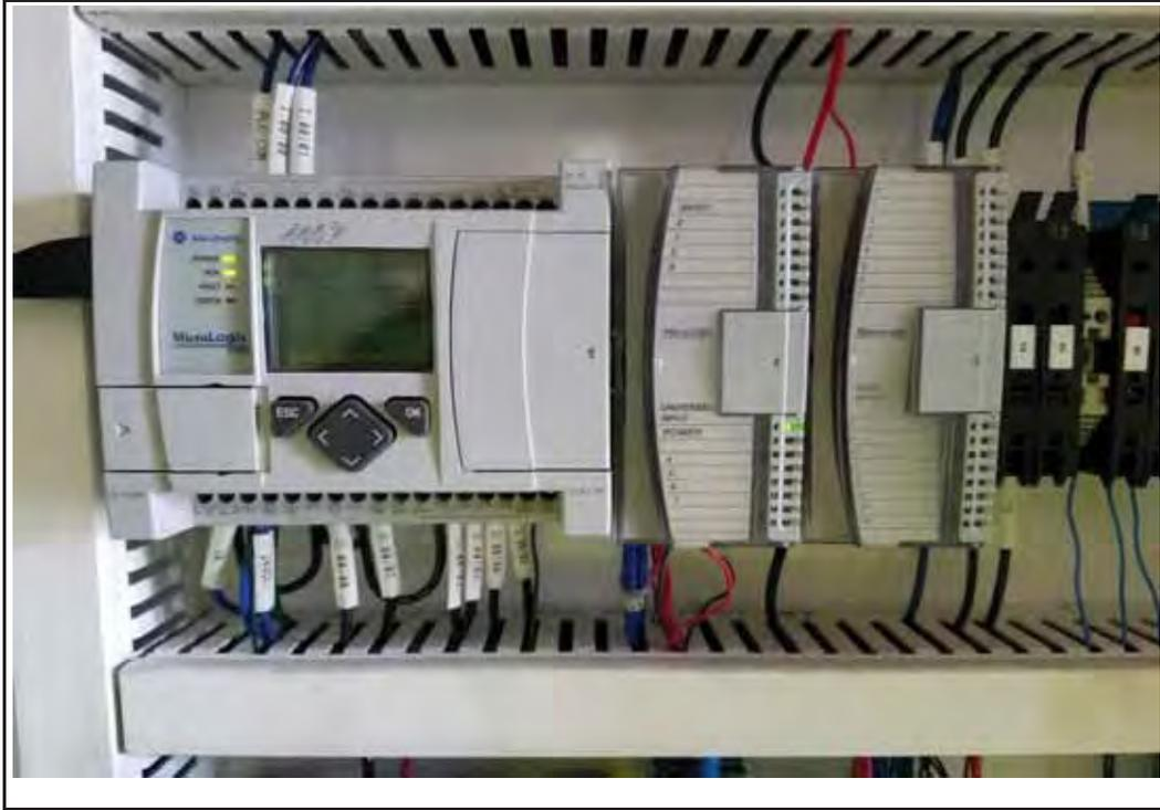
Photo 21: View of the VMS Control Panel Allen Bradley PLC unit (located in upper left of the control panel interior).
