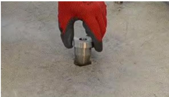
**Figure 3.** Installing the Drilling Guide.
