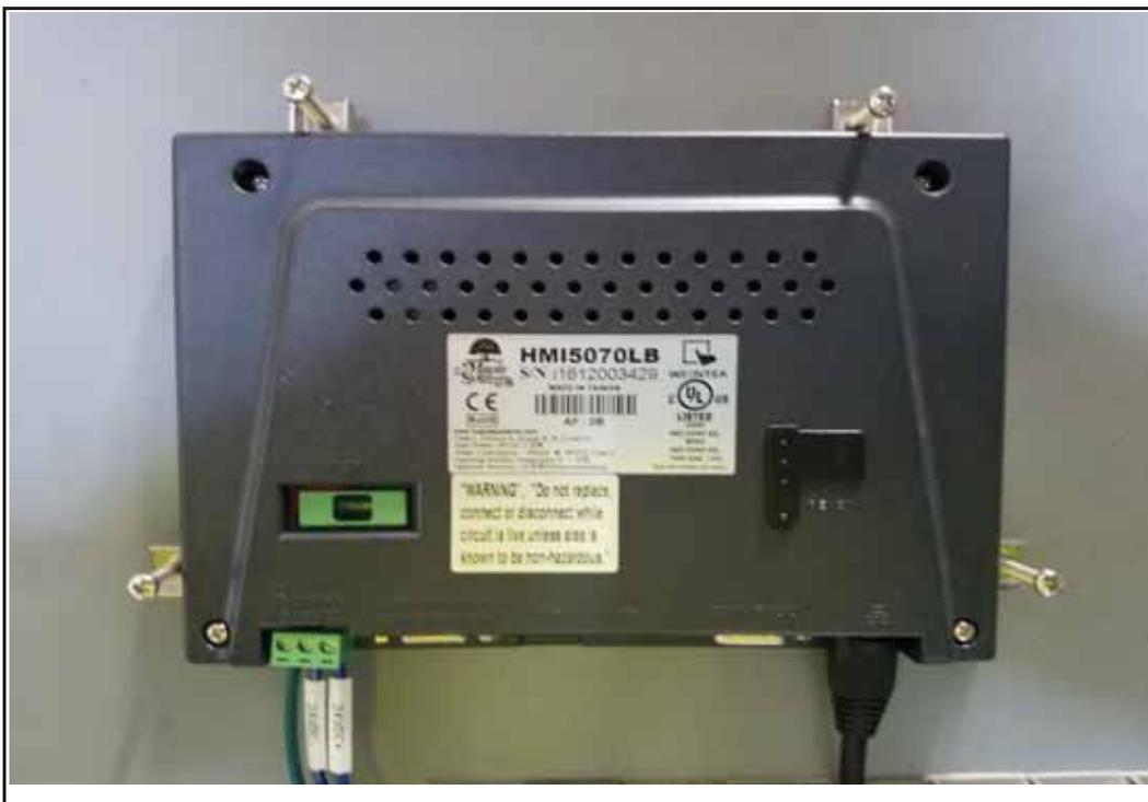
Photo 22: View of the back of the human-machine interface (touchscreen) on the back of the door panel inside the VMS Control Panel.
