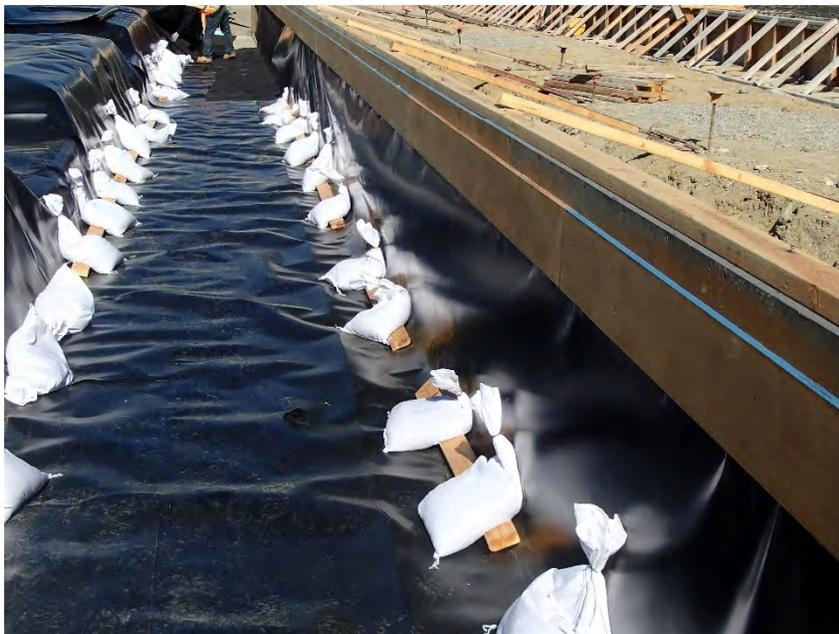
Photograph 16 Liner installation on East wall
