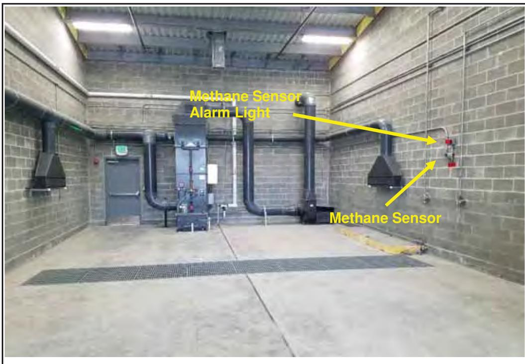
Photo 8: View of room "B" (from plans) looking to the west. Note the methane sensor and associated alarm light on the north wall (right side).
