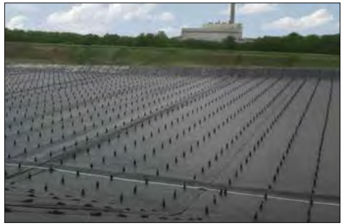
Landfill Rainshed Cover
