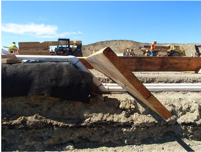
Photograph 5 Pipe crossing at future grade beam location
