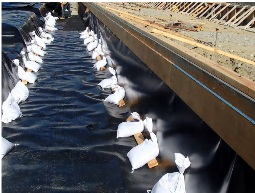
Photograph 16 Liner installation on East wall
