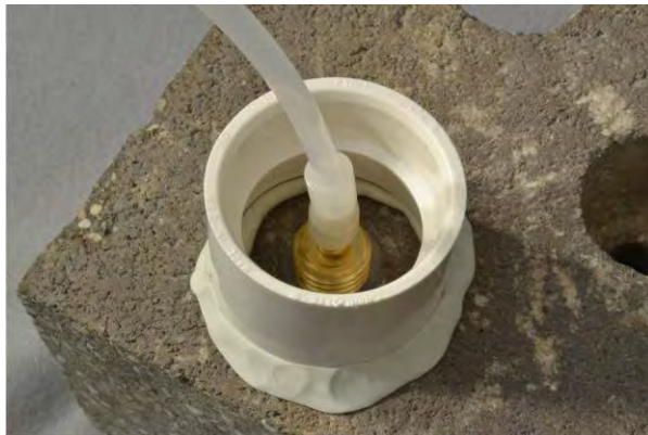
Figure 6. Water dam used for leak detection.
