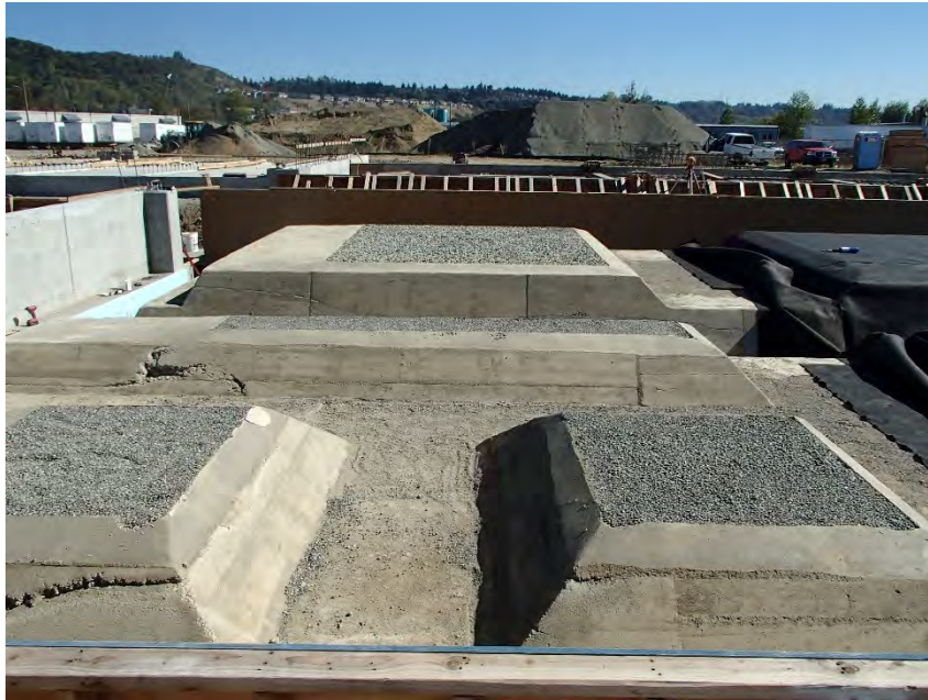
Photograph 11 Gravel backfill
