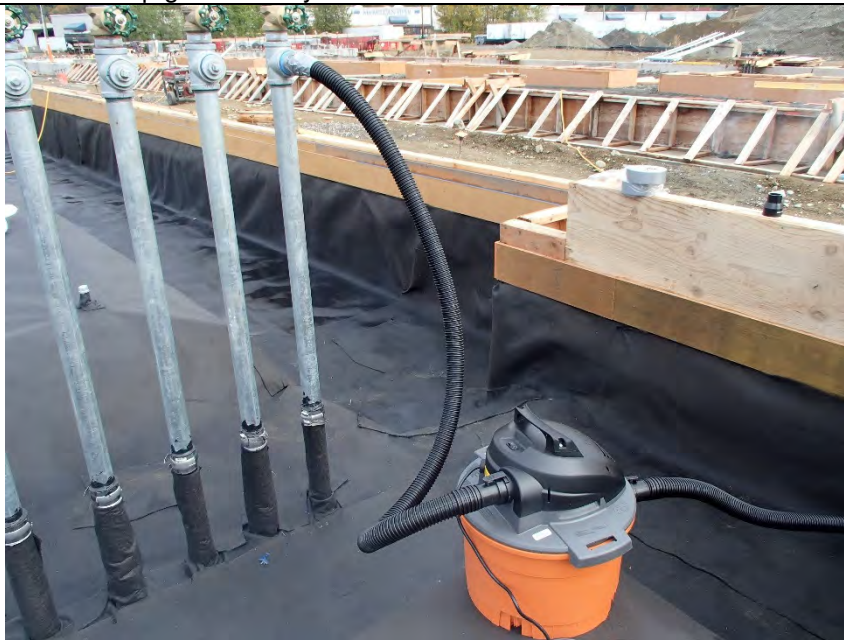
Photograph 22 Smoke testing liner
