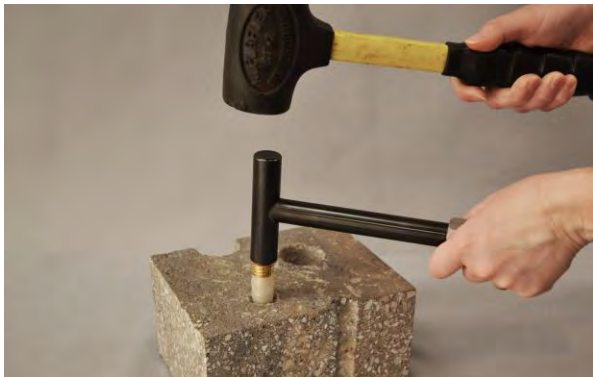
Figure 2. Installing the VAPOR PIN®
