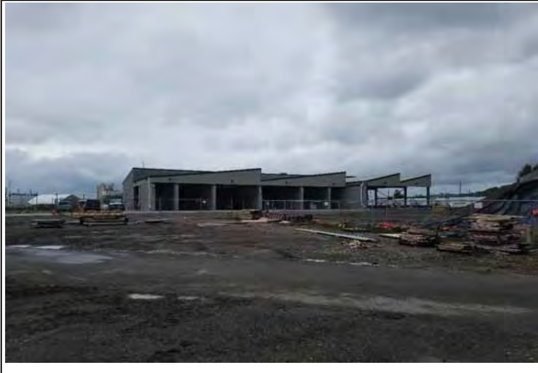
Photo 1: View of the eastern side of the new receiving building.
