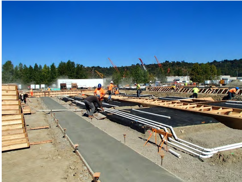
Photograph 1 Overview of project site and initial pipe layout
