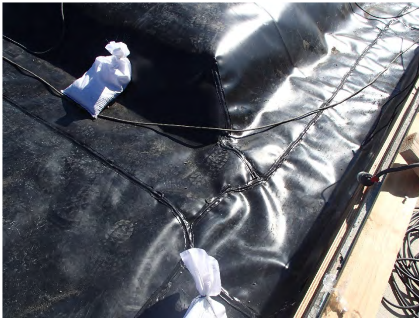
Photograph 14 Liner welds
