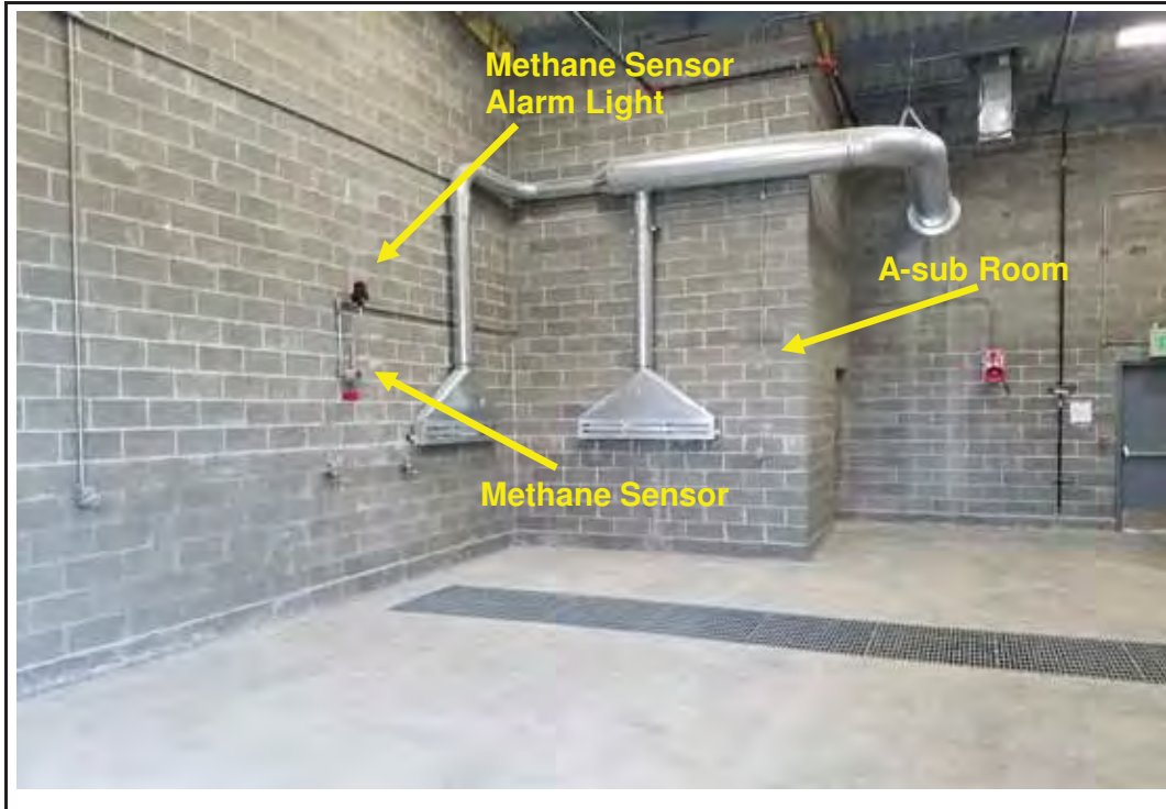
Photo 9: View of room "A" (from plans) looking to the west. Note the methane sensor and associated alarm light on the south wall (left side). Note A-sub room in corner.
