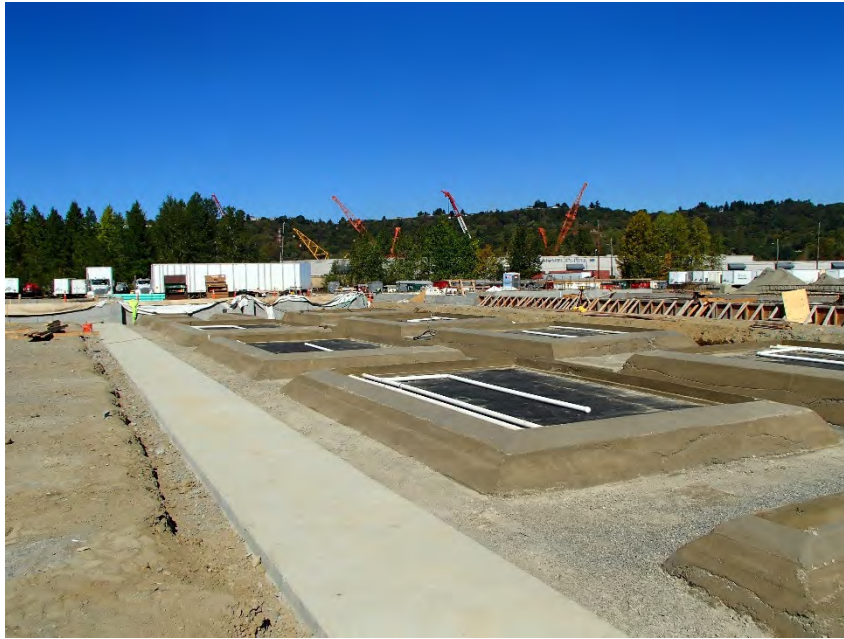
Photograph 7 Project overview after CDF cells have been poured
