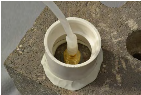
Figure 6. Water dam used for leak detection
