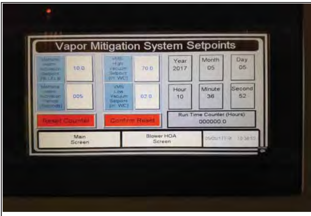
Photo 18: View of the VMS Control Panel - System Setpoints screen. Note the blue control set point buttons, red counter reset buttons, and date/time buttons.
