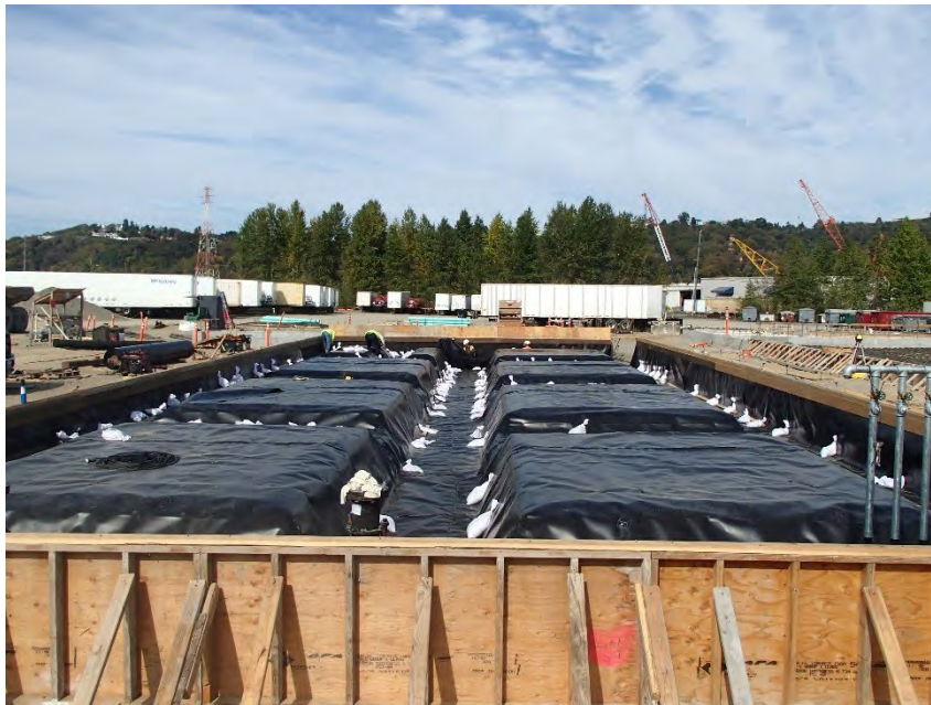
Photograph 17 Site overview of liner installation
