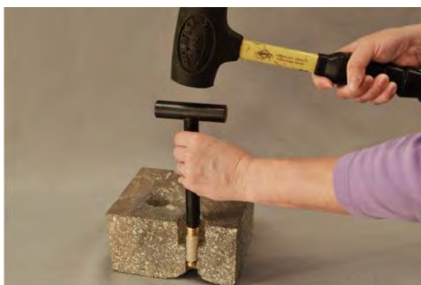
Figure 3. Flush-mount installation.
