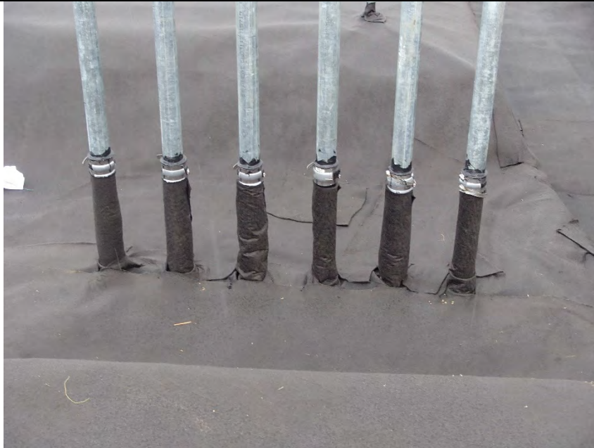
Photograph 21 Manifold top geofabric layer
