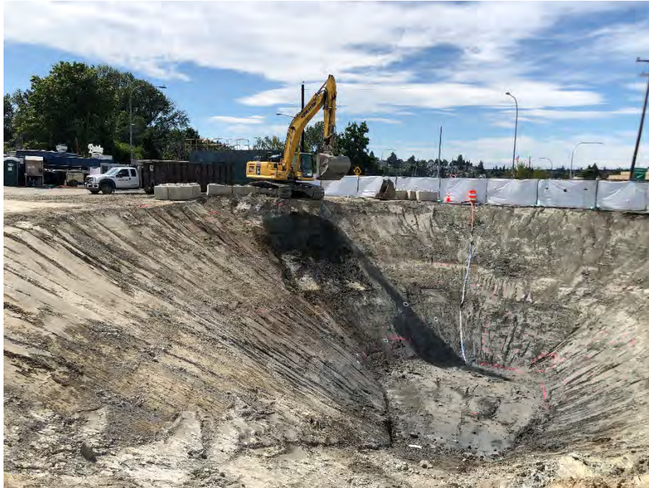
Photo 9. Looking west at Stage 1 excavation. August 6, 2021.
