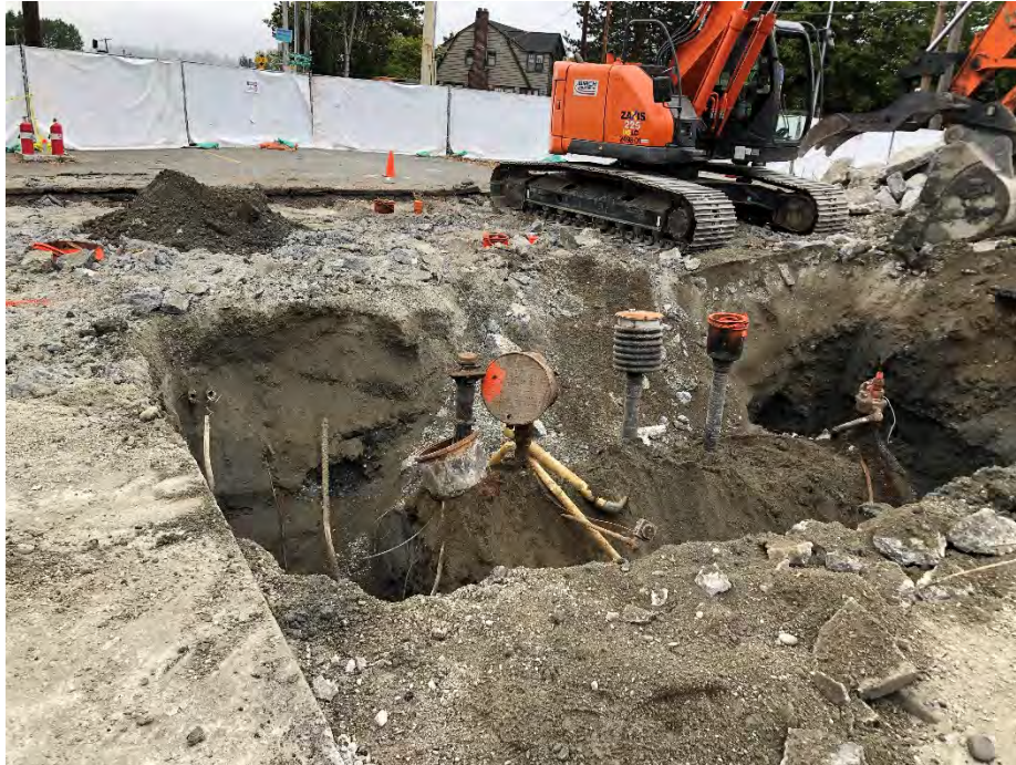
Photo 3. Excavating soil for removal of 5,000-gallon gasoline UST. July 20, 2021.
