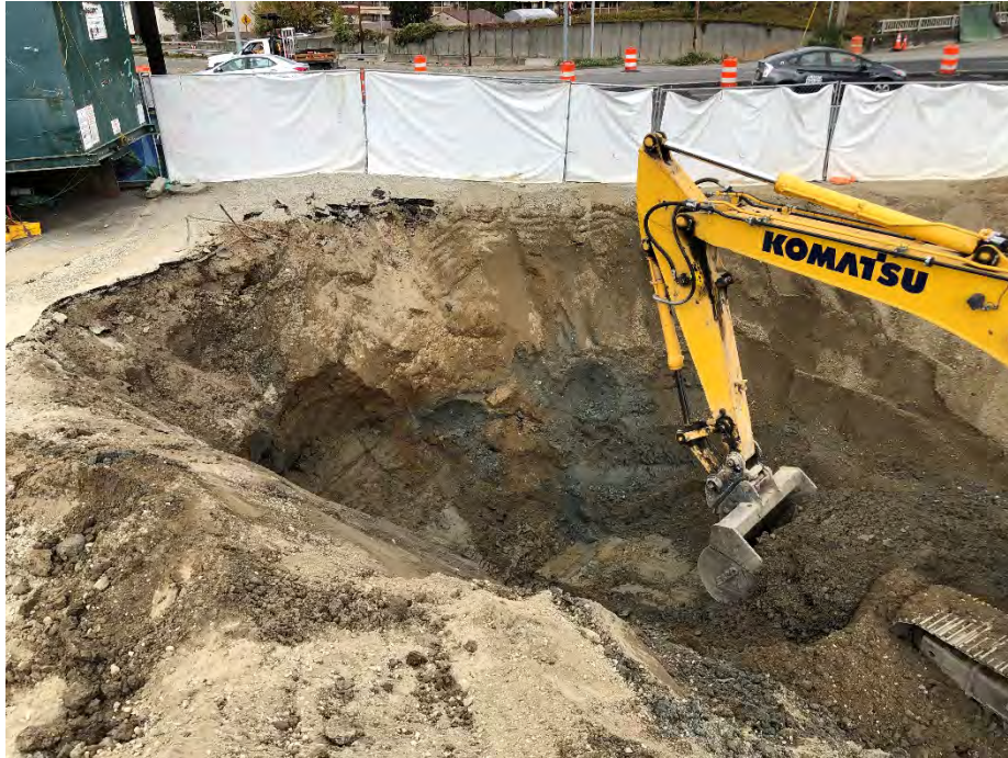
Photo 17. Over excavation west of sample location B2. September 13, 2021.
