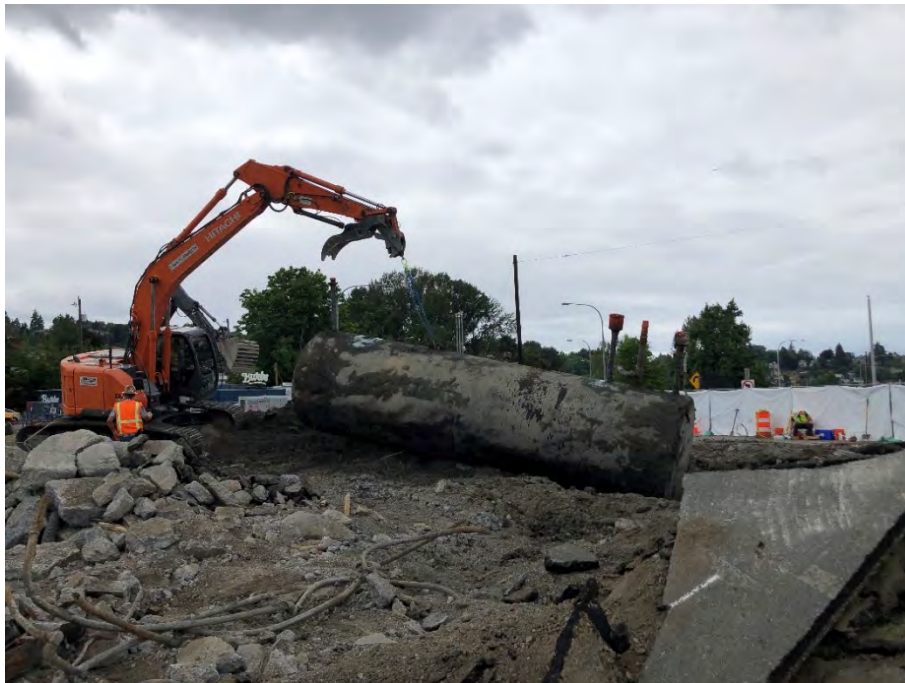
Photo 4. Removal of 10,000-gallon gasoline UST from ground. July 20, 2021.
