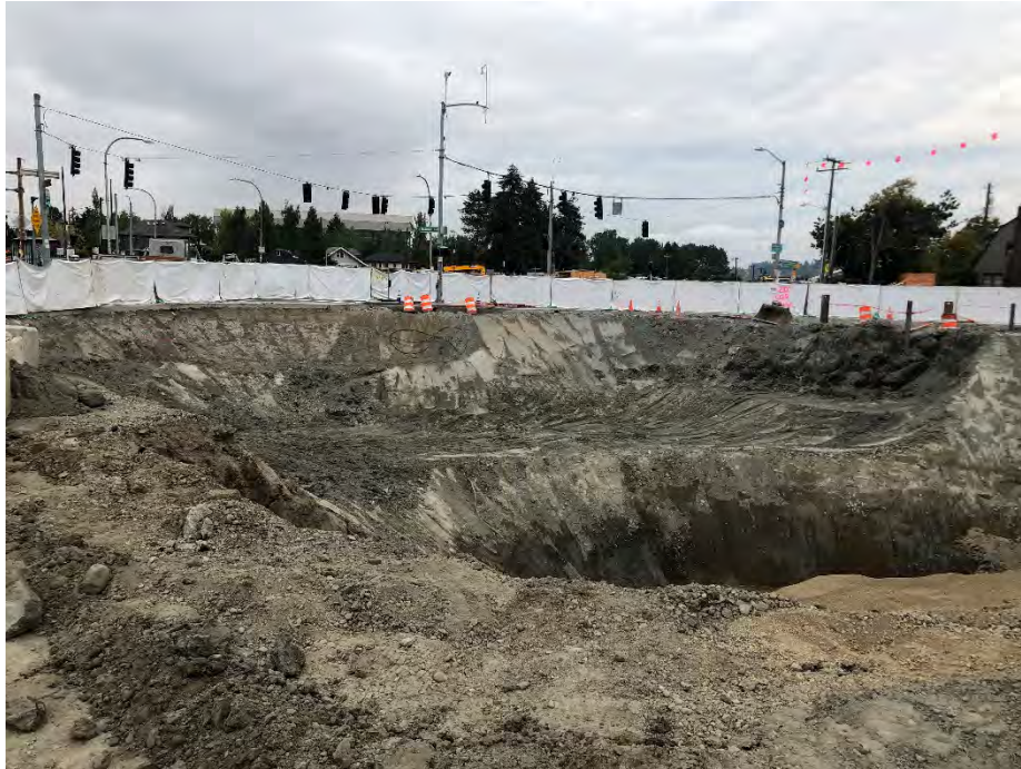
Photo 11. Begin Stage 2 excavation in right-of-way. August 16, 2021.
