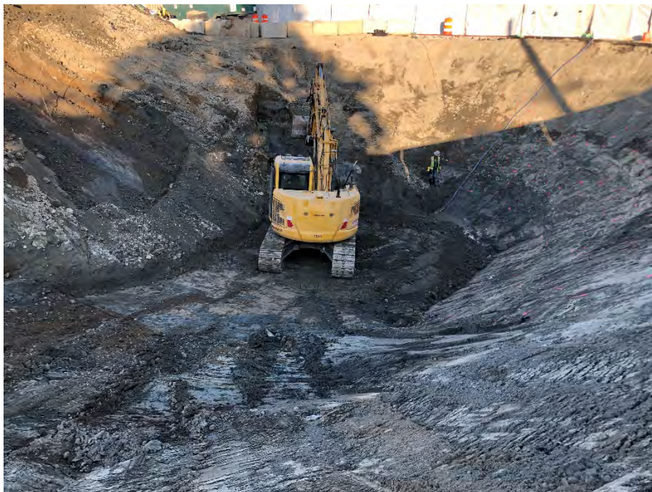
Photo 8. Looking west at Stage 1 excavation. 7/30/2021.
