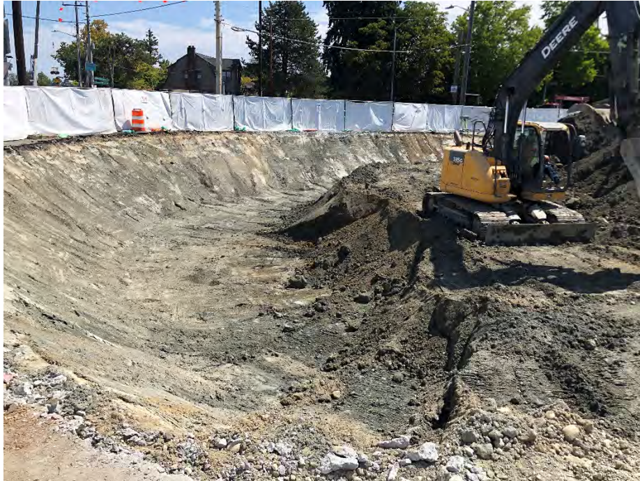
Photo 7. Begin cutting 1.5H:1V slope along northeastern boundary of Stage 1 excavation. July 27, 2021.
