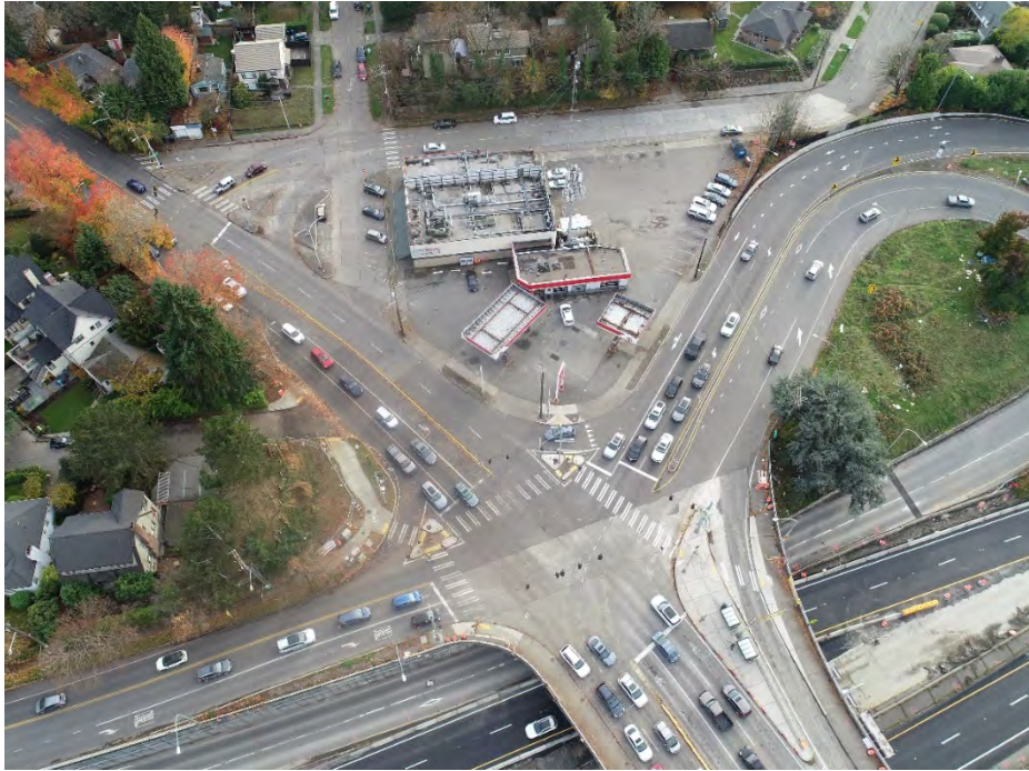
Photo 1. Former Montlake Market as seen prior to demolition of site structures, decommissioning of underground storage tanks (USTs) and remedial action by soil removal.
