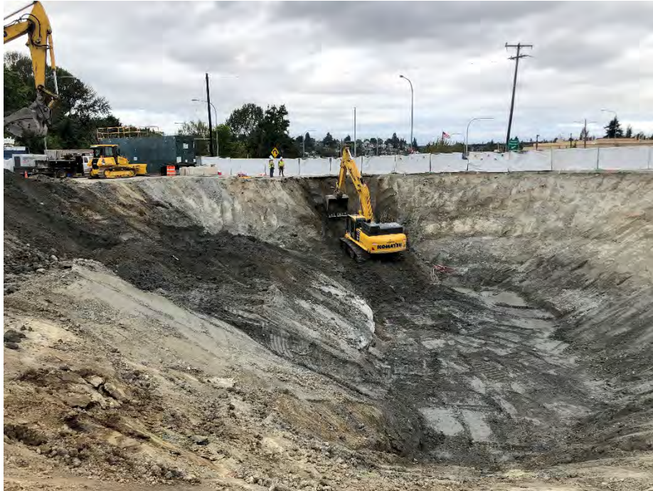
Photo 13. Begin over excavation of sample location D1 and D0.5. August 20, 2021.
