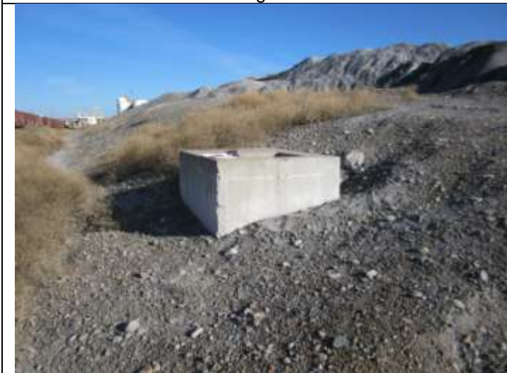
11 – Vault near dross stockpile
