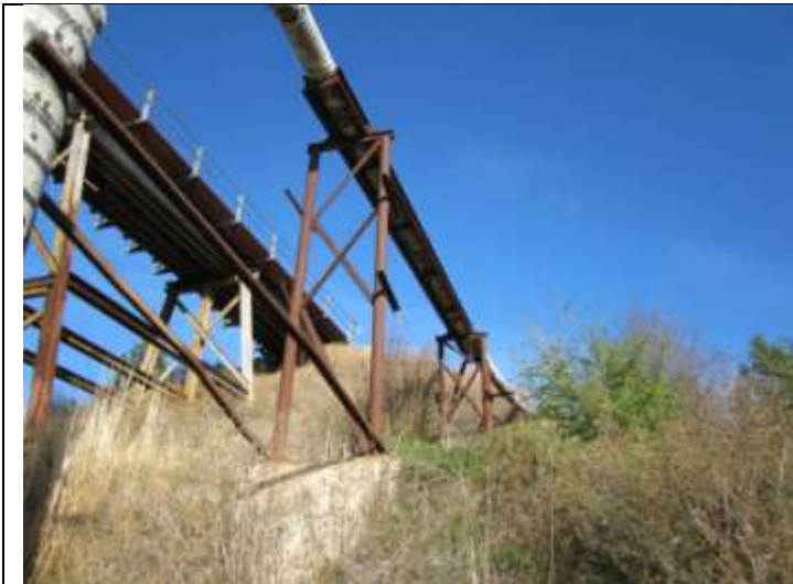
7 – Pipeline upslope of drop pipe
