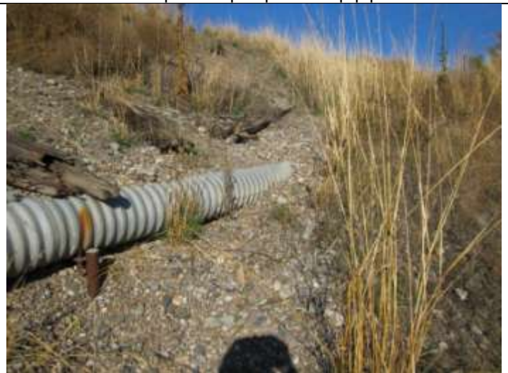
10 – Junction between above and underground pipeline
