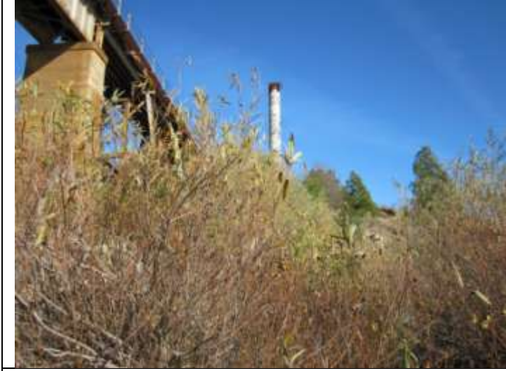
3 – View upslope from near shoreline showing drop pipe
