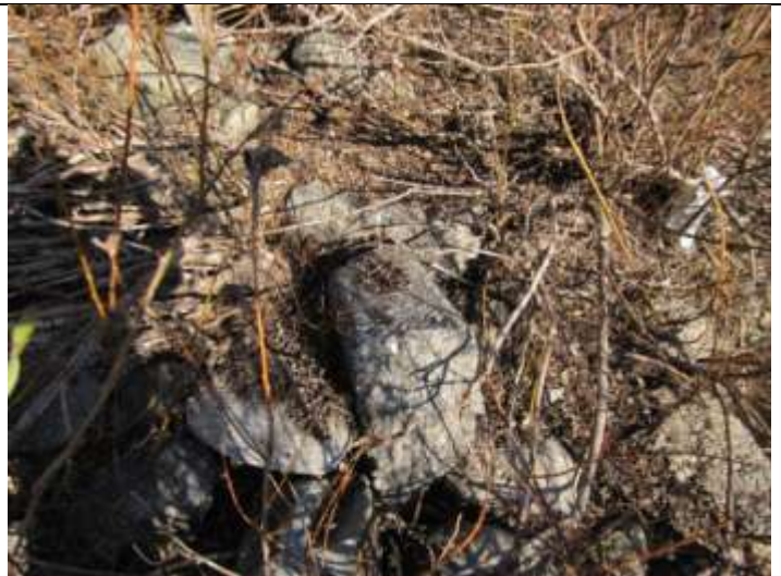
2 – Old concrete foundation near shoreline
