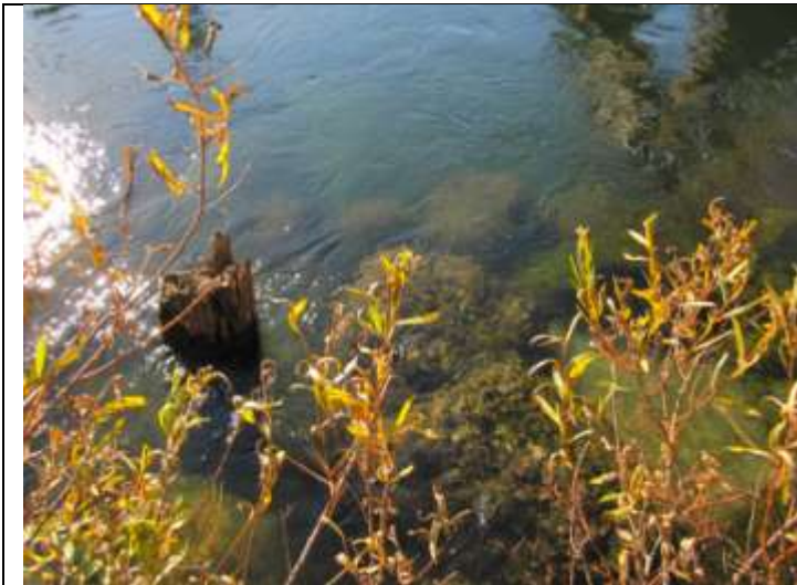
1 – Old concrete foundation underwater at shoreline
