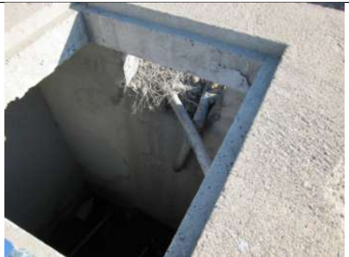
12 – Close-up of vault near dross stockpile
