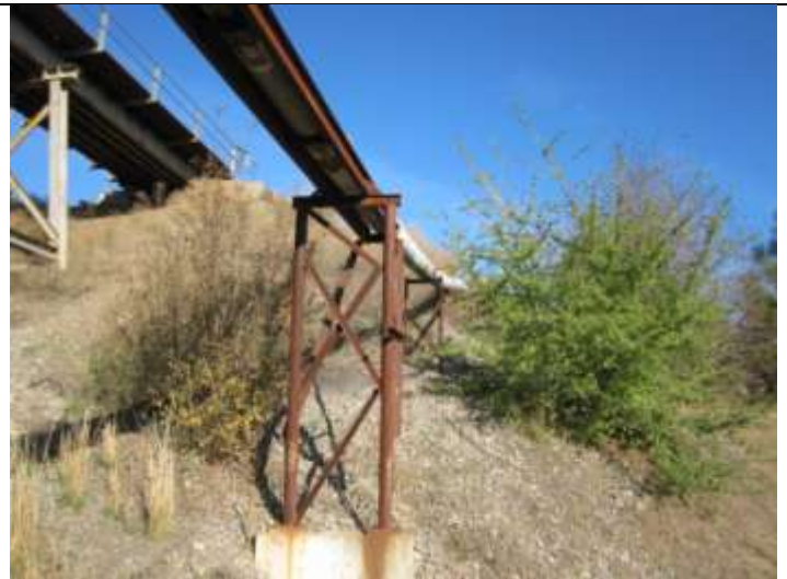
8 – Pipeline upslope of drop pipe
