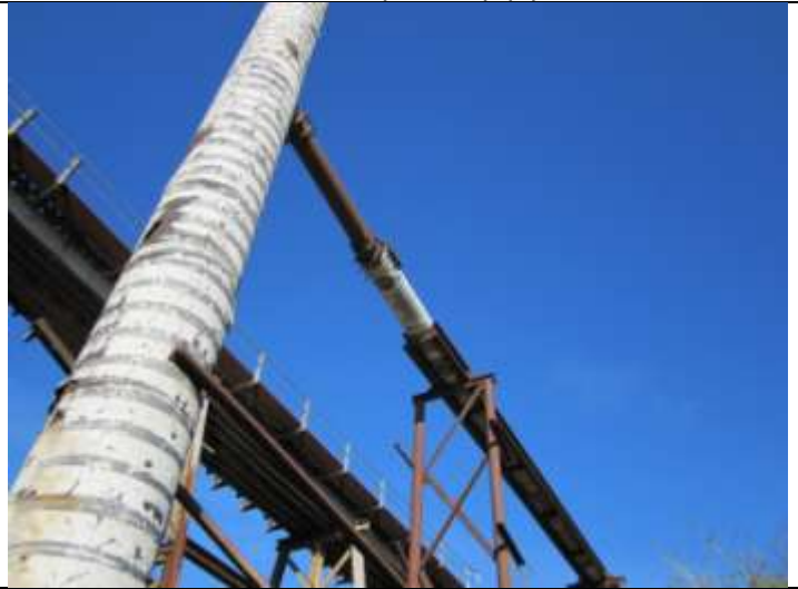
6 – Close-up – top of drop pipe and end of pipeline
