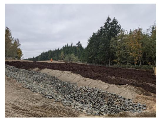
2020 – Stormwater Diversion (Photo shows Grass on the Capped Areas, and Rock Lined Ditches conveying water to Infiltration Ponds
