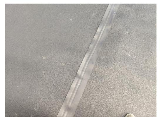
2020 – Cap Installation (Photo shows Geomembrane and Geocomposite Installed)
