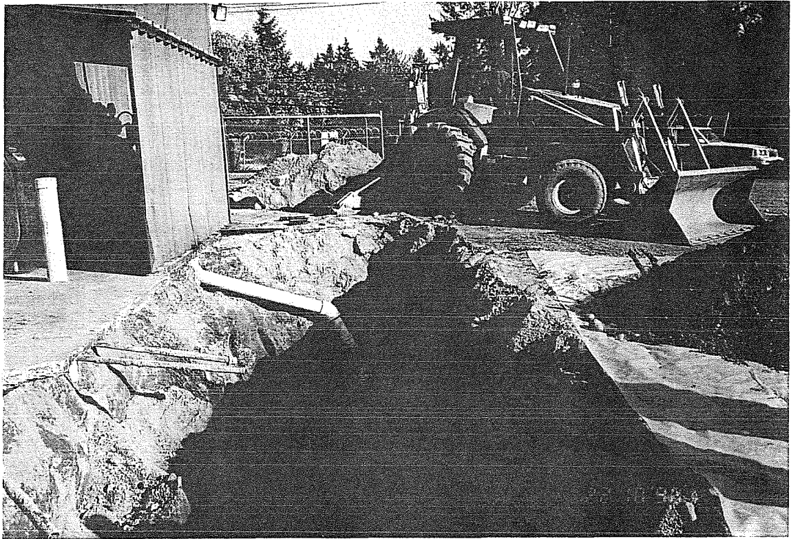
Plate 3. Excavation 2, after Removing (2)-2,000-g Gasoline USTs. O/W Discharge Pipe at NE End of Excavation. (View to NE).
