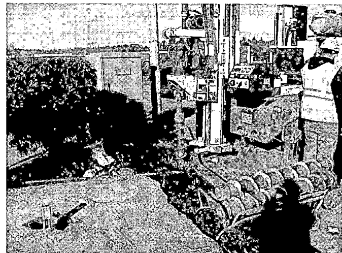
Well MW-3 in progress, over-drilling
